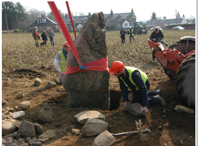
Fig. 12a - Packing stones into the socket
