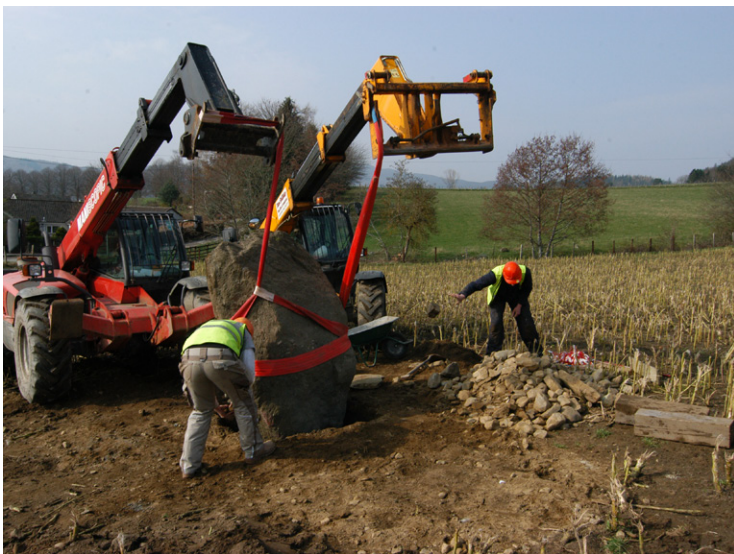
Fig. 12b - VPacking stones into the socket
