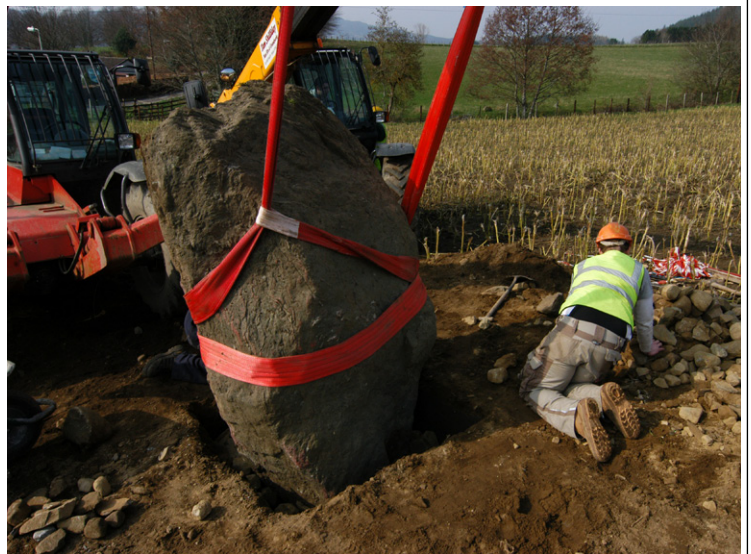
Fig. 12c - Packing stones into the socket
