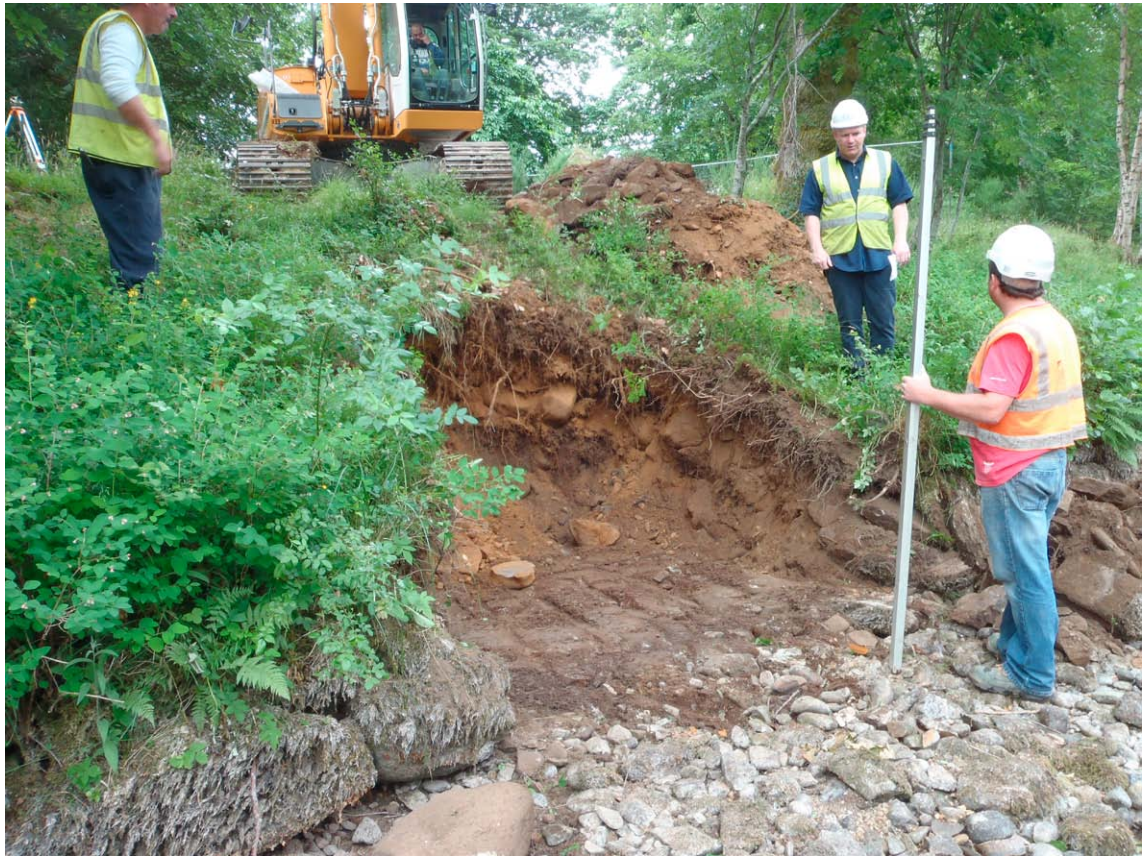
Fig. 2 - Trench excavated for the new concrete outflow, looking S
