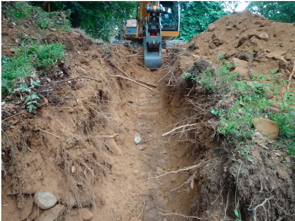
Fig. 3 - Trench excavated between the Outflow and the Manhole
