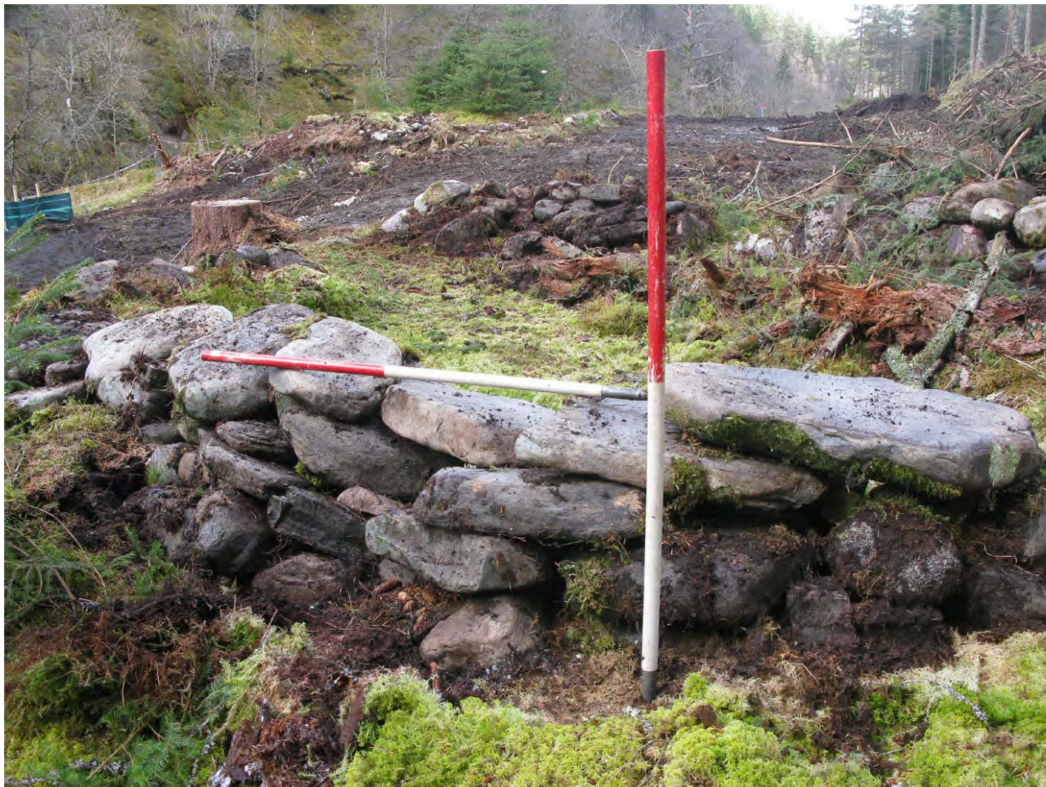
Fig. 8 External elevation of the south-east wall of Structure 4b
