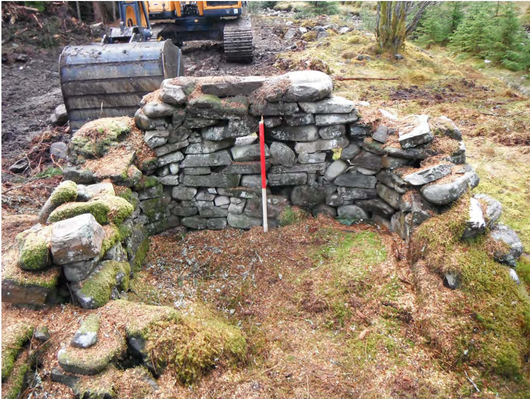
Fig. 7 Internal elevation of the south-east wall of Shieling 4a
