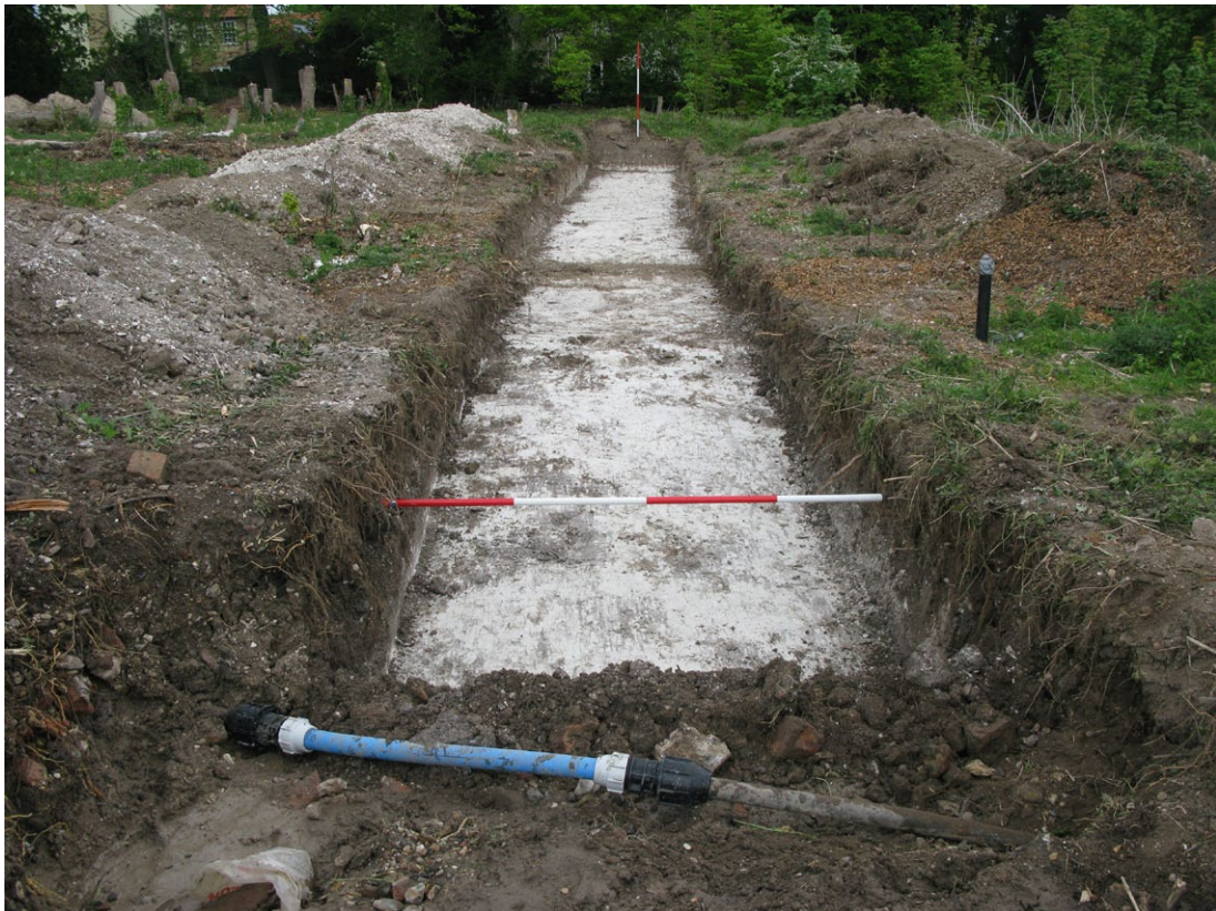
Fig. 5 - Trench 1 after excavation showing water pipe at south-west end.
