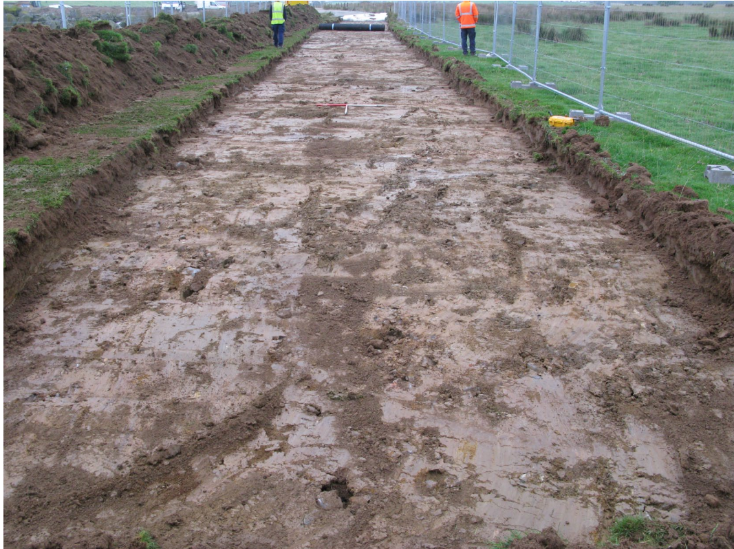
Fig. 11 - General shot of stripped access road between Towers WA11-12
