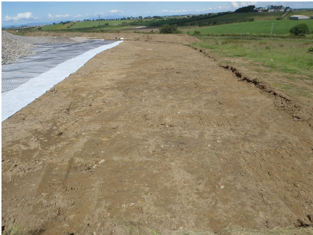
Fig. 10 - General shot of stripped area at Tower WA10
