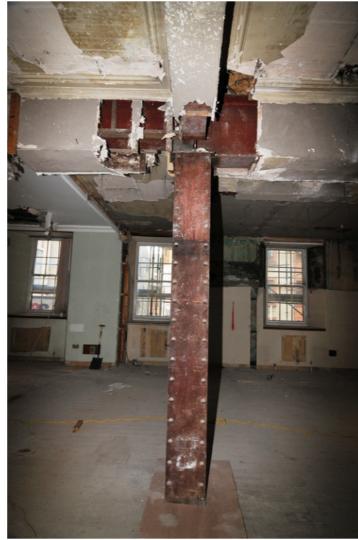
Fig. 18 Level 4, riveted steel stanchion and supporting steelwork beams above
