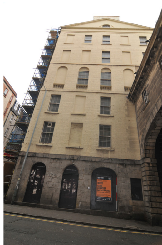
Fig. 27 Exterior south-facing elevation, general shot
