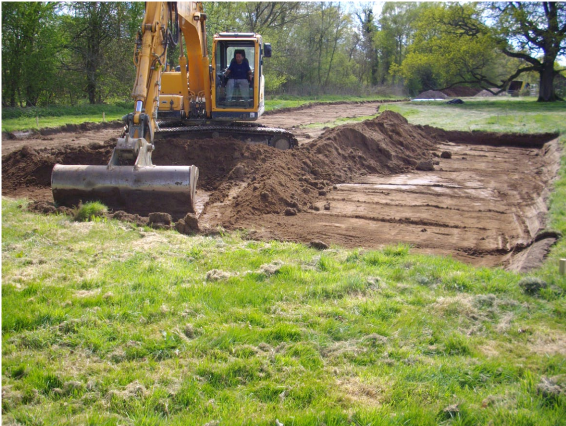
Fig. 6 - Excavation to formation level showing quarrying
