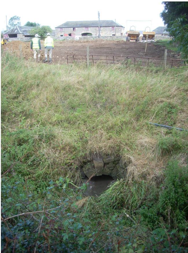
Fig. 3 - The outflow from the culvert
