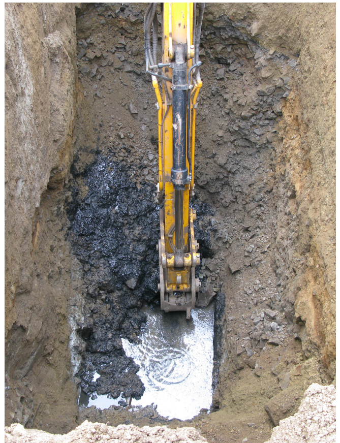
Fig. 4 - Working shot showing the removal of the culvert structure
