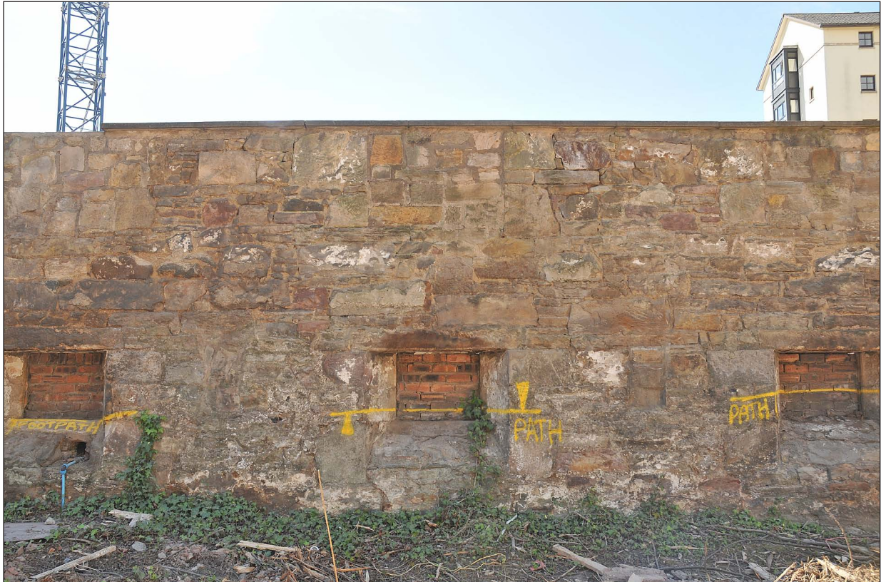
Plate 3 - General view of the blocked vents (Feature 8) on the north-facing elevation with the level of the footpath on the opposite side marked in yellow paint.
