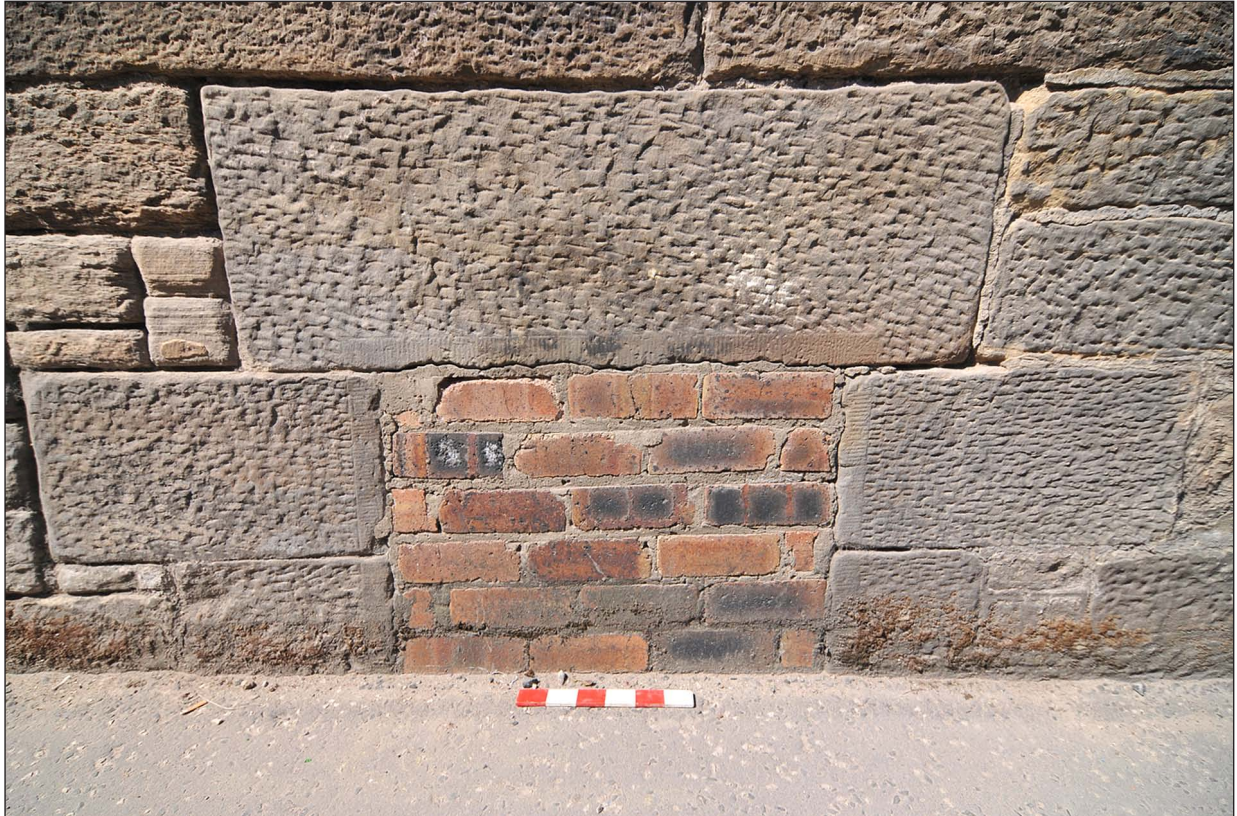
Plate 7 - General view of one of the blocked vents (Feature 8) at ground level on the south-facing elevation.
