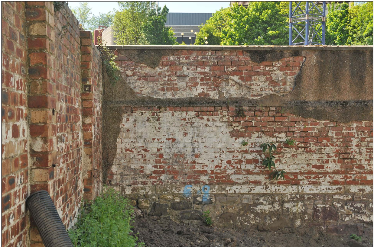
Plate 2 - Brick-built walls (2-3) over rubble wall (1), eastern terminus of the north-facing elevation.
