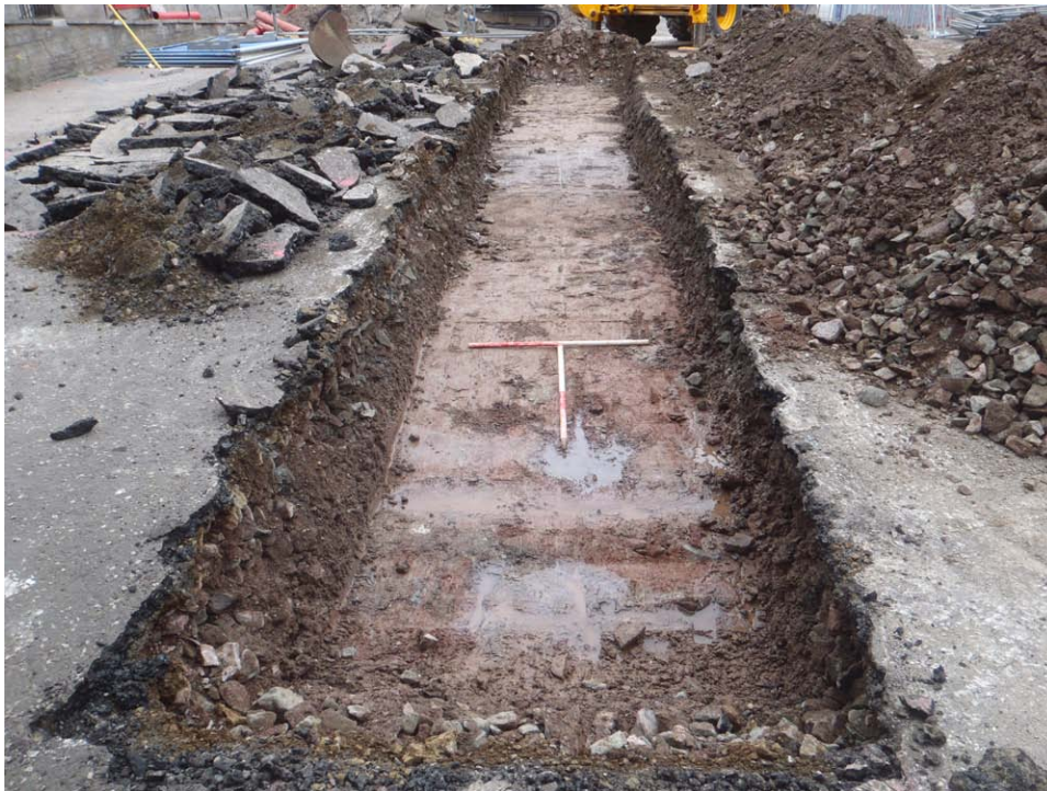
Fig.3 - Trench 2 from the north-west
