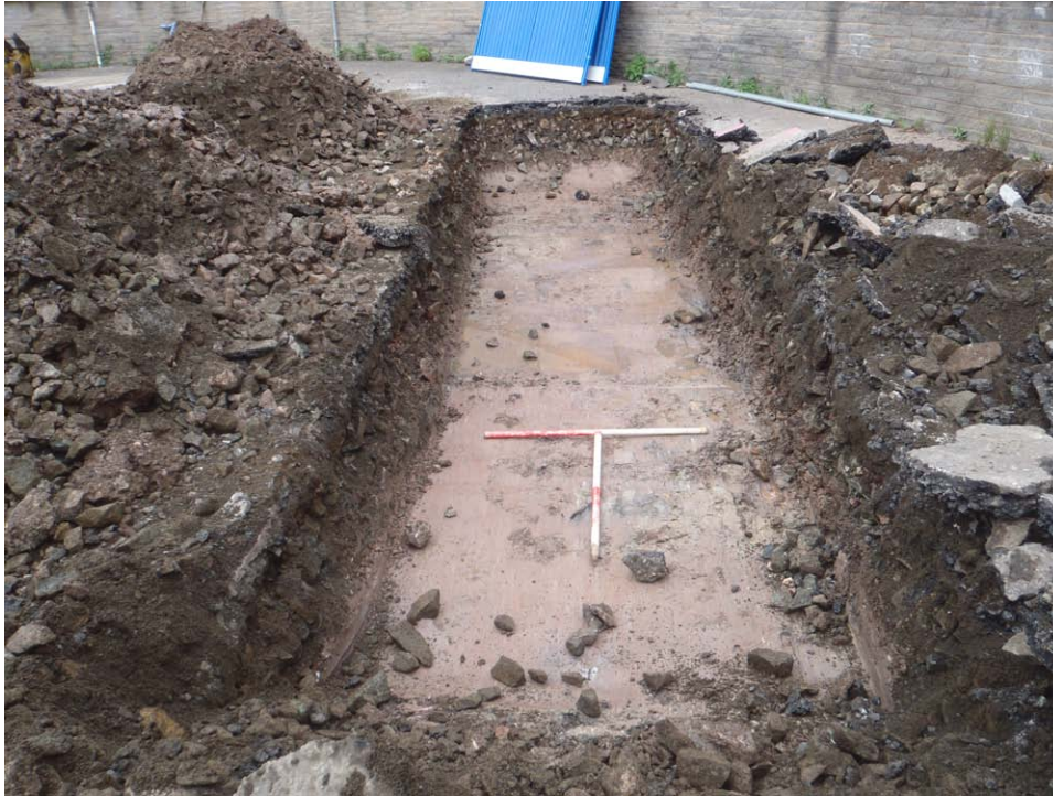
Fig.4 - Trench 3 from the south-east
