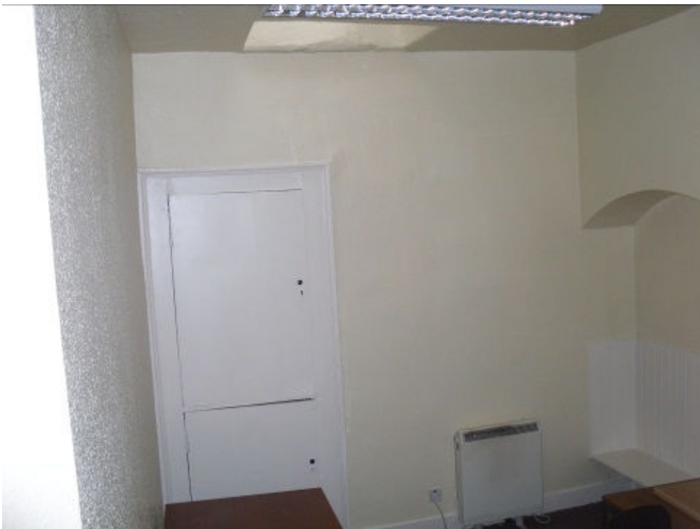
View of S.08 facing east wall, featuring arch recess with bench on right and aperture for skylight on ceiling.
