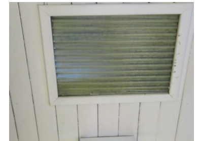
Roof hatch leading to neighbouring building
