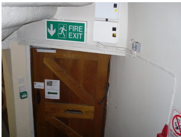
Main public entrance to SHBT, with underside of turnpike stair in left hand corner.
