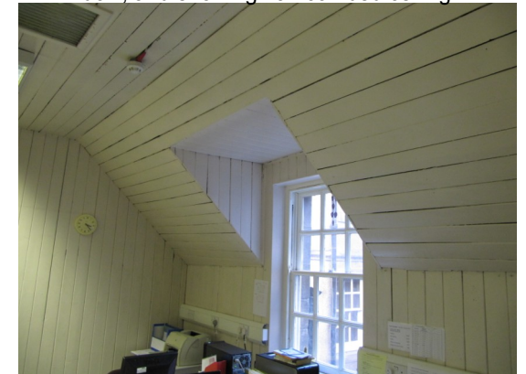
View of F.04 facing south with dormer window, and showing half combed ceiling.
