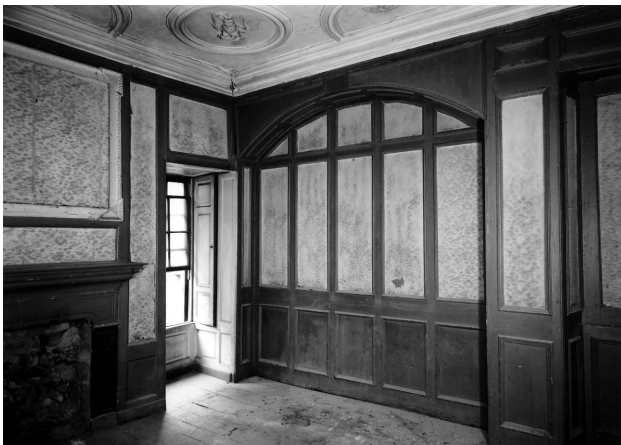
View of S.03, facing north-west, before renovation started 1964. ©RCAHMS
