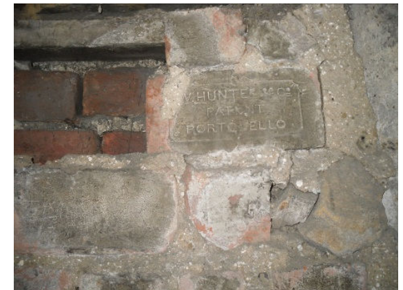
Engraved brick on north wall (right hand side of entrance).
