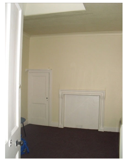
View of blocked c. 17th century fireplace and small press.
