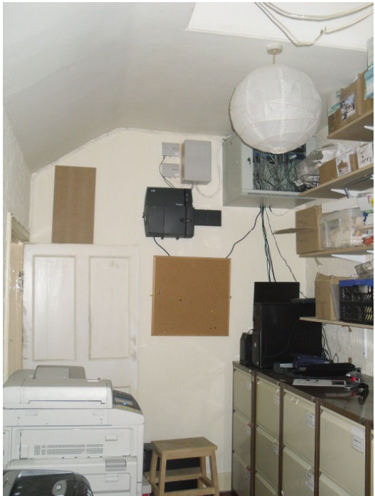
View of S.18 from entrance door, with sloping ceiling on left, and aperture for skylight on right.
