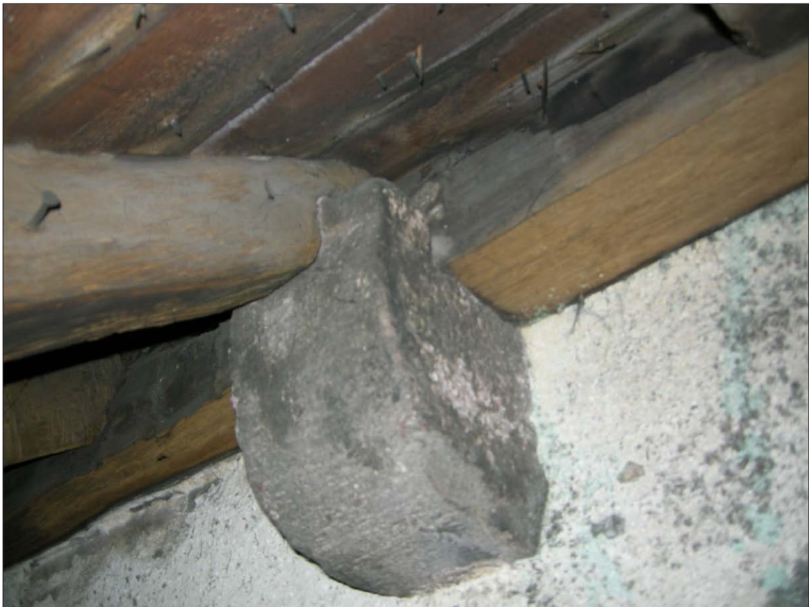
Plate 6 - South Block, north side, detail of the corbel and overlapping timber work
