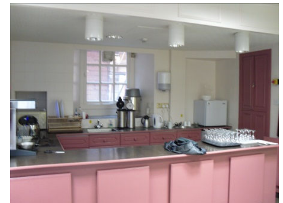
Kitchen galley of G.04 with suspended ceiling.
