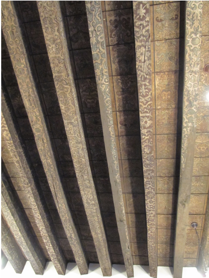
General view of the beam ceiling of F.02.
