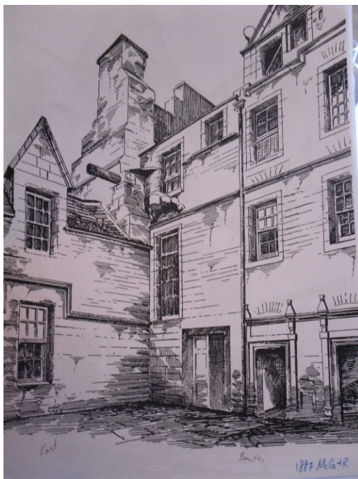
Image of courtyard identifying possibility of formerly longer window in F.12 (seen in the corner where the south and east wings meet). From MacGibbon and Ross sketches (1887).
