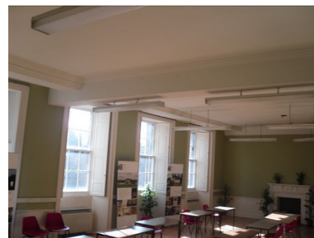
View of south wall facing Victoria Street and Terrace, with evidence of former walls on ceiling.
