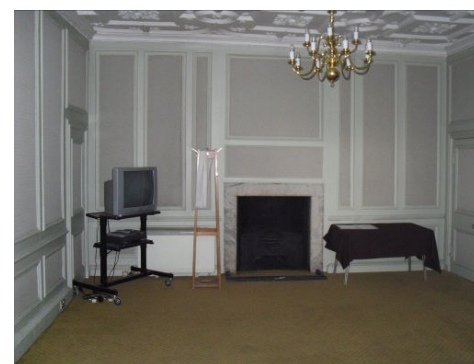
F.10 facing north, featuring 18th century panelling on walls.
