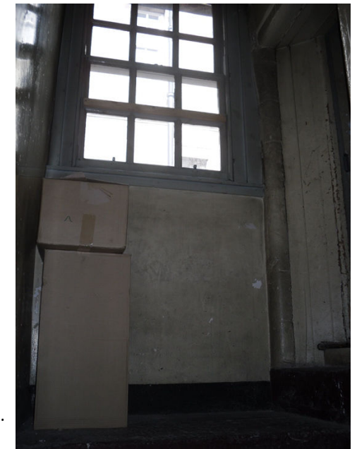
View of F.11 from stair 02, facing courtyard.
