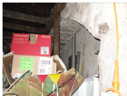
Stone arch on north wall with timber beams above.
