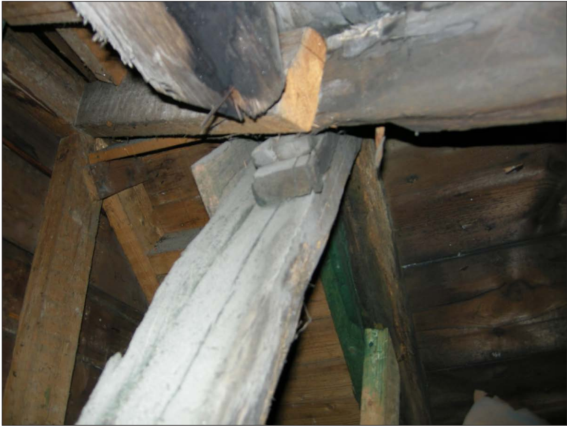
Plate 7 - South Block, north side, complicated arrangement of timber repair work
