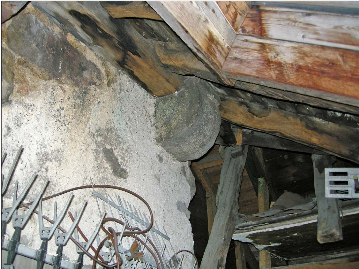
Plate 5 - South Block, north side, one of four corbels supporting the roof structure
