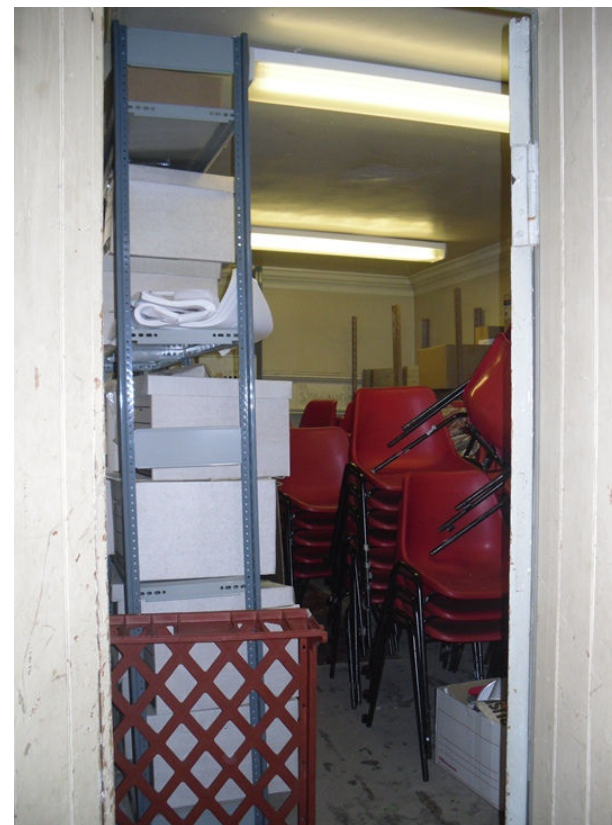
View of F.12 from F.11, facing east.
