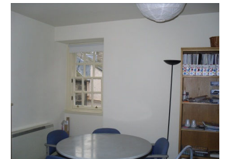
View of window facing west, with replaced south wall on left.
