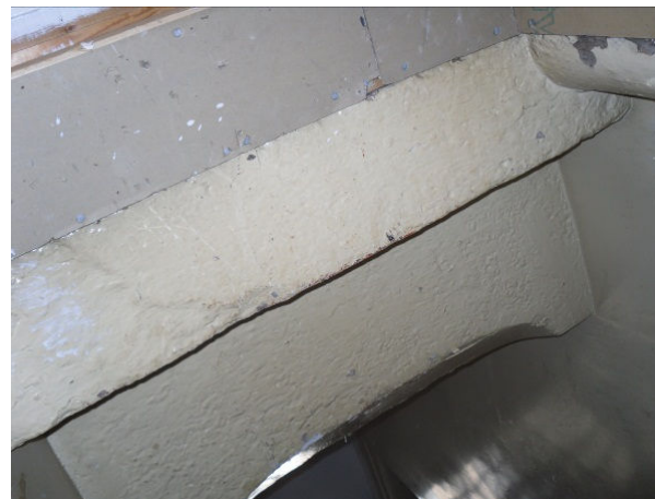
View from under the door frame looking up. Brown edge in left hand corner indicates timber section of door frame, with strong cardboard immediately below this (grey) and the stone thereafter (cream).
