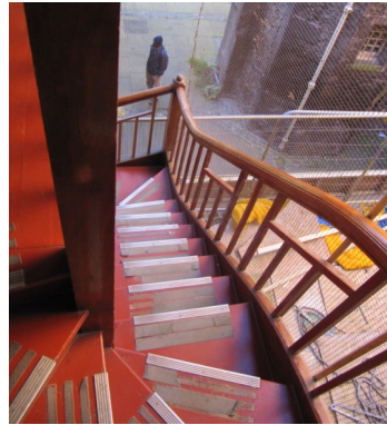
View of Stair O4 from the second floor.
