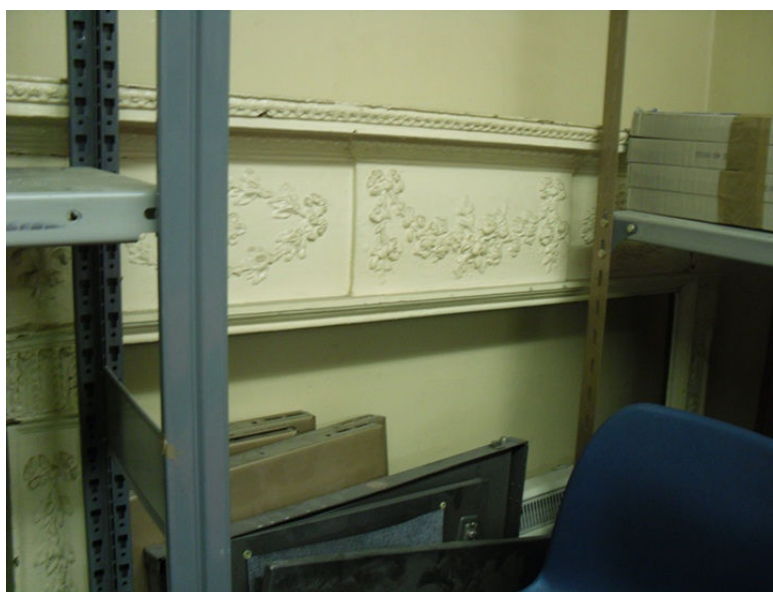
View of 18th century chimneypiece/fire surround, formerly on east wall of G.08.
