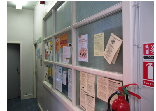
View of F.01, facing east, with glass pane wall to F.02.
