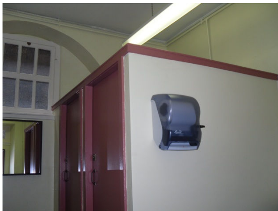
View of stone arch on west wall and W.C.'s.
