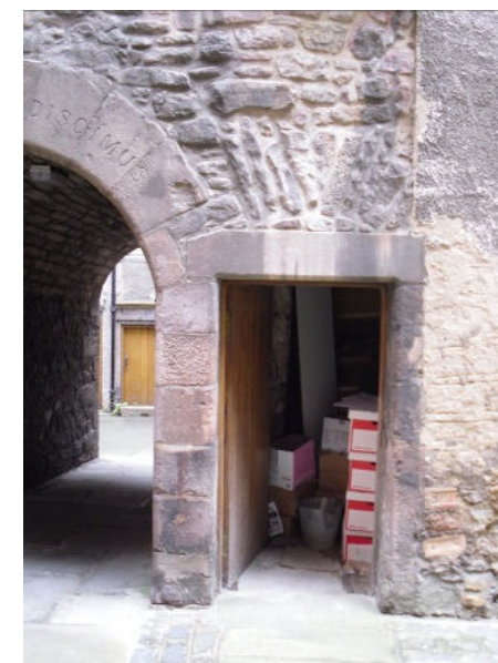
Entrance to G.01 from outer court with pend to left.
