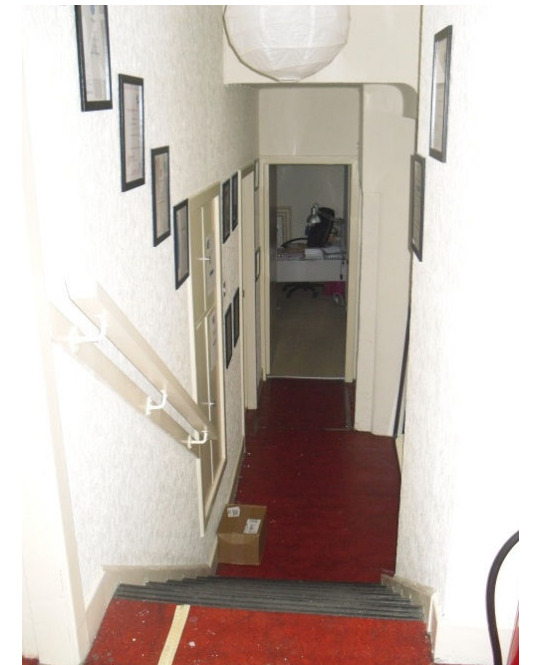
View of S.12 from top of stair 07, featuring remaining section of earlier wall on ceiling (immediately behind the light in above photo).
