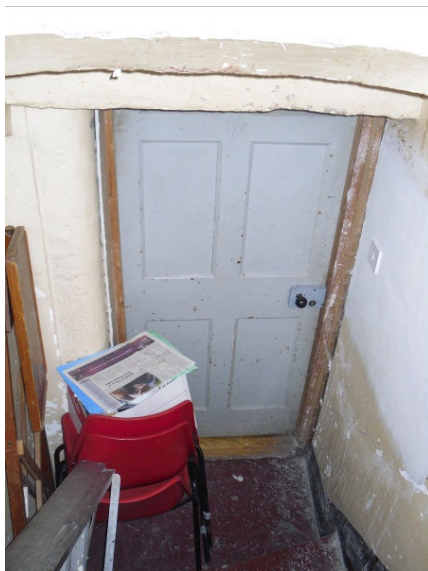
View of G.09 from stair 02.
