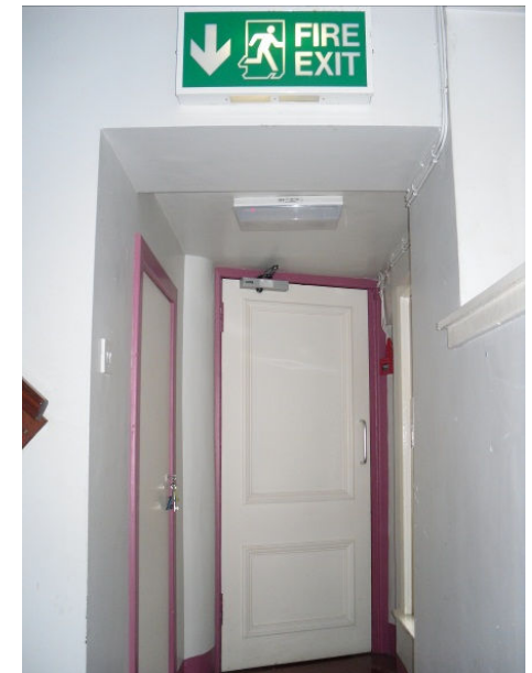
View of S.07, facing door (i).
