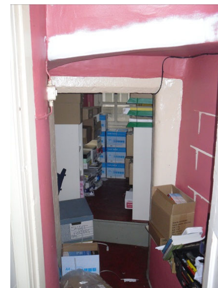
View looking down into S.19 from S.18, with section of former wall highlighted in white paint at top of photo.
