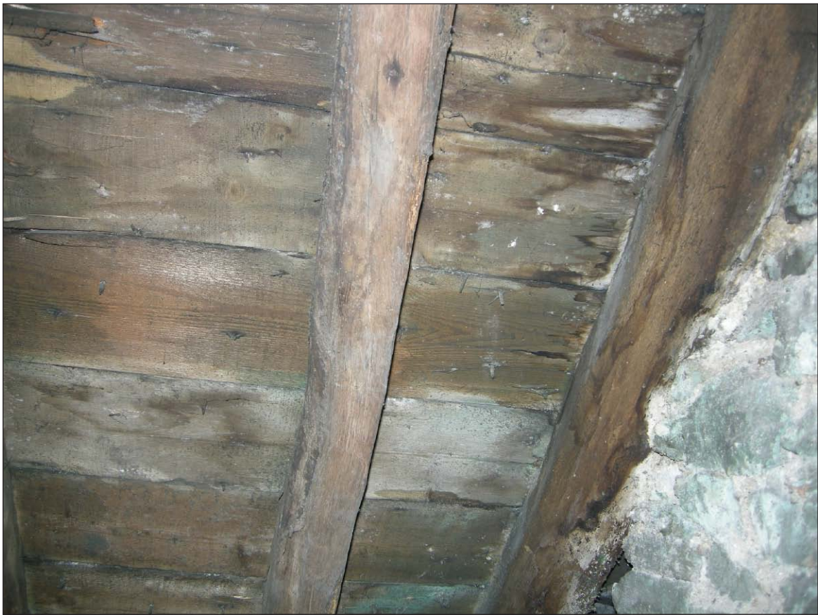
Plate 8 - South Block, north side, pine sarking boards nailed to oak rafters
