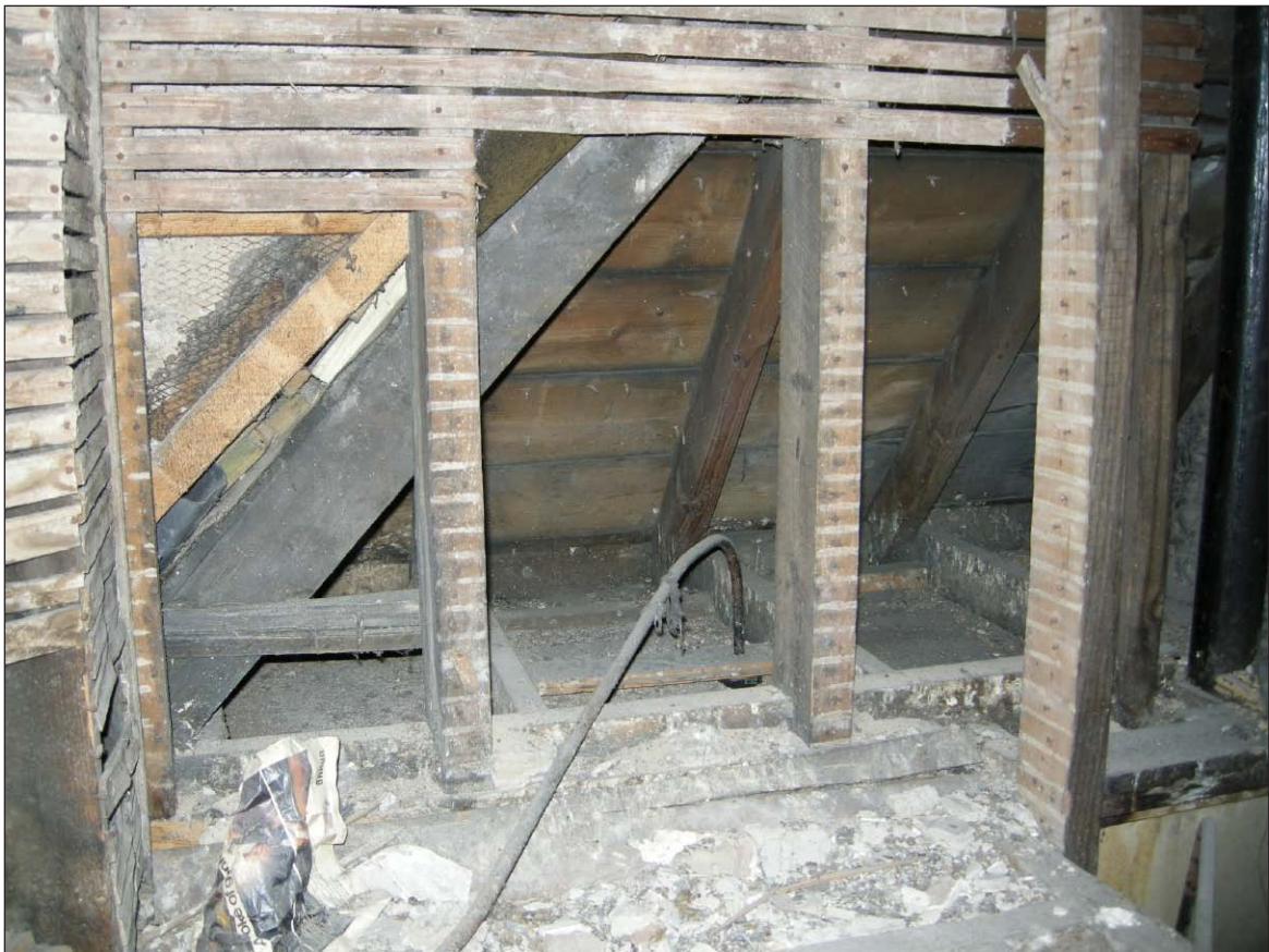
Plate 10 - North Block, north-east end, stud partition work relating to earlier (19th century?) occupation of the attic space
