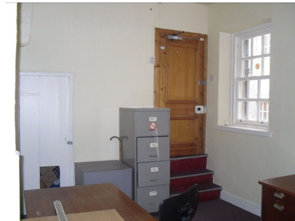
Protruding section of wall in top left corner and desks and filing cabinets from previous occupiers.
