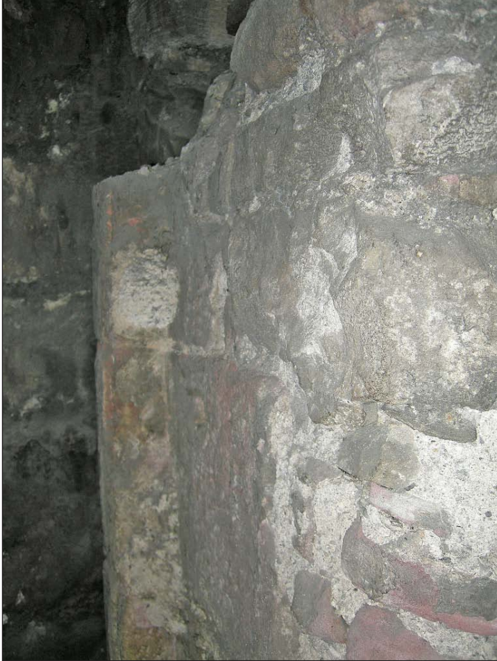
Plate 11 - North Block, north-east end, the remains of window rybats
