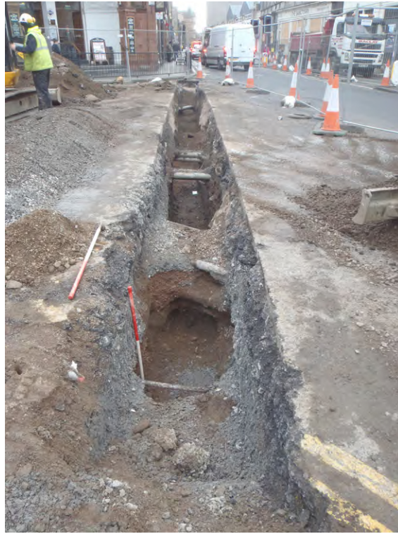
Fig. 9 Trench 1 showing the numerous services crossing the trench
