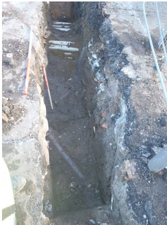
Fig. 10 Trench 2a showing the numerous services crossing the trench
