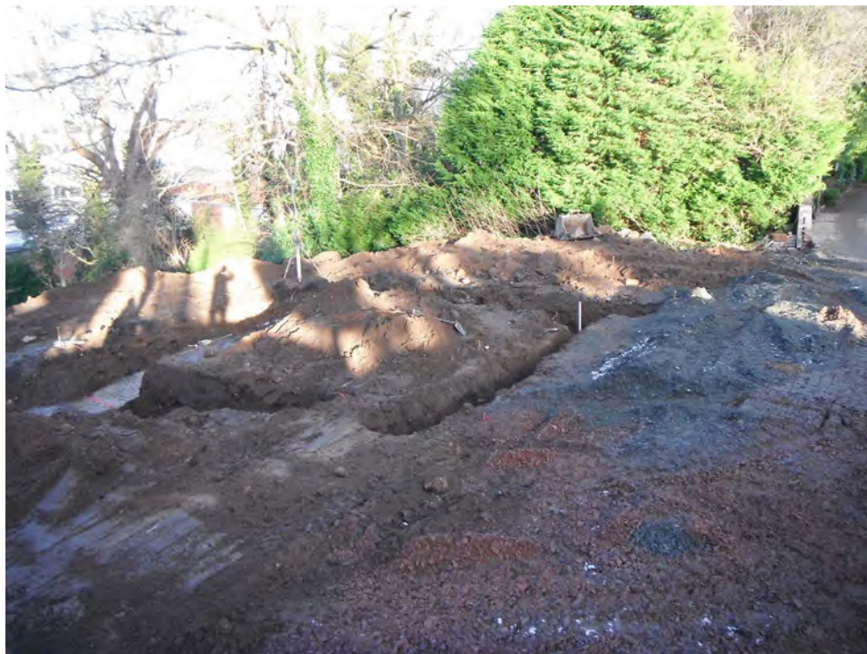
Fig. 5 - Site following foundation excavation
