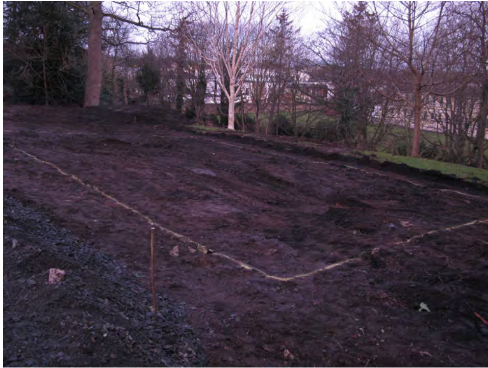
Fig. 2 - Site prior to foundation excavation
