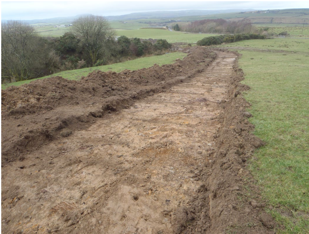
Fig. 4 - General view of wayleave, eastern end, from S
