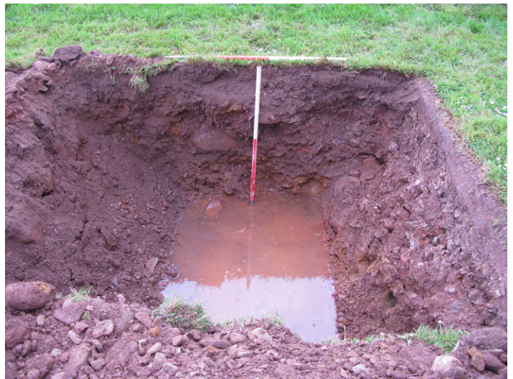
Fig. 5 - Photograph of Trial Pit 4
