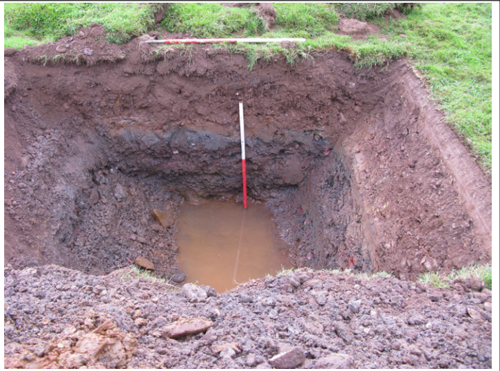
Fig. 7 - Photograph of Trial Pit 6
