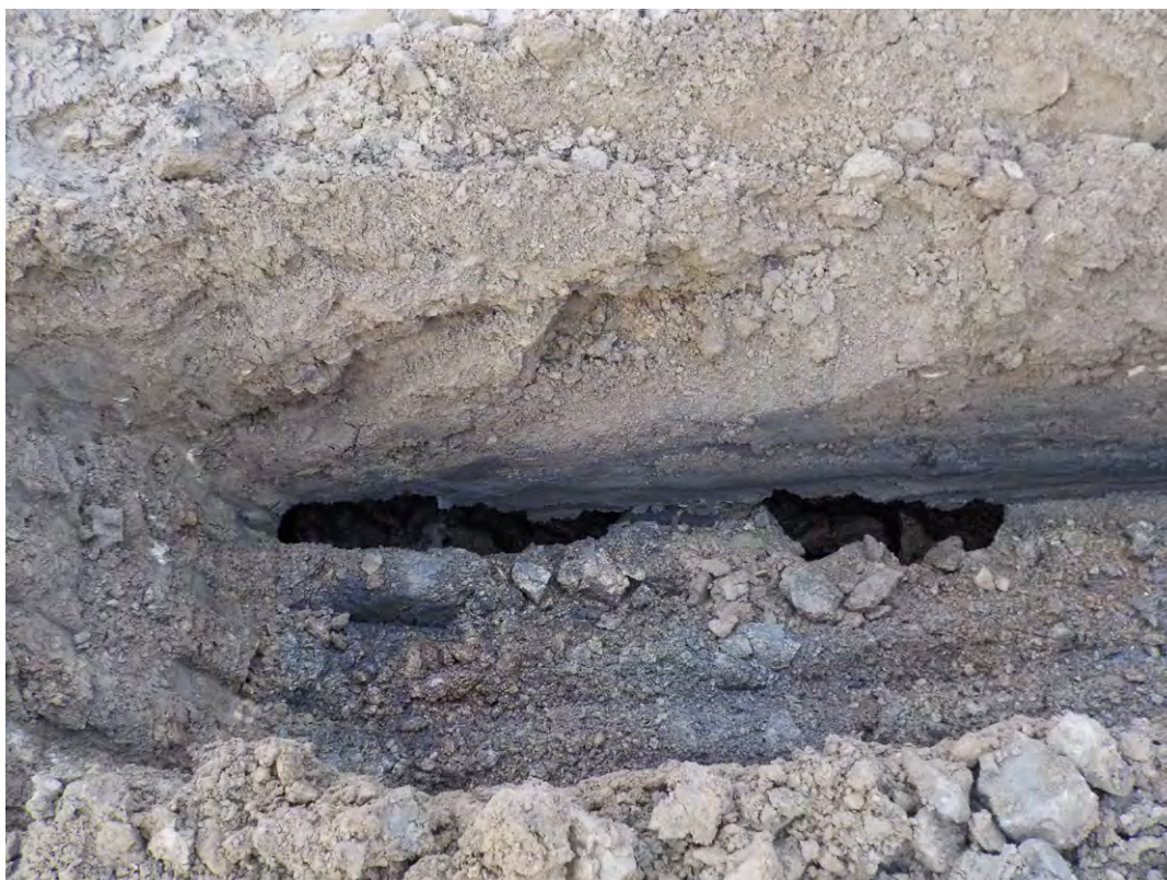
Fig. 4 East facing section of collapsed adit
