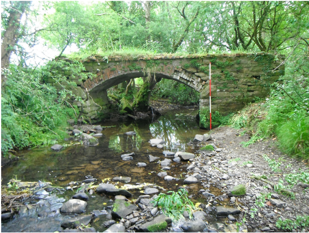
Fig. 15 - Site 11. North-east-facing elevation
