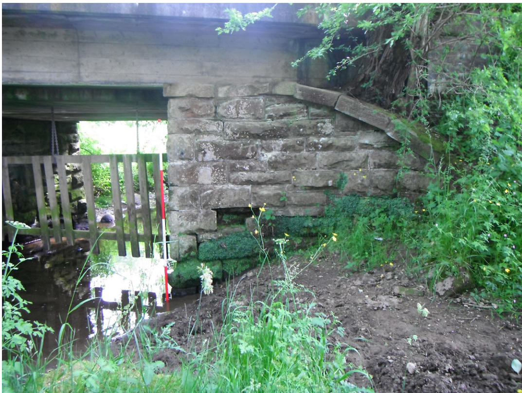
Fig. 12 - Site 8. North-facing elevation, western abutment
