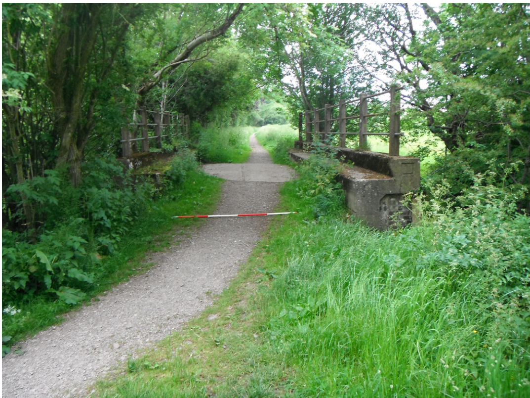
Fig. 14 - Site 8. View of the bridge deck from the east
