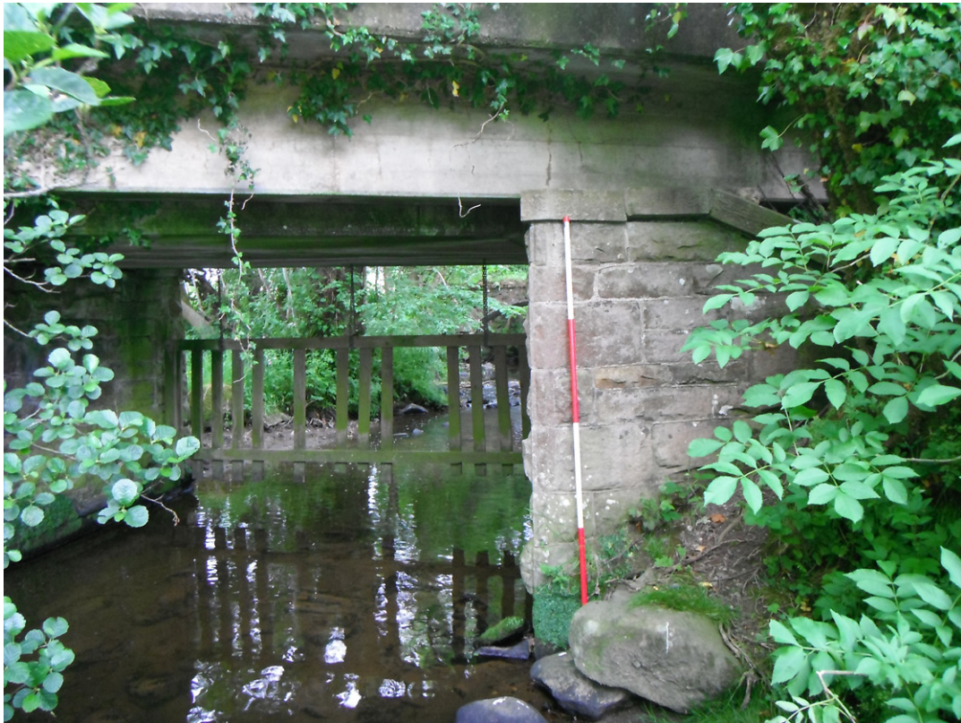
Fig. 13 - Site 8. South-facing elevation, eastern abutment
