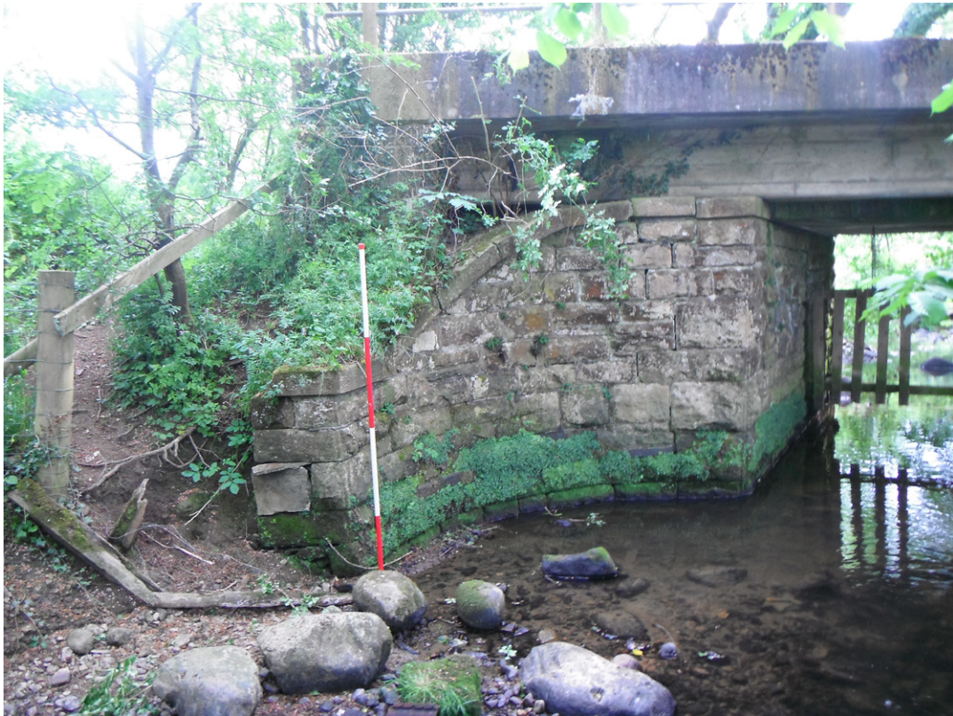
Fig. 11 - Site 8. North-facing elevation, eastern abutment
