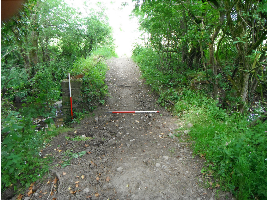
Fig. 17 - Site 11. View of the bridge deck from the south-east
