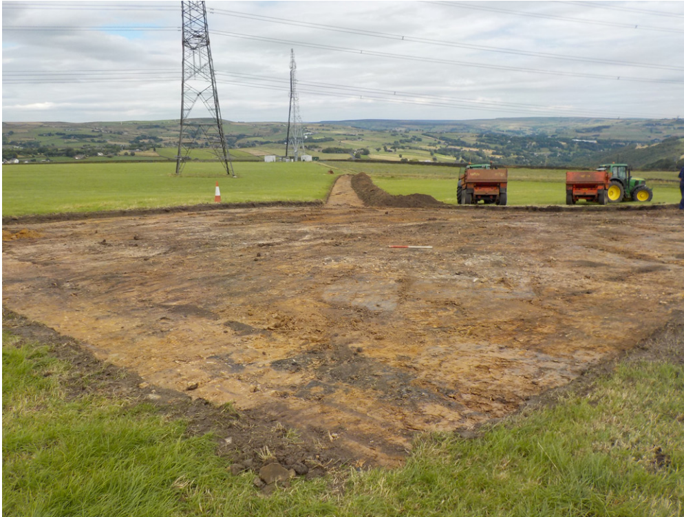
Fig. 2 - The turbine base stripped
