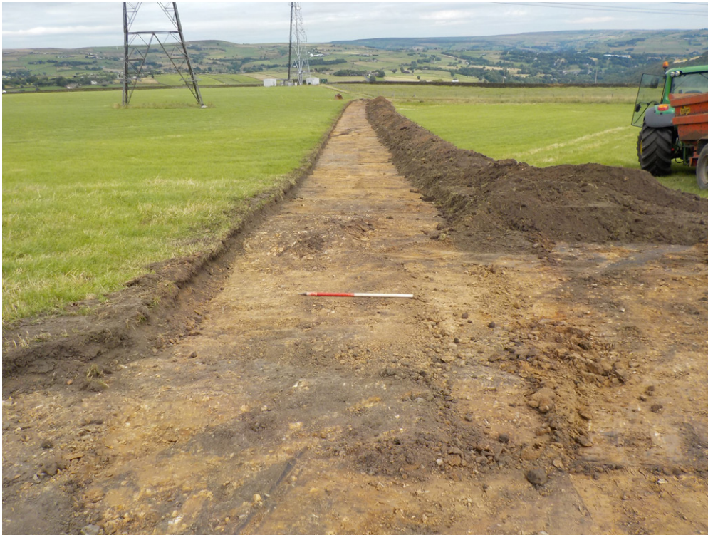
Fig. 3 - The access road stripped
