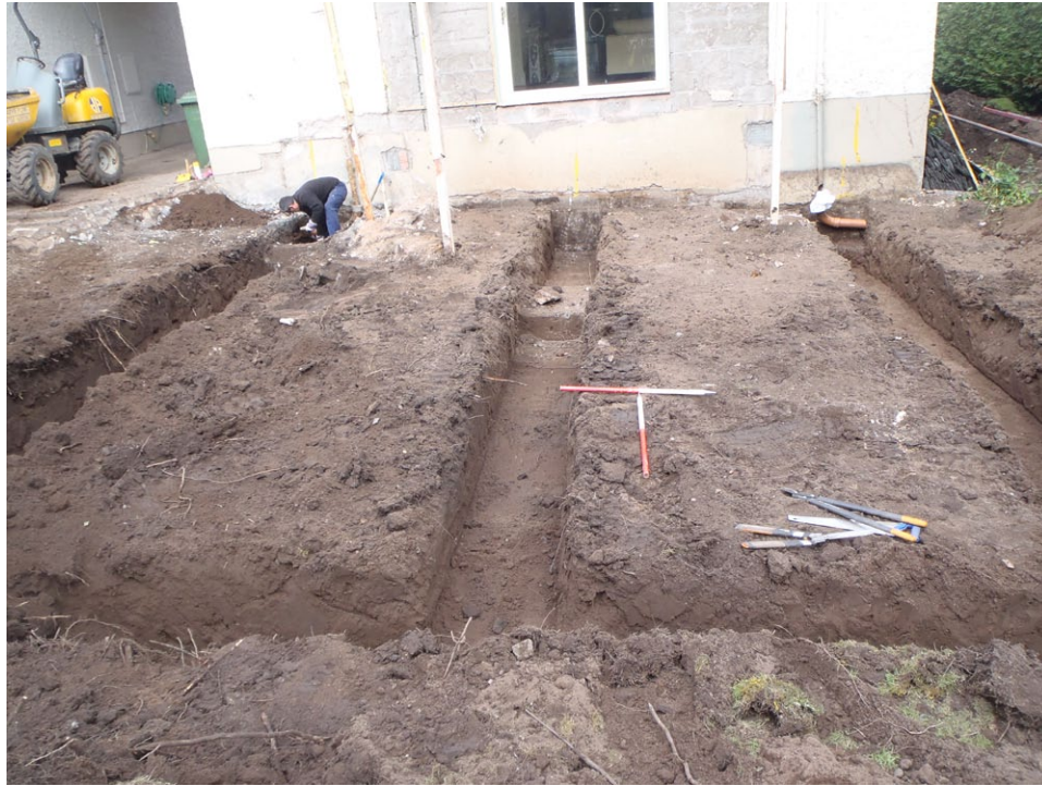
Fig. 2 - Layout of foundation trenches post-excavation
