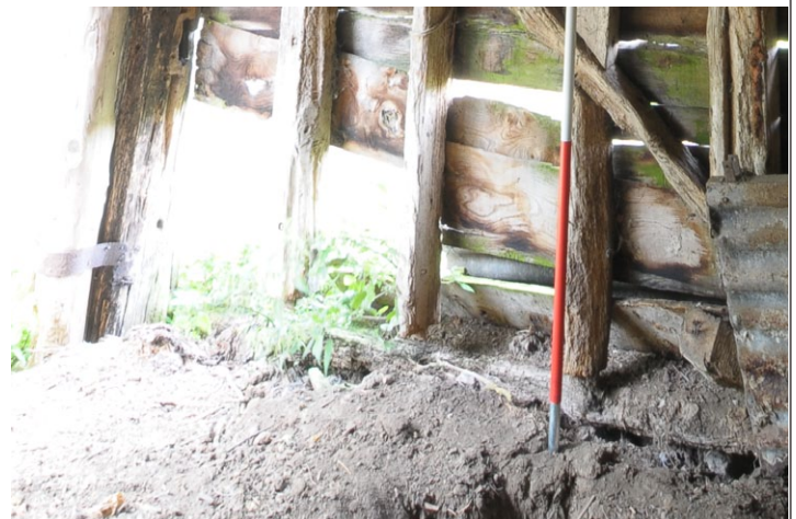
Fig. 23 - Shot of sill beam of west gable
