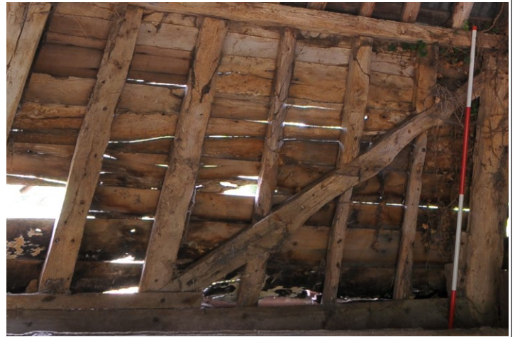
Fig. 19 - Studs, east end of rear wall
