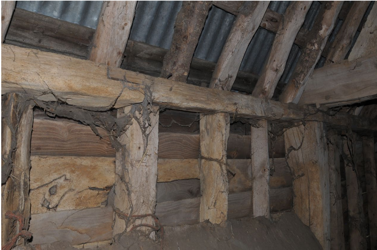
Fig. 16 - Shot of wall plate of rear wall
