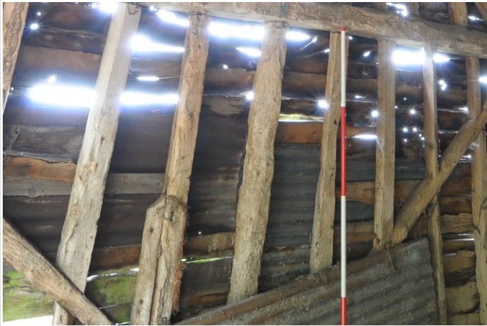
Fig. 18 - Studs, west gable
