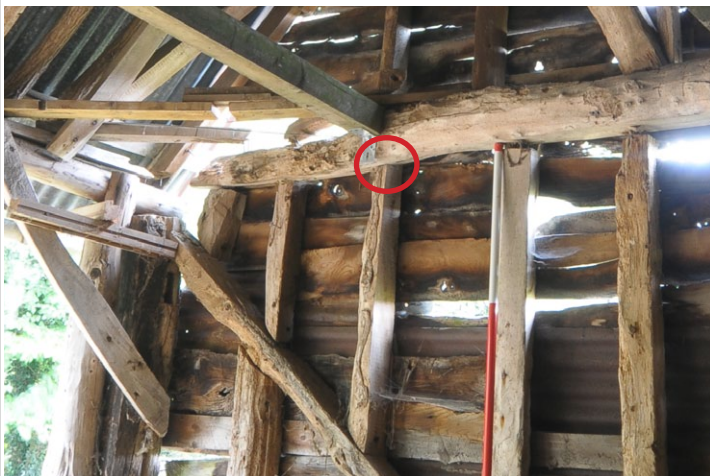
Fig. 20 - Notched stud attached to tiebeam, west gable
