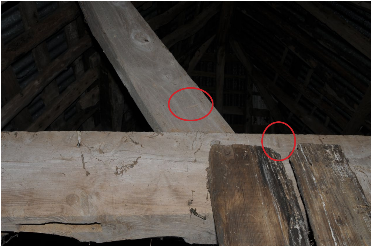
Fig. 33 - Assembly marks on eastern truss
