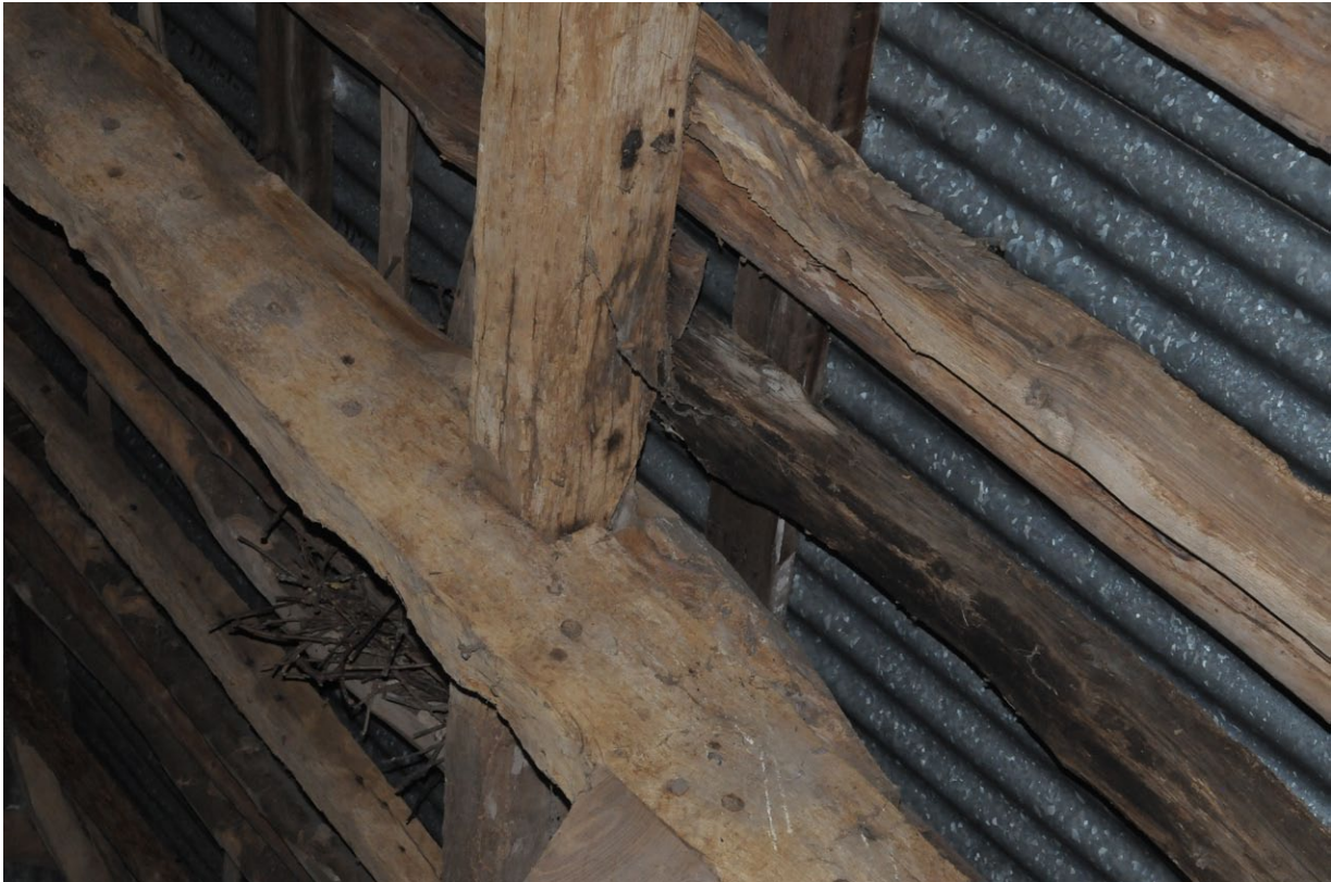
Fig. 24 - Shot of southern purlin showing trenching
