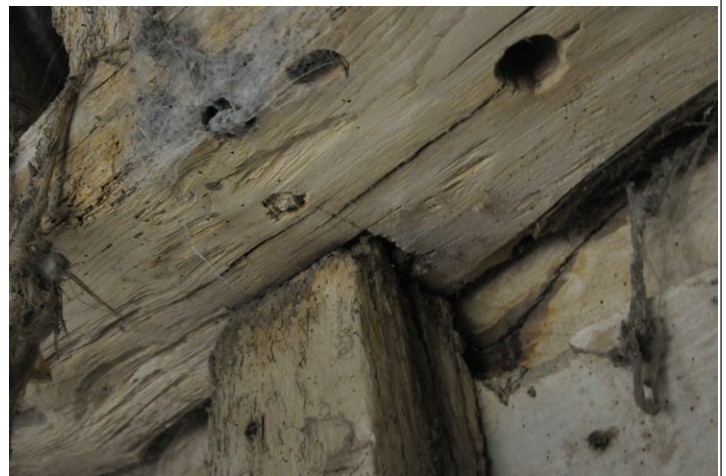
Fig. 21 - Stud mortised to wall plate, east end of rear wall
