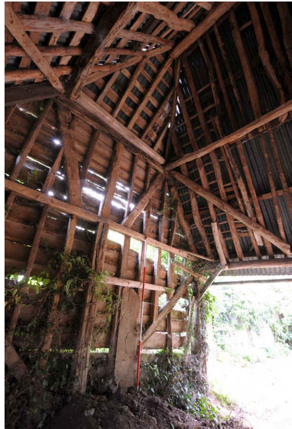
Fig. 15 - Interior shot of E gable
