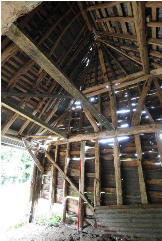
Fig. 14 - Interior shot of W gable
