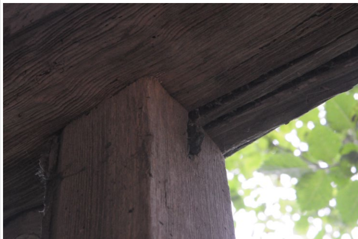
Fig. 22 - Stud mortised and nailed to tiebeam, east gable
