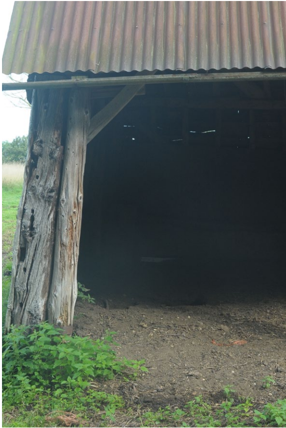
Fig. 31 - The round pole replacing the original post, south-west corner
