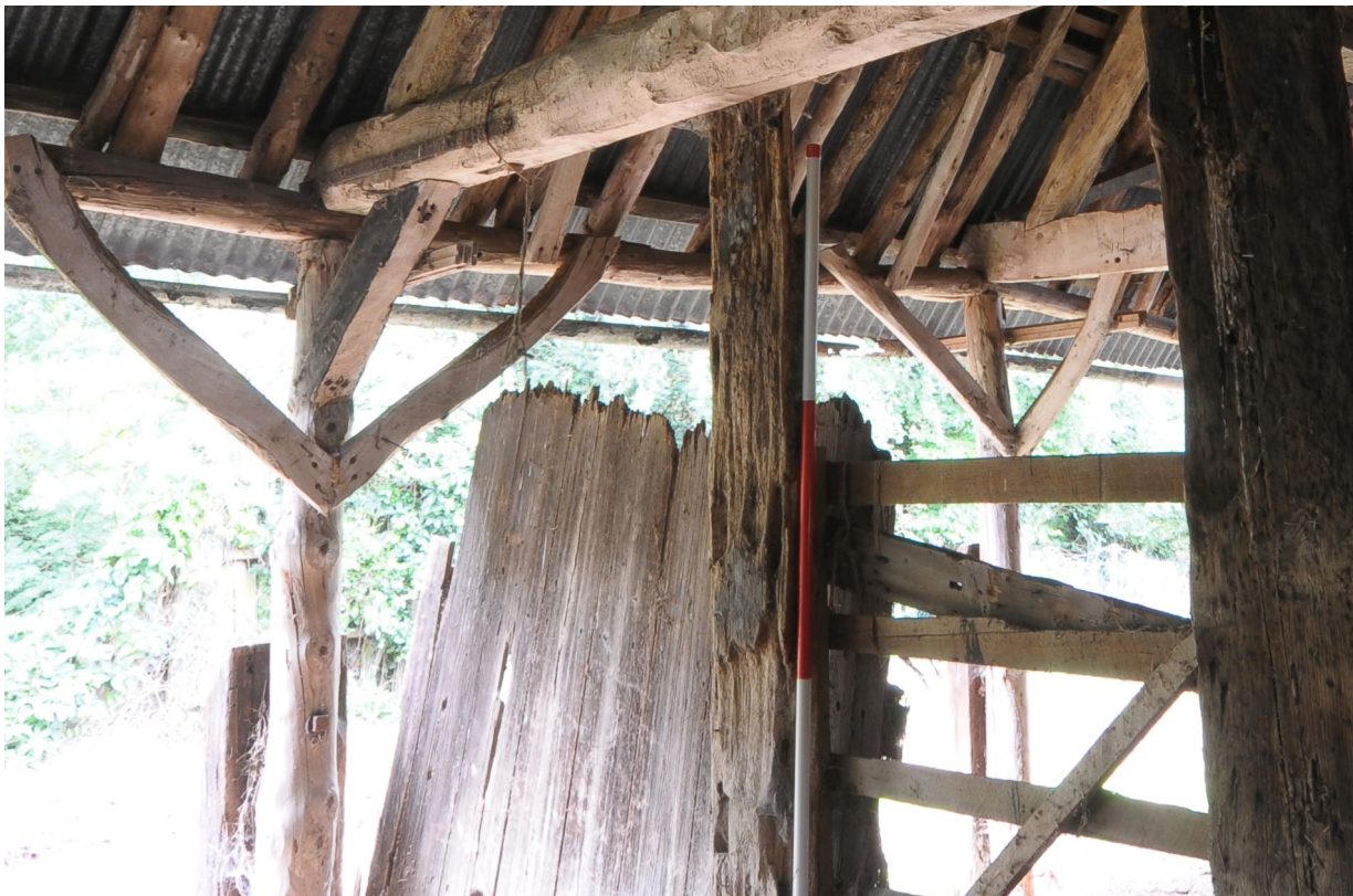
Fig. 17 - Shot of bressumer beam and bracing supporting central posts
