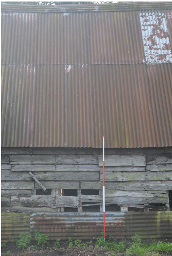
Fig. 10 - Centre of the rear elevation
