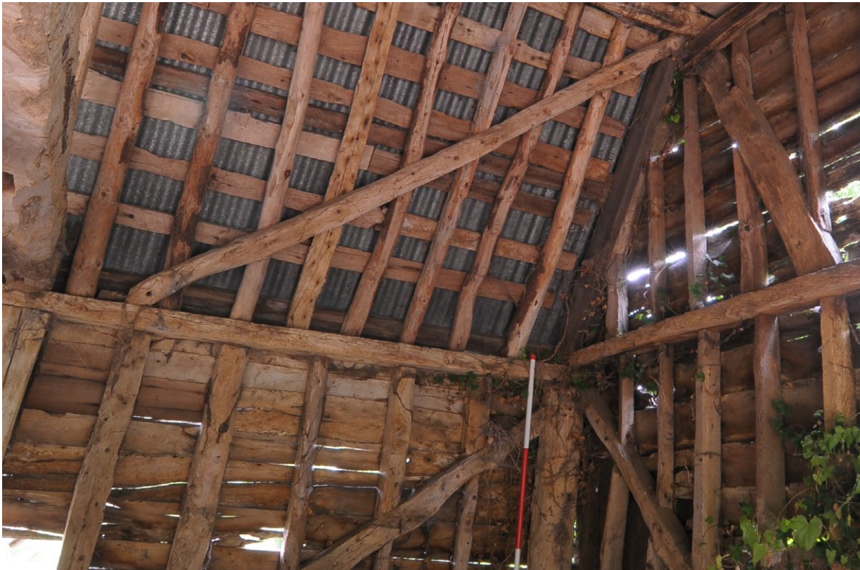
Fig. 27 - Rafter bracing, east end of northern pitch
