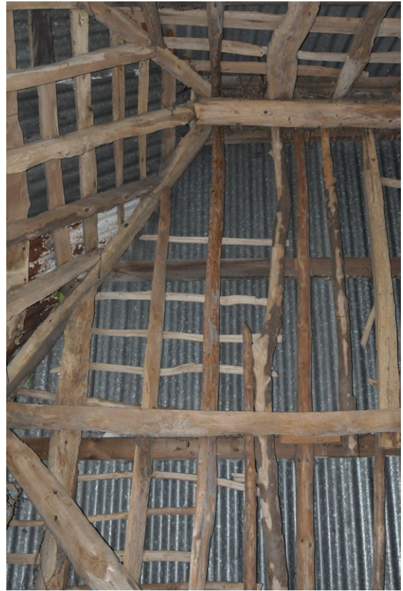
Fig. 29 - Shot of split laths, east end of south pitch
