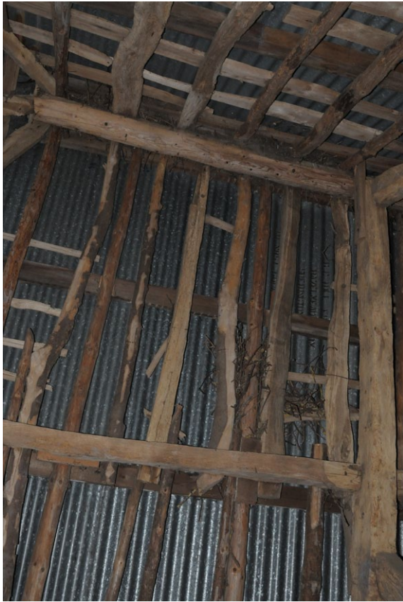
Fig. 28 - General shot of rafters, south pitch
