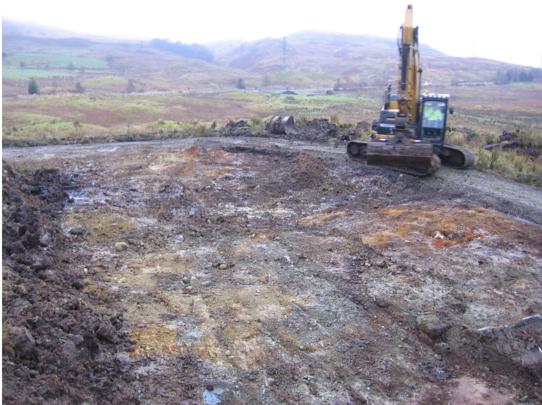
Fig. 5 Topsoil stripping for the storage area
