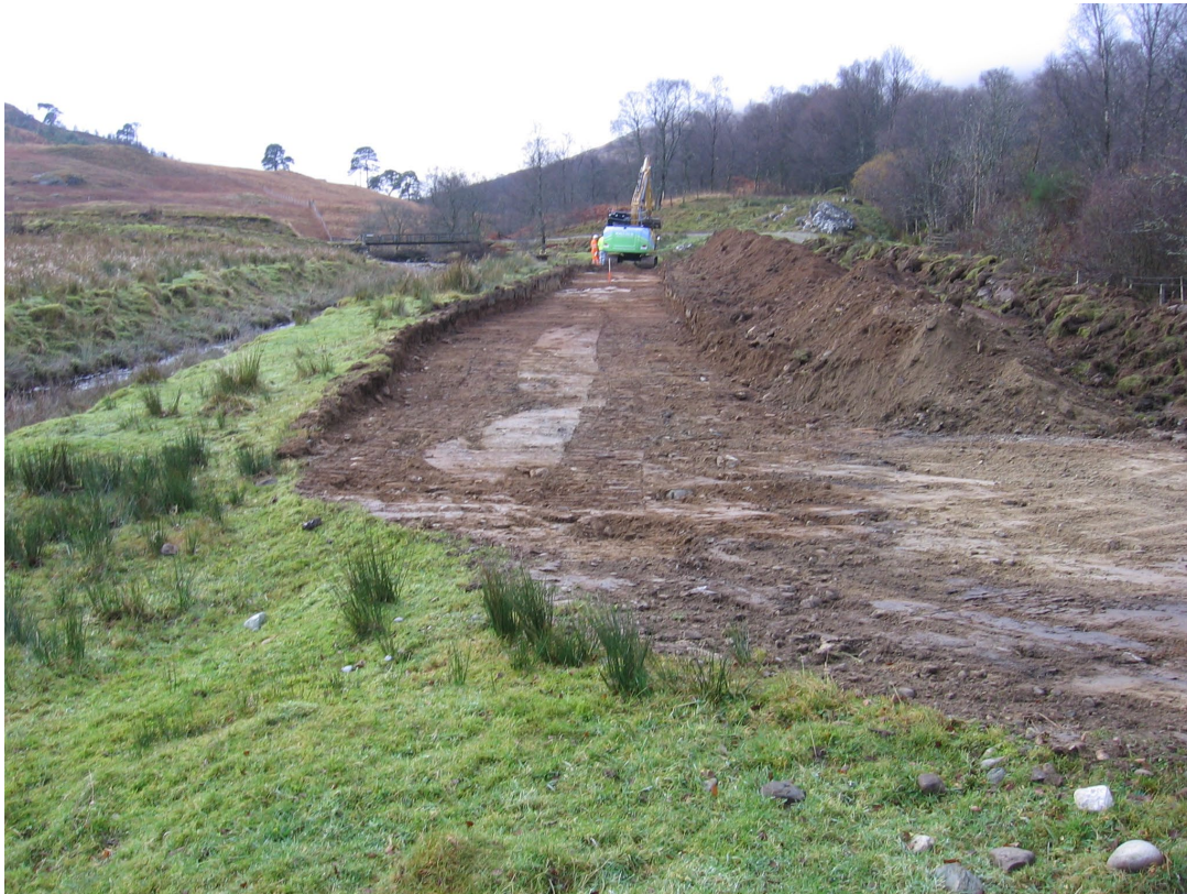
Fig. 4 Topsoil stripping for the access road
