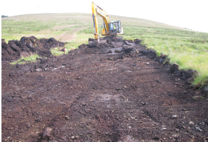
Fig. 4 - General view of topsoil stripping between existing wind farm and turbine 17
