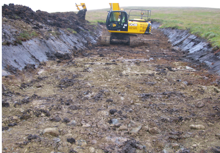
Fig. 5 - General view of topsoil stripping between turbines 17 and 18
