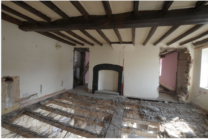
Fig. 19 - Shot of west room, 1st floor, Unit 1, looking east
