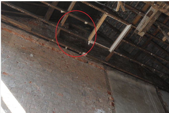
Fig. 33 - Blocked window at east end of Unit 1 attic, shot taken from Unit 2, view north-west
