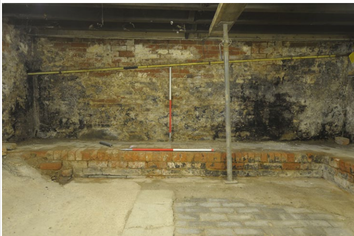
Fig. 11 - West elevation of Cellar, Unit 1, looking west
