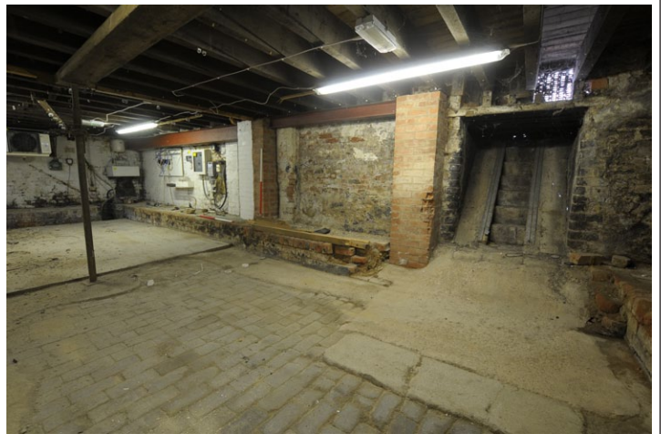
Fig. 10 - The Cellar, Unit 1, looking south-east
