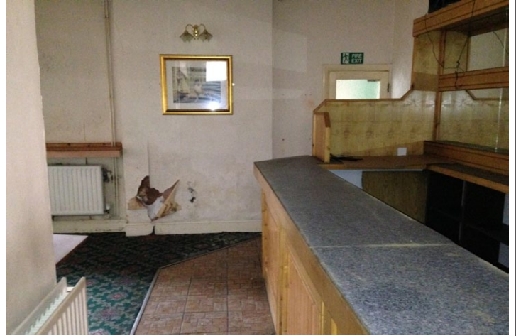
Fig. 38 - Internal view of lower floor of Unit 3, looking east
