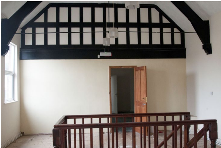
Fig. 44 - Upper floor of Unit 4 prior to removal of modern partition, looking east
