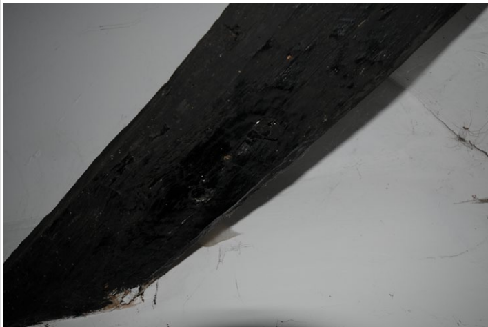
Fig. 35 - Shot of unused pegged holes, corner tie in south-east corner of east room, 2nd floor (attic), Unit 1, looking east
