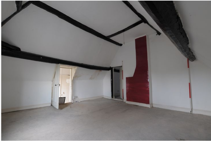
Fig. 31 - Shot showing fireplace in west room, 2nd floor (attic), Unit 1, looking north-east
