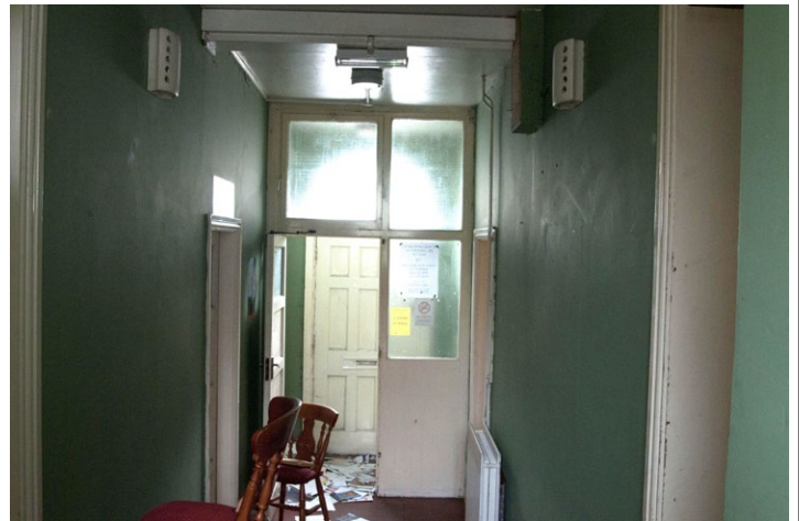
Fig. 36 - Internal view of lower floor of Unit 2, looking south
