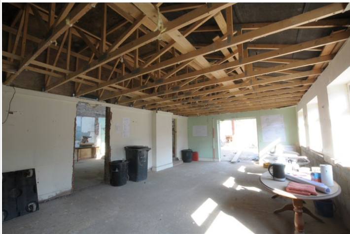
Fig. 48 - Interior of Unit 5, looking north-west
