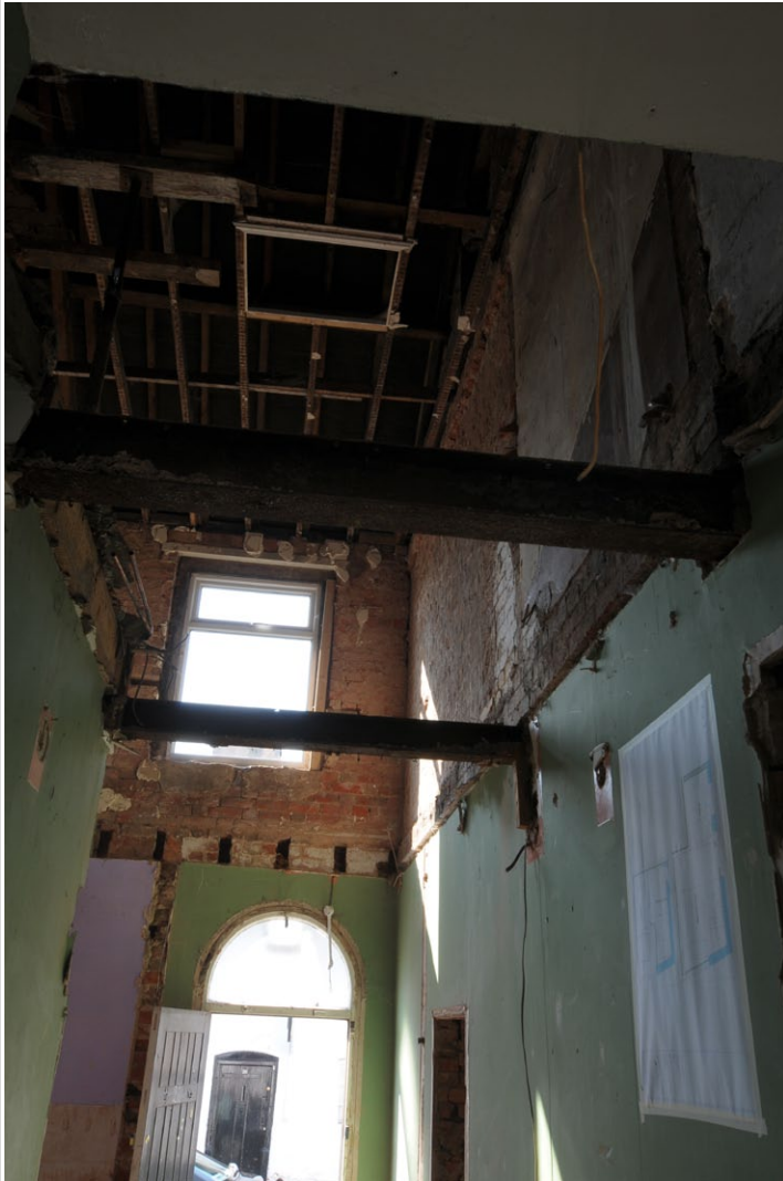
Fig. 37 - Internal view of lower floor of Unit 2 after ceiling removed, looking South
