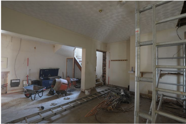
Fig. 46 - South end of the ground floor of Unit 4, looking south-west
