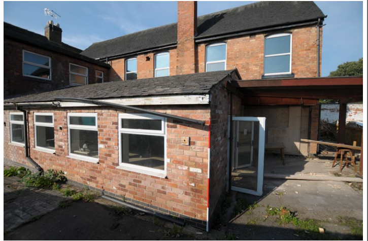
Fig. 47 - The exterior of Unit 5, looking south-west
