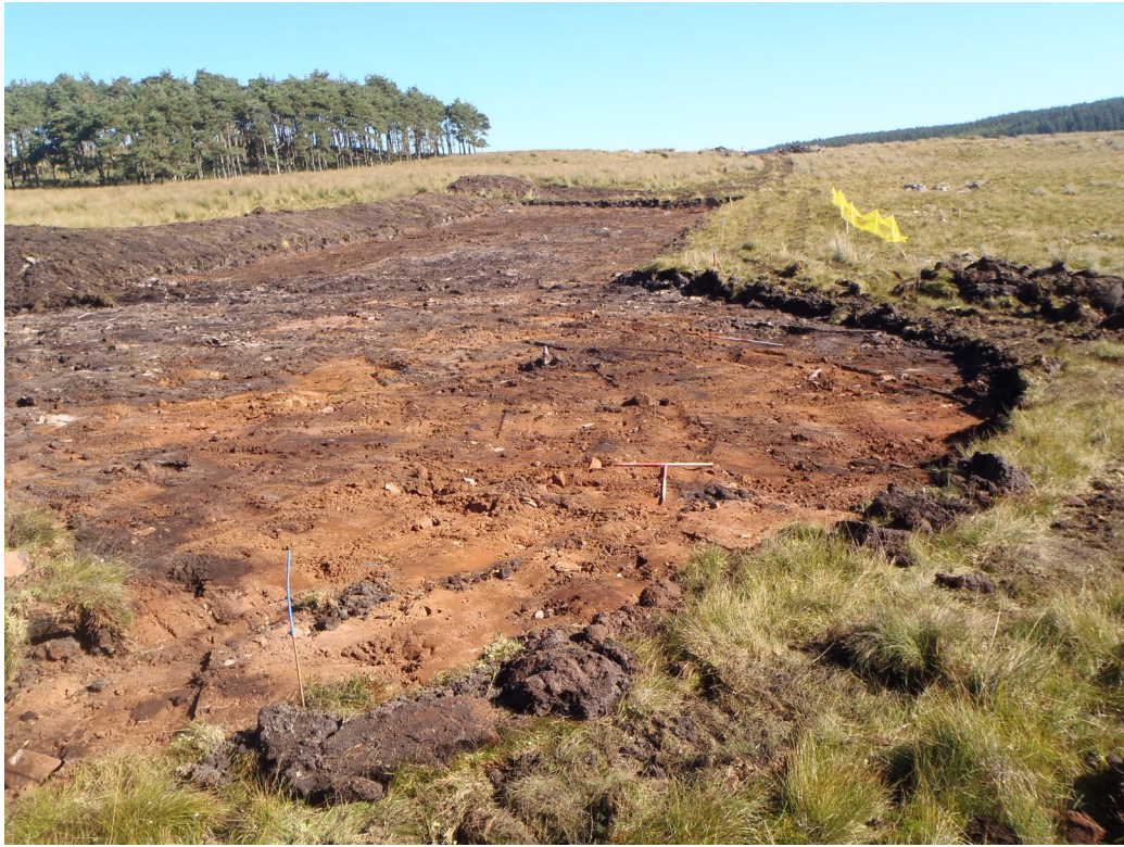
Fig. 4 Site 9 fenced off next to excavated Crane Pad at Turbine 11
