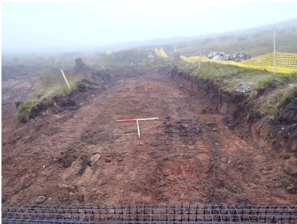
Fig. 3 Access road at Turbine 9 junction
