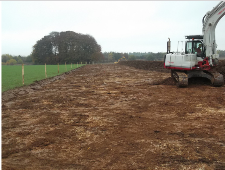
Fig. 3 - Easement strip towards western end of pipeline, looking south-west
