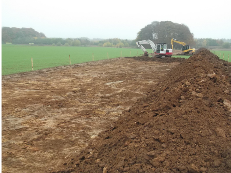
Fig. 4 - Easement strip towards centre of pipeline, looking south-west
