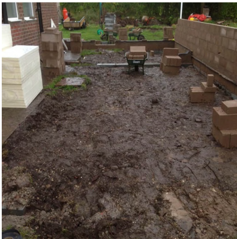
Fig. 4 - Footprint of extension following the removal of deposits between foundations
