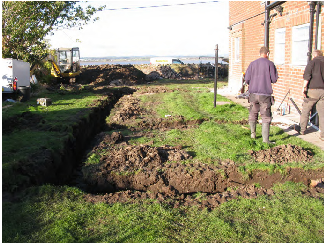
Fig. 2 - Post-excitation of the foundation trenches on the western side of the existing domestic structure
