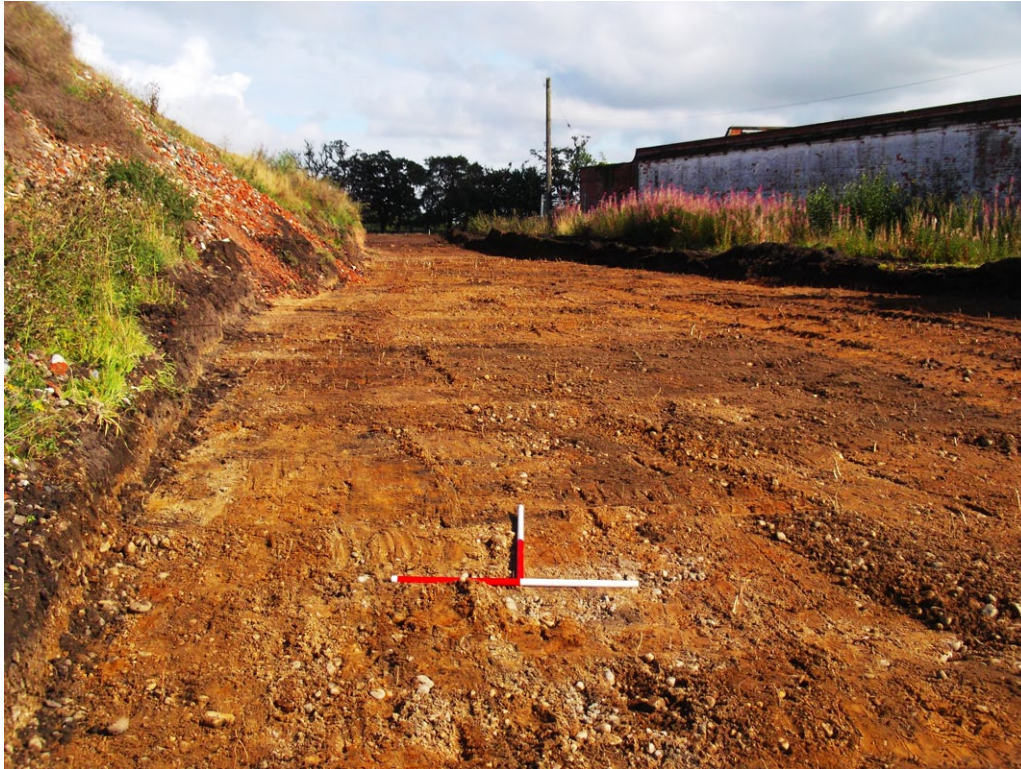
Fig. 12 - Area 2.4 being stripped, looking NE
