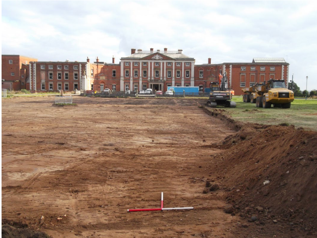
Fig. 18 - General shot of Area 4 being stripped, looking SE
