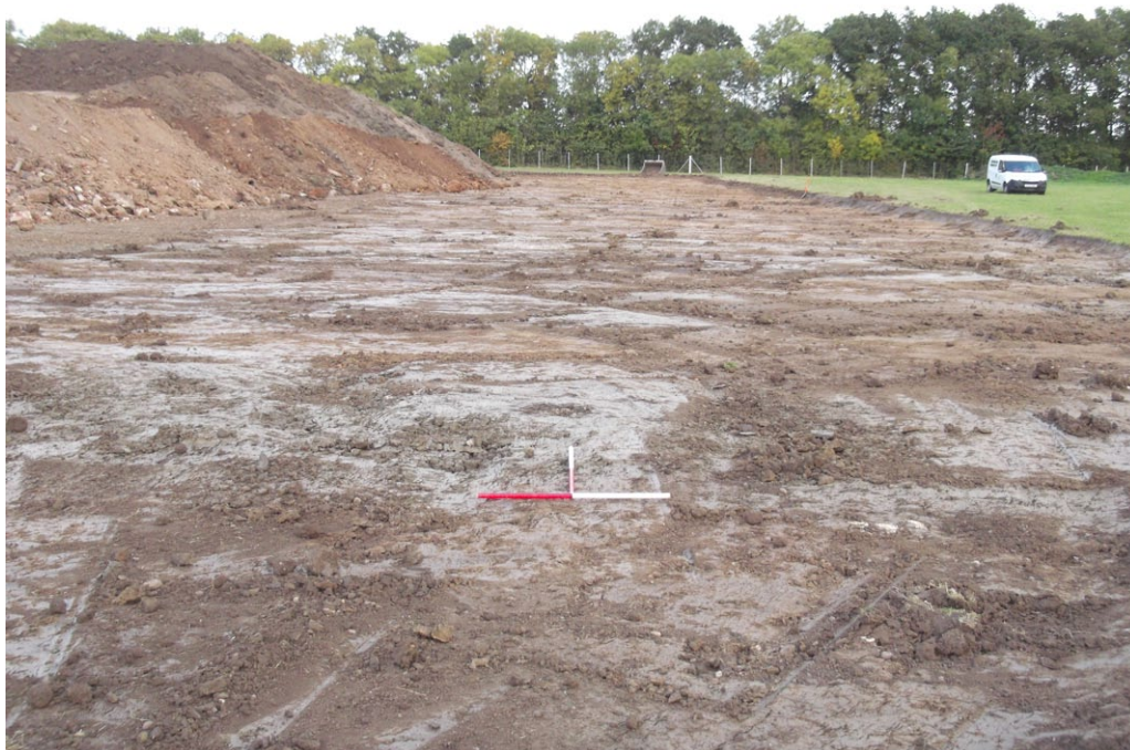
Fig. 25 - Area 6 after stripping, looking NE
