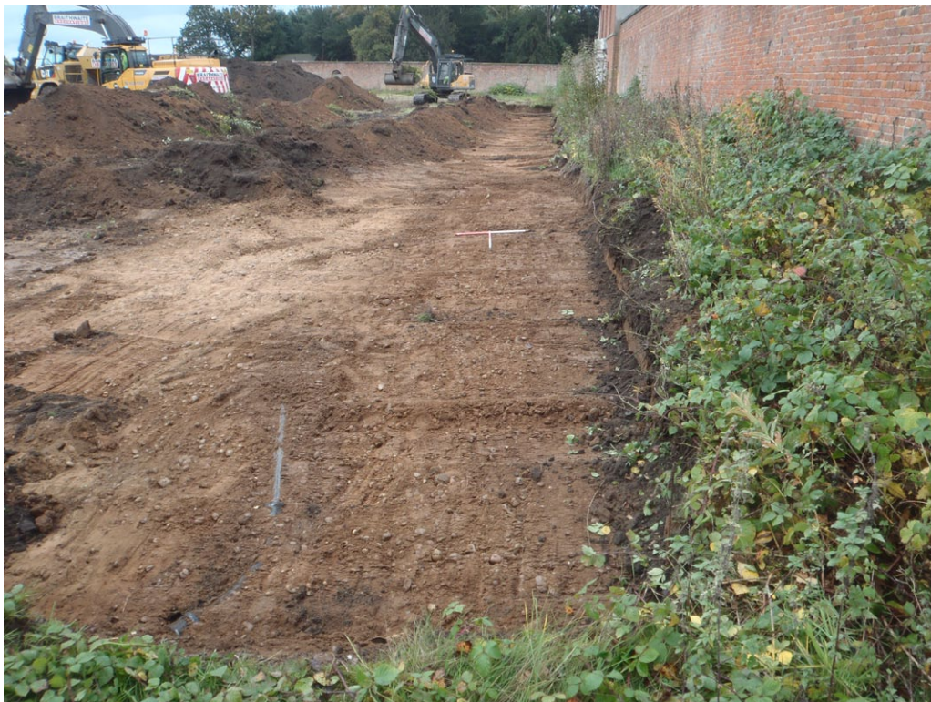
Fig. 15 - Area 2.5, the Walled Garden, being stripped of topsoil, looking SE
