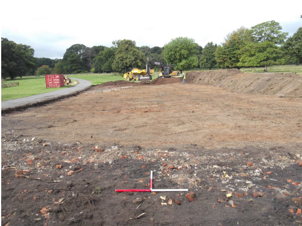
Fig. 17 - Area 3 during stripping, looking NW
