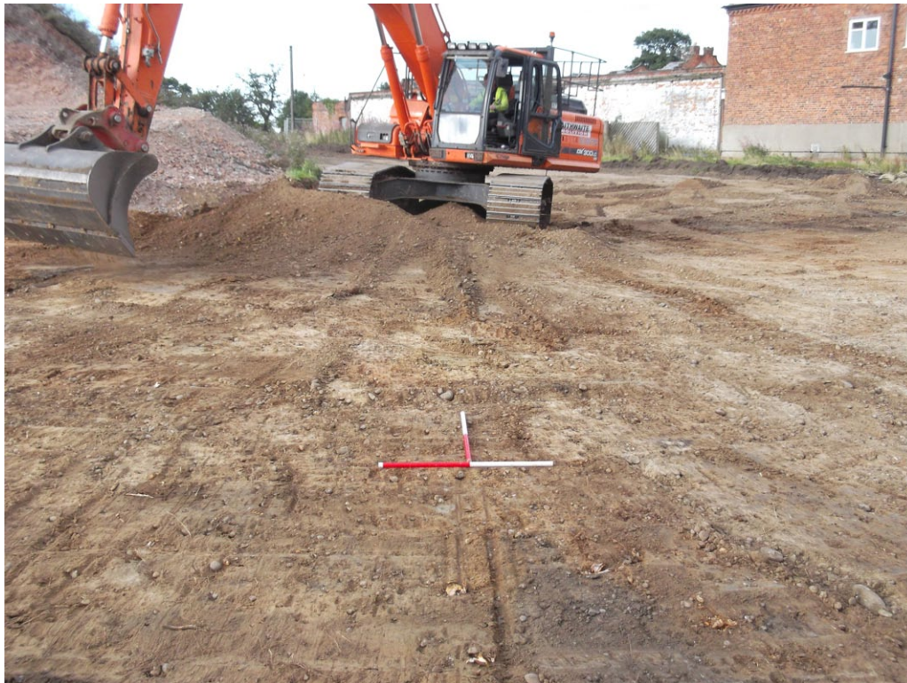
Fig. 10 - Area 2.1 being stripped, looking NE
