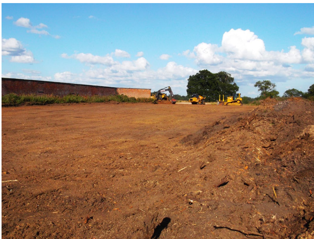
Fig. 11 - Area 2.3 during topsoil stripping
