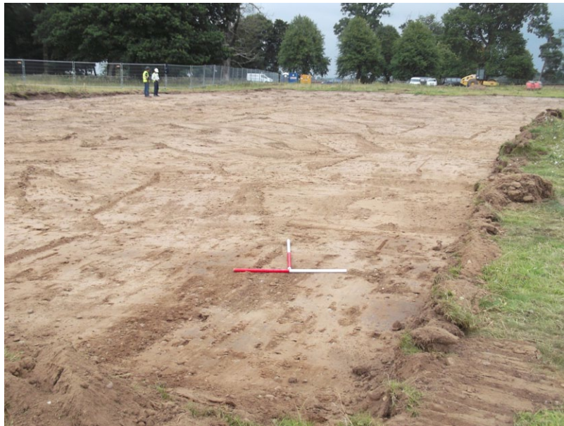
Fig. 9 - General shot of Area 1 being stripped of topsoil, looking NE
