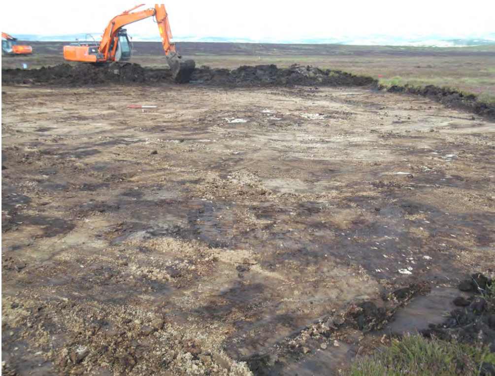
Fig. 3 Crane Pad at Turbine 5 after strip, looking north-east
