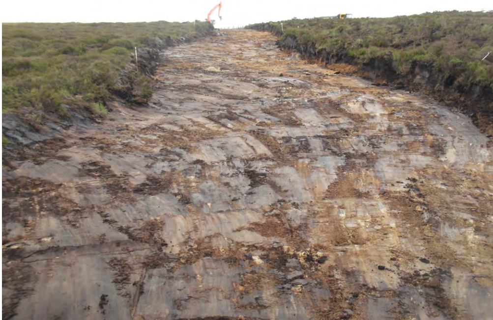
Fig. 8 New access track after strip, looking south
