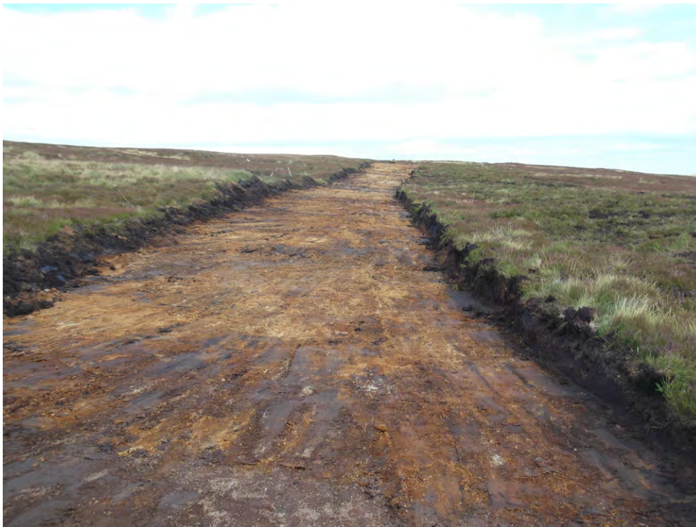
Fig. 7 Spur road towards Turbine 9 after strip, looking north-east
