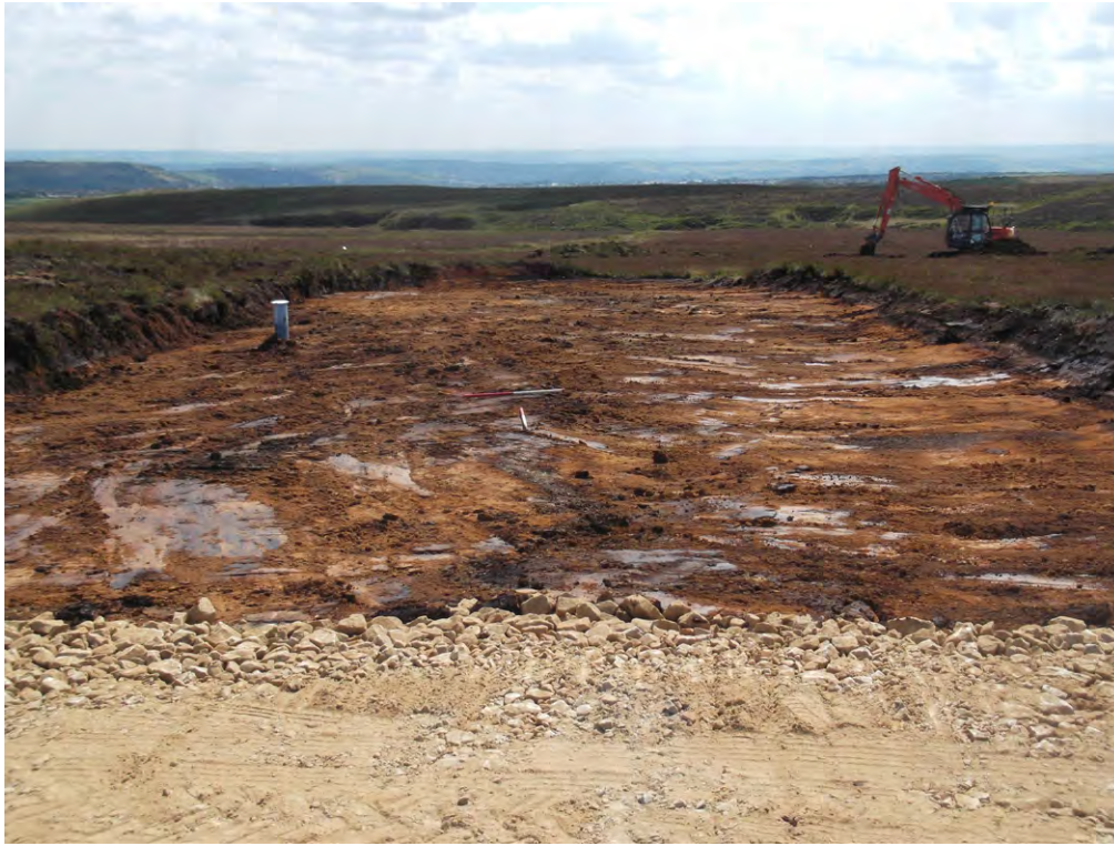
Fig. 6 Crane pad at Turbine 9 after strip, looking south-east
