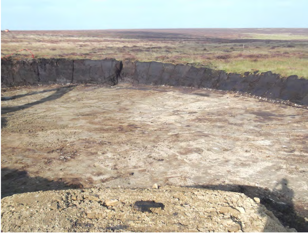
Fig. 2 Turbine Base at T2 after strip, looking north-east
