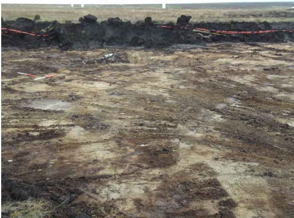
Fig. 5 Crane Pad at T7 after strip, looking north
