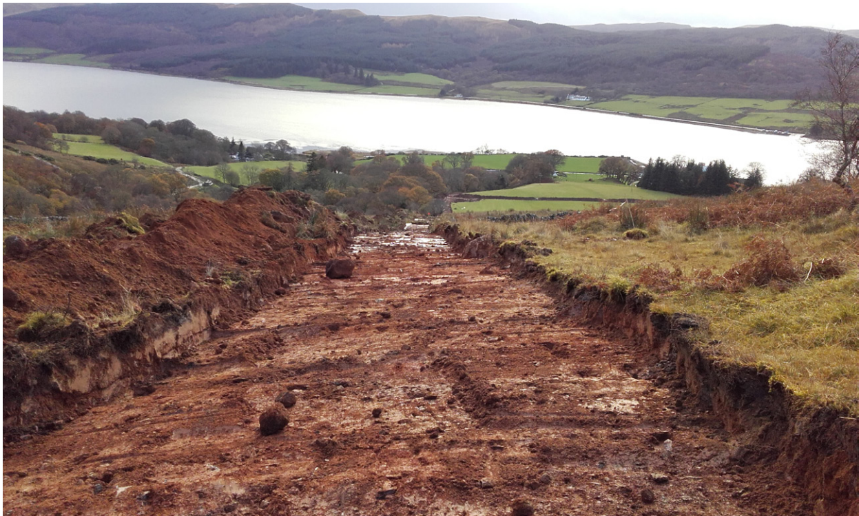
Fig. 10 General shot of main watching brief area (from the north-north-east)
