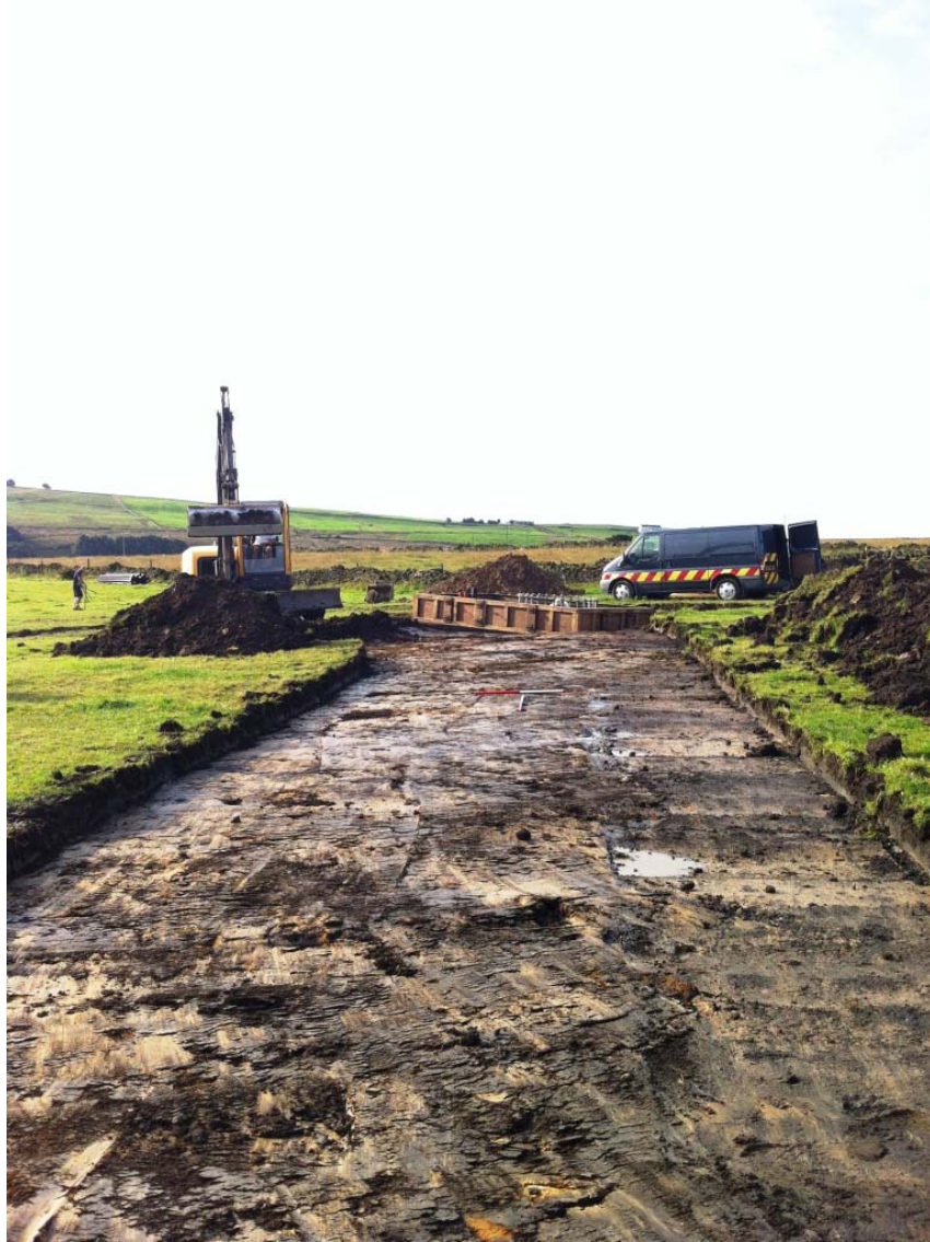
Plate 3: Access Track, Post-excavation
