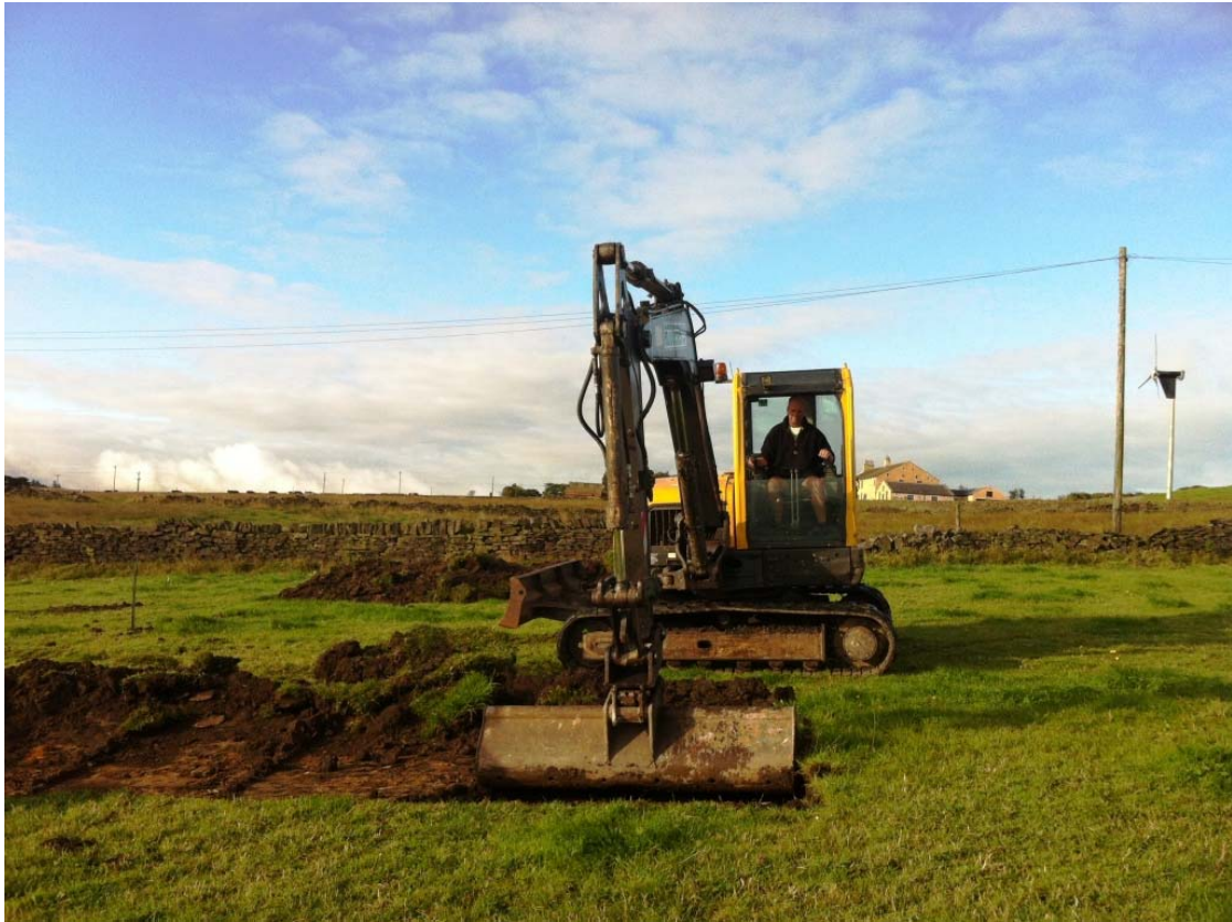
Plate 1: Working Shot, Stripping the Turbine Base
