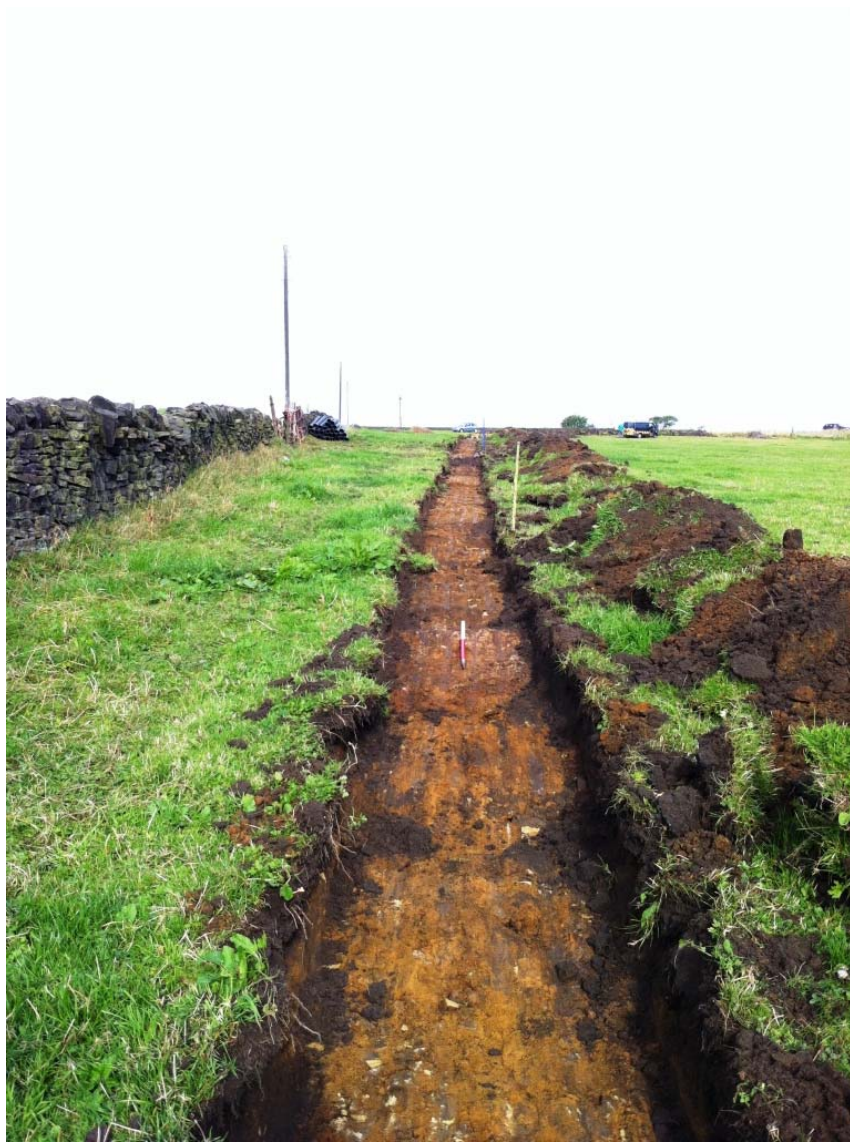
Plate 4: Cable Trench, Post-excavation
