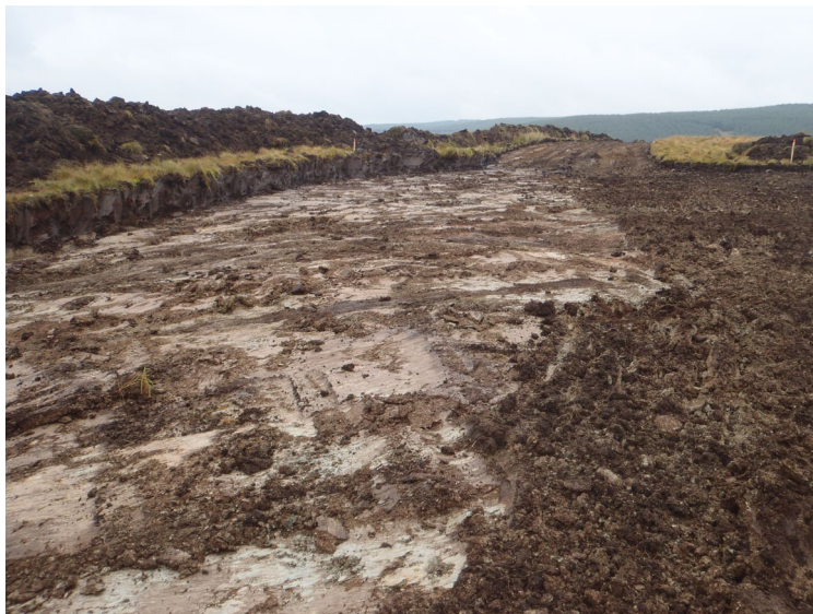
Fig. 9: Topsoil stripping within buffer zone at SAM12666
