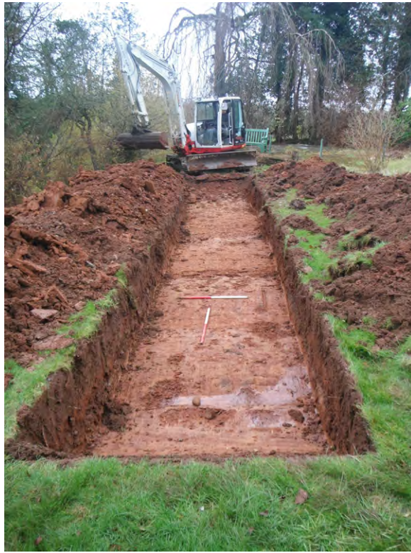
Fig. 2.1 Trench 1, general shot facing north-west
