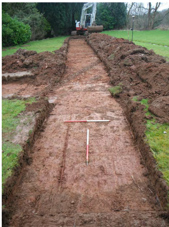
Fig. 2.4 Trench 3, general shot facing south
