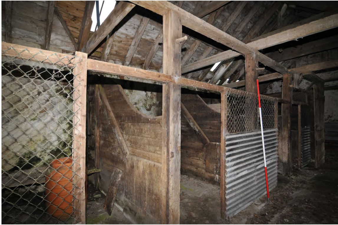
Fig. 26 Loose boxes within the stable
