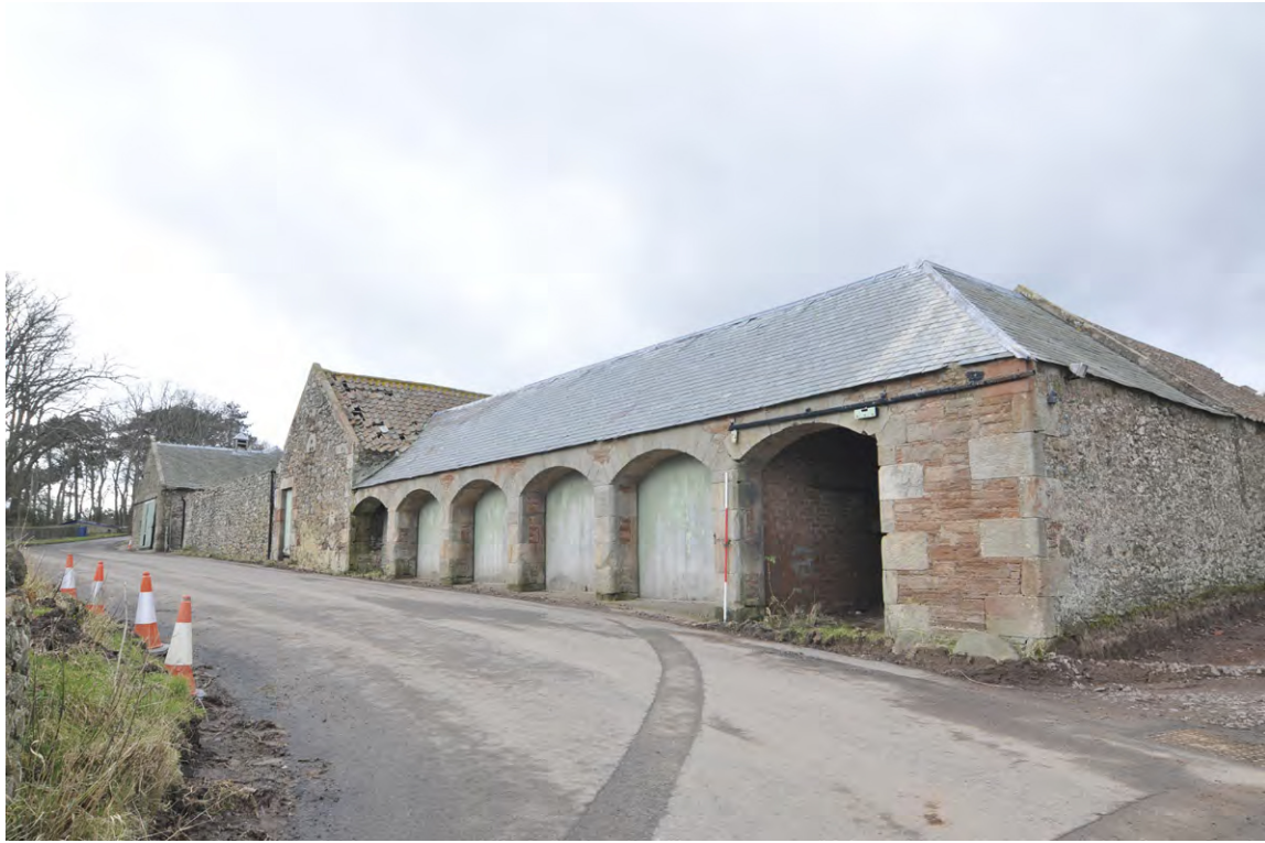
Fig. 10 South Range with cart sheds and central range gable
