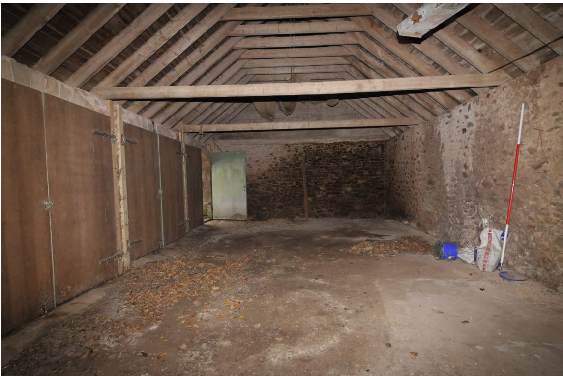
Fig. 15 Cart shed, Unit 2, interior
