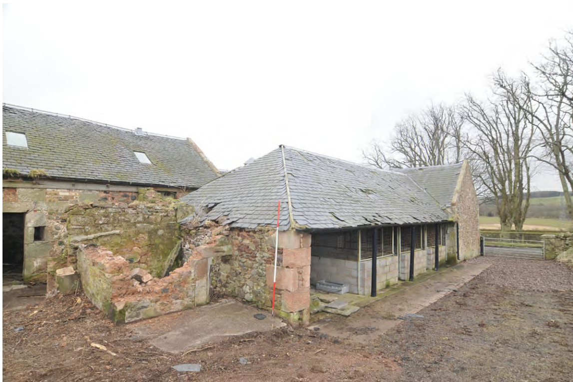
Fig. 25 Open sided shed/kennels with cast-iron columns, Unit 27
