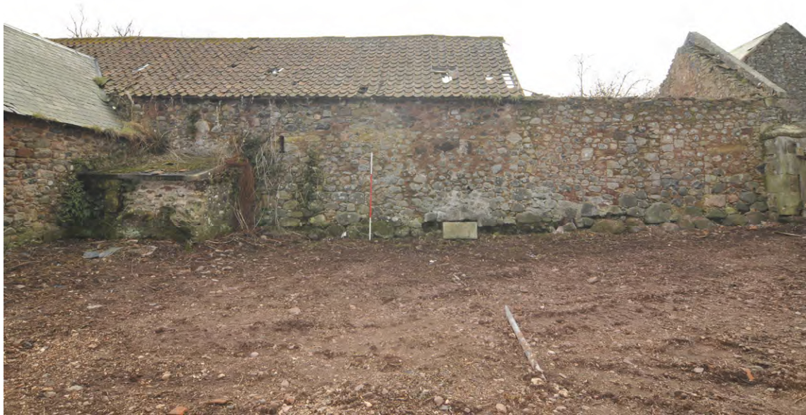
Fig. 13 Central Range, east-facing elevation
