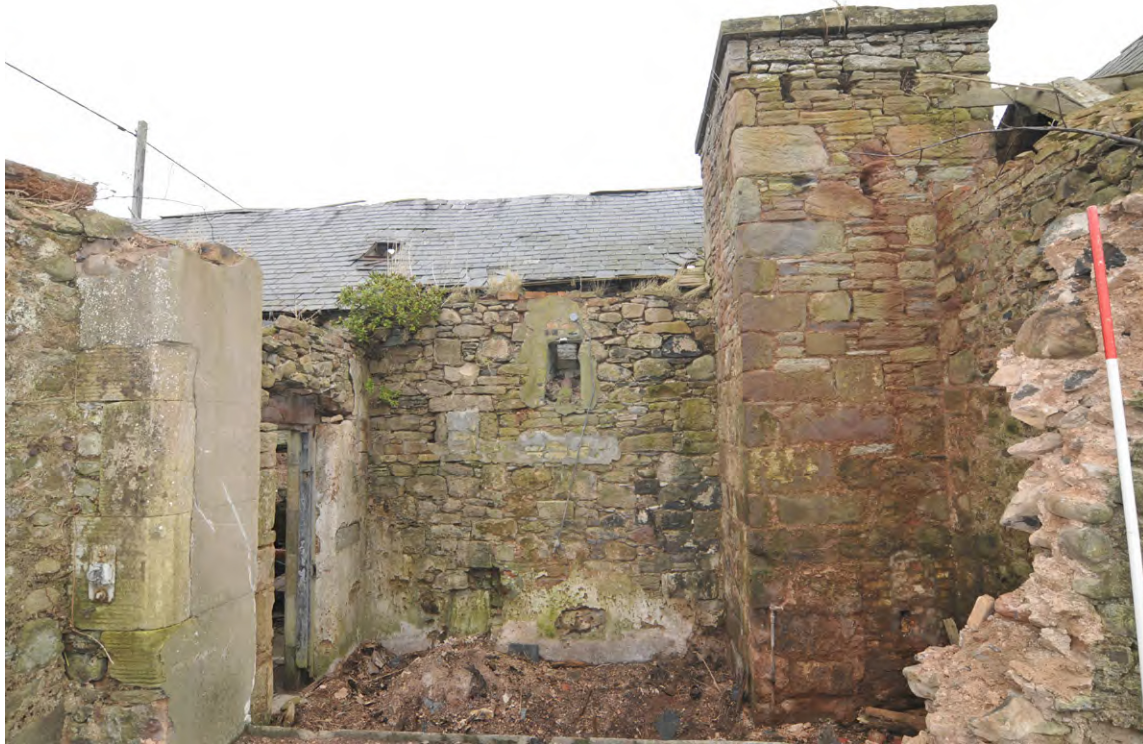
Fig. 22 Boiler house chimney in Unit 21
