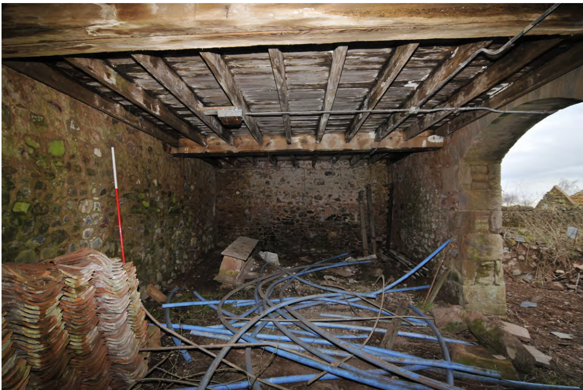
Fig. 19 Interior of the byre, Unit 19
