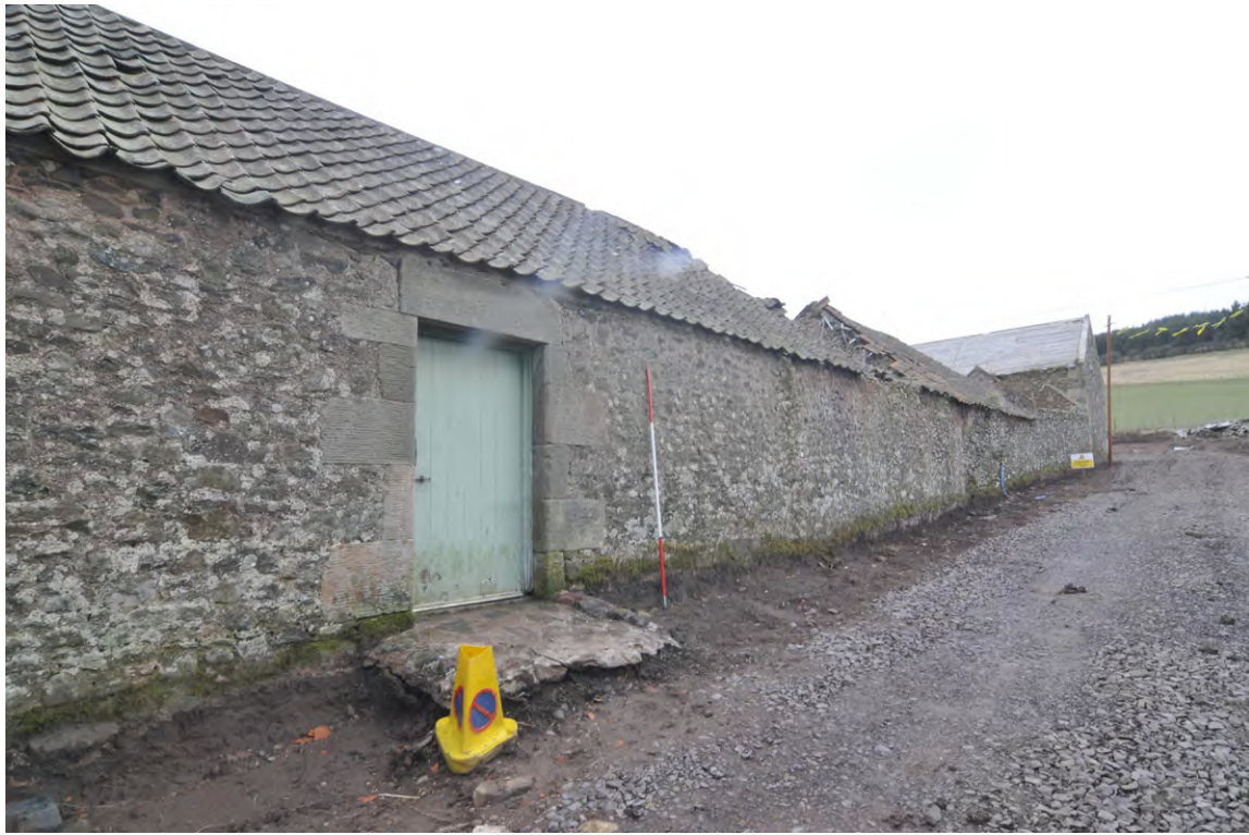
Fig. 8 East Range, east side, looking north
