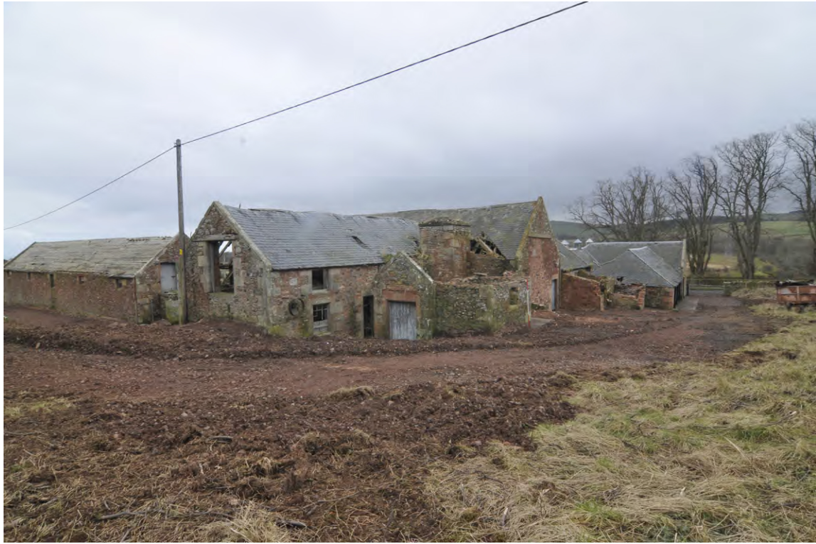
Fig. 12 West Range, general view facing south
