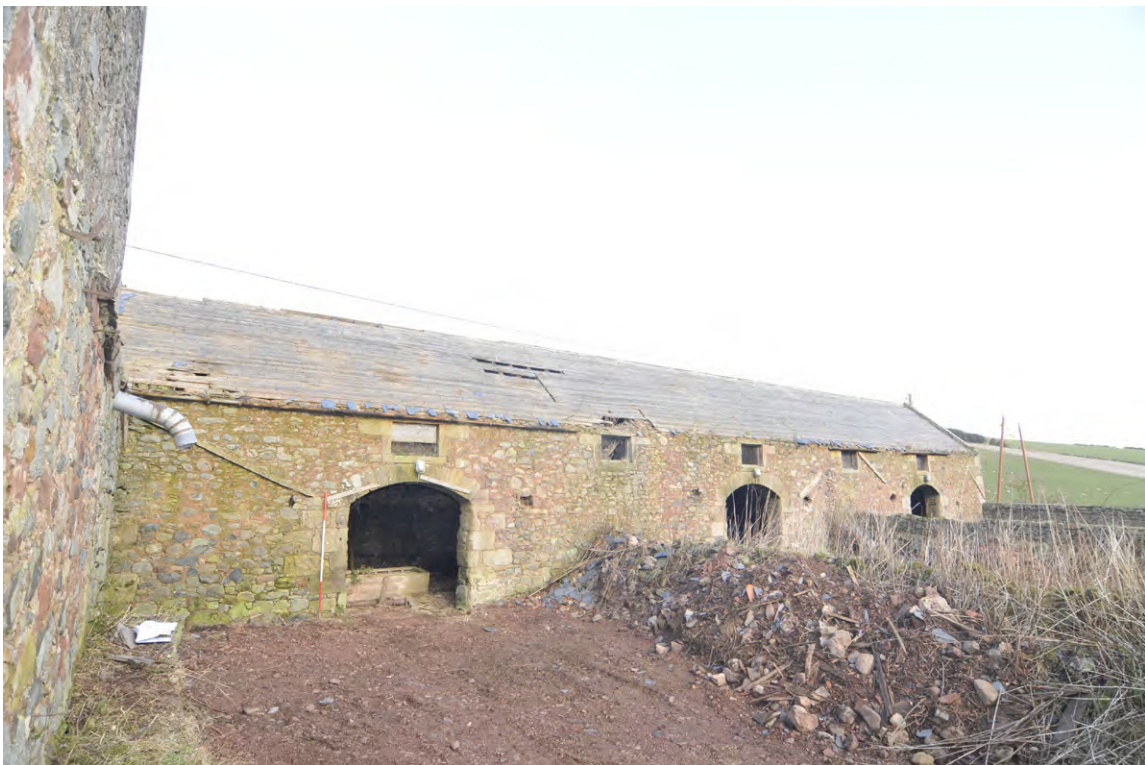
Fig. 7 North Range, south side, looking north-east
