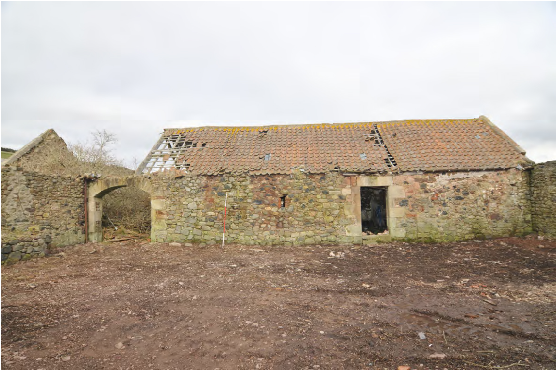
Fig. 14 Central range, west-facing elevation side
