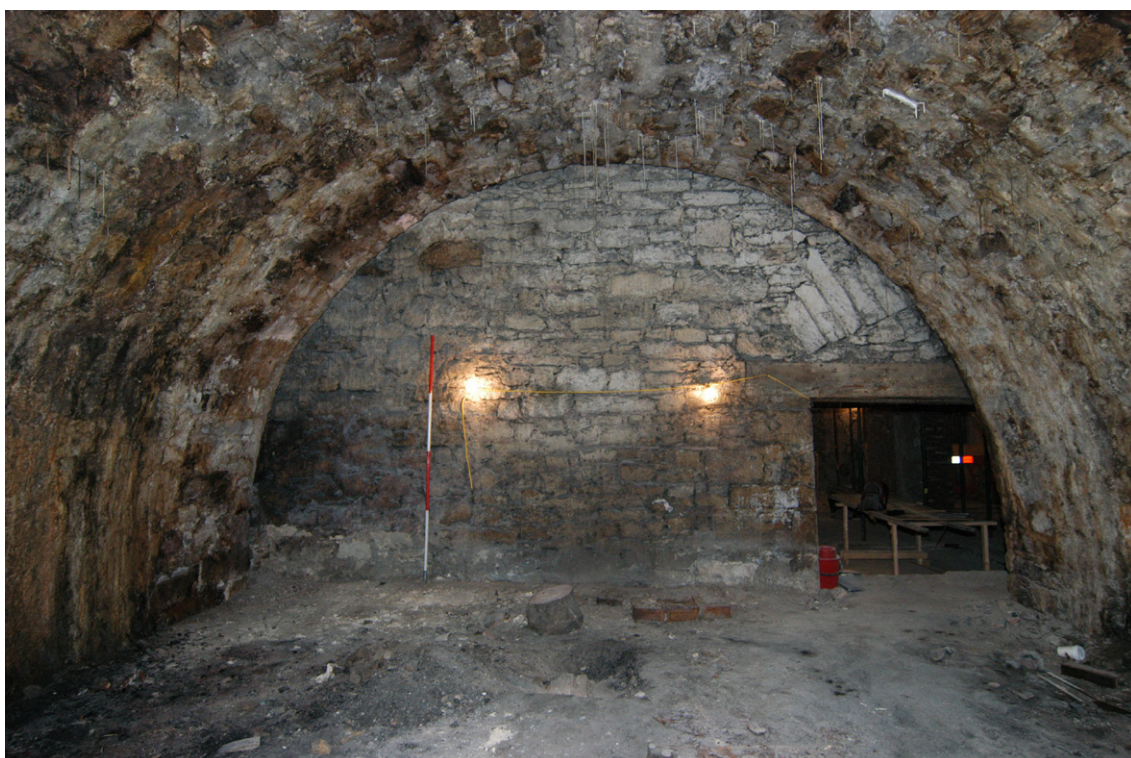
Fig. 7 Interior east-facing elevation of Vault 2 showing part of the larger opening with a segmented relieving arch
