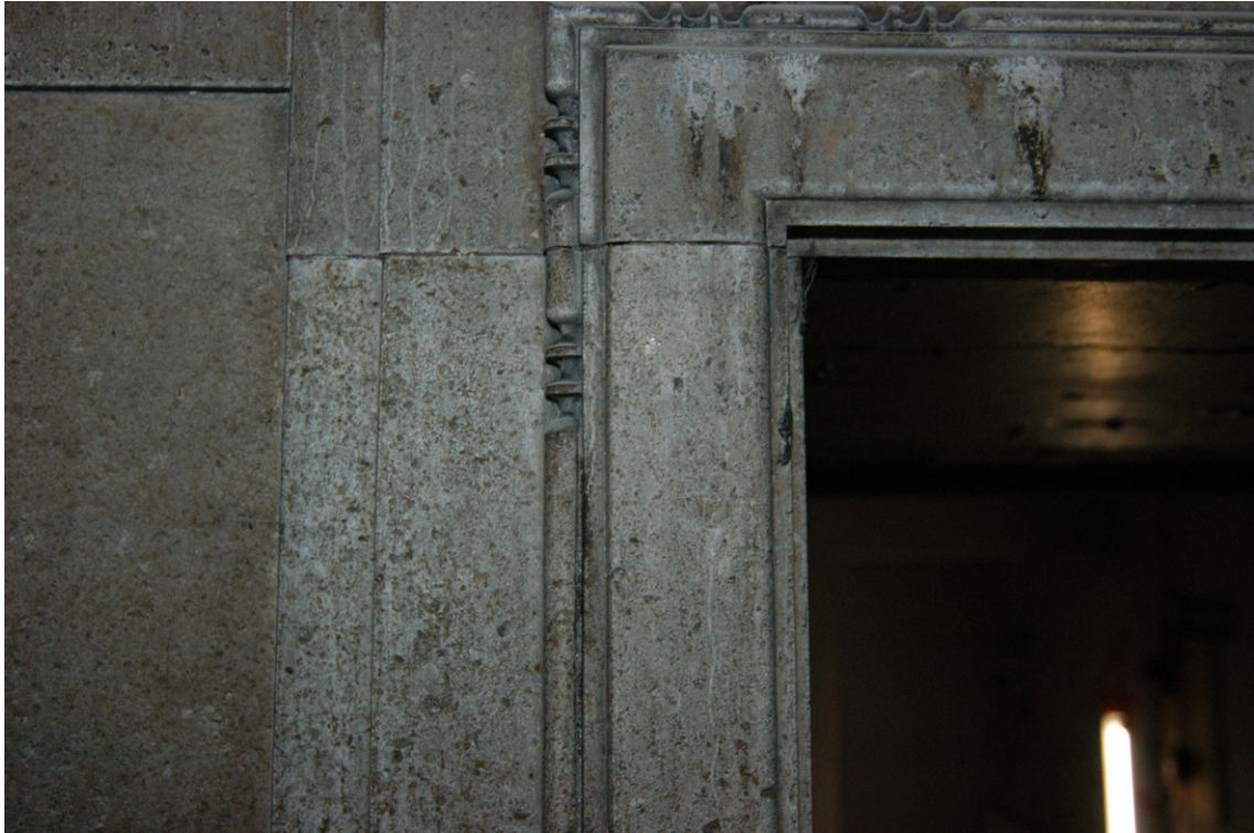
Fig. 14 Detail of the bead-moulding around the marble door frame
