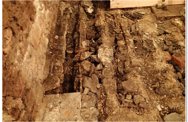
Fig. 3 - Mortered walls and rubble supporting flagstone floor in Room 1/5
