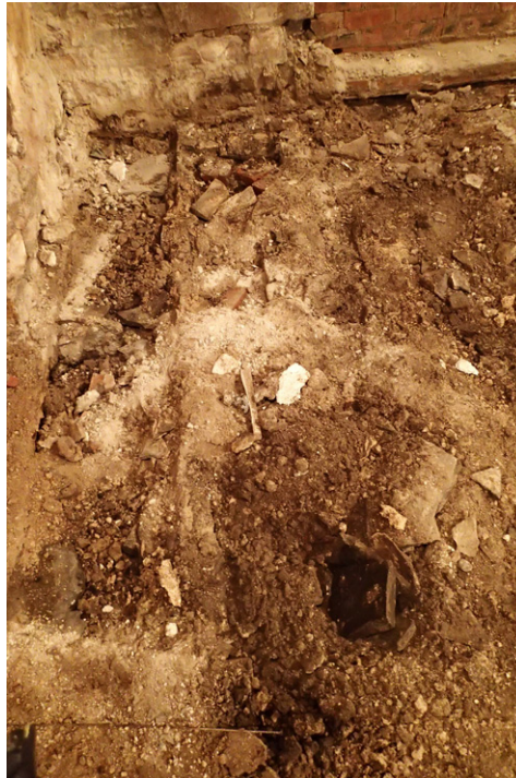
Fig. 4 - Mortered walls and rubble supporting flagstone floor in Room 1/6
