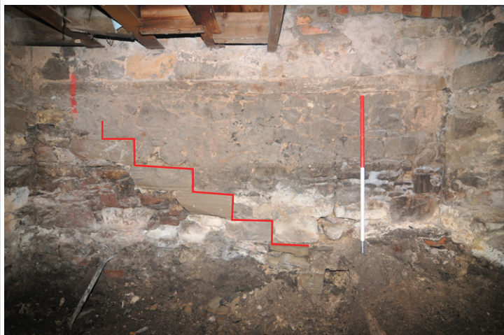
Fig. 10 - Room 1/4, rising stair treads cut flush with the wall on the north-facing elevation
