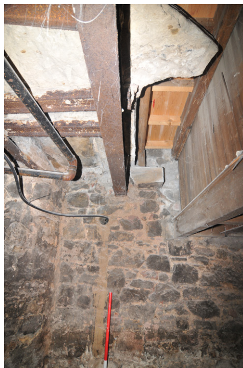
Fig. 9 - Room 1/4, the remains of a stair tread on the south-facing elevation
