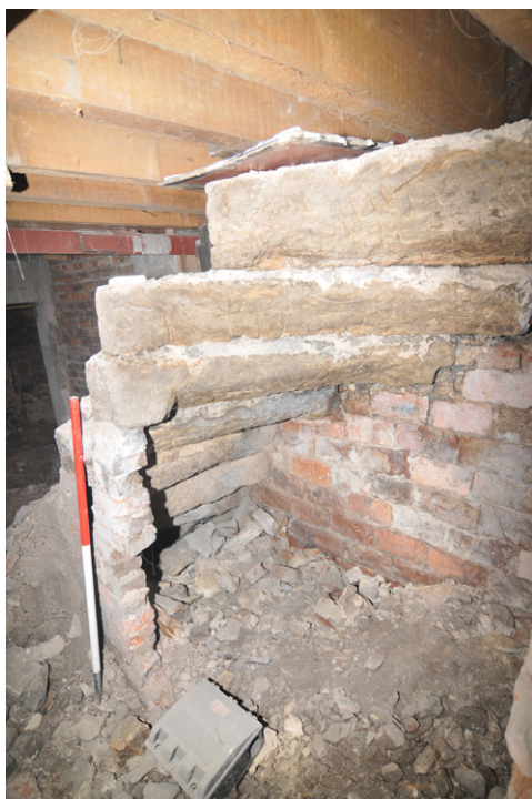
Fig. 8 - Room 1/3, detail of the underside of the stair treads
