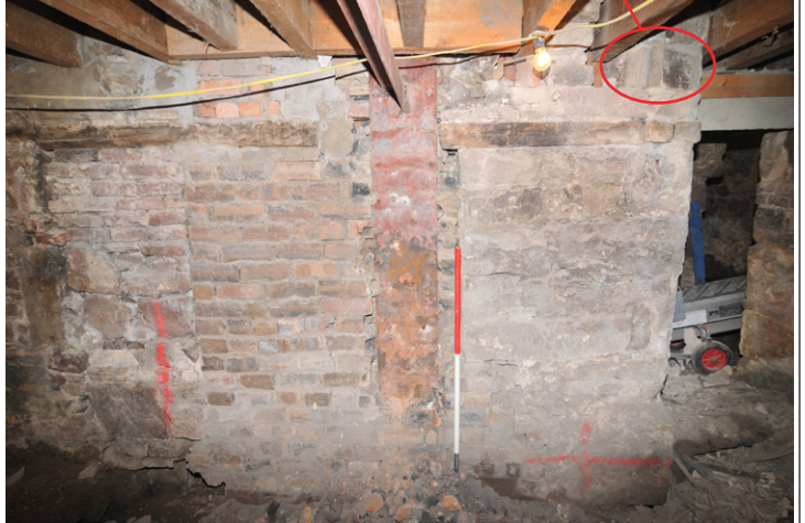
Fig. 13 - Room 1/5, 1930s steel stanchion cutting through a timber wall plate with re-used roll-molded masonry highlighted
