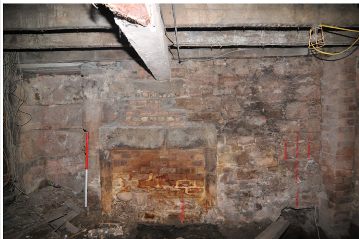
Fig. 3 - Room 1/1, press and blocked fireplace on the south-facing elevation
