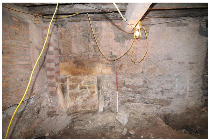
Fig. 5 - Room 1/2, blocked fireplace on the south-facing elevation
