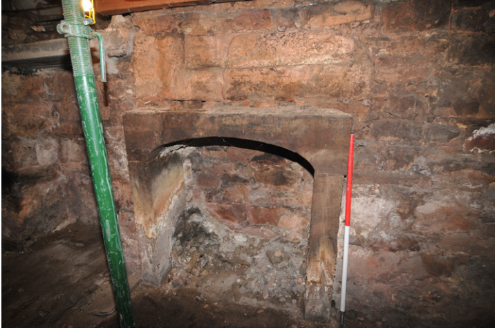
Fig. 17 - Room 1/6, ashlar built fireplace with re-used carved architectural stone in the chimney breast, north-facing elevation
