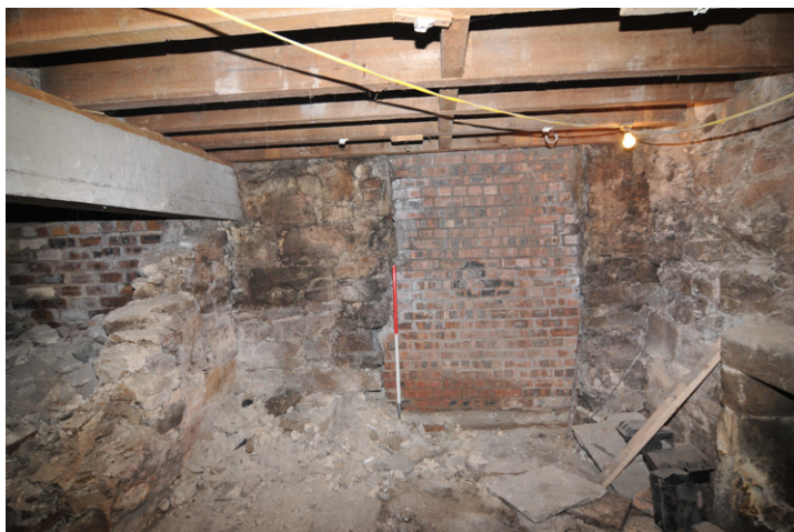
Fig. 11 - Room 1/5, blocked opening on the north-facing elevation
