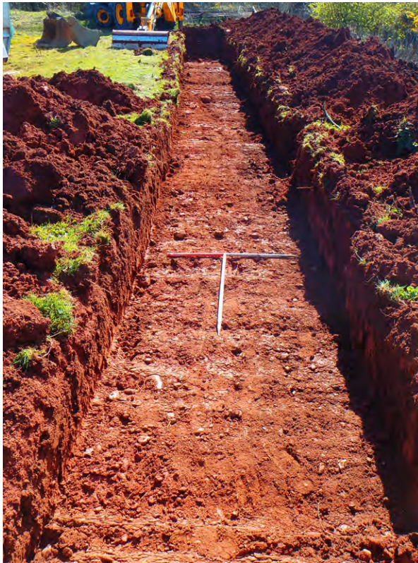
Fig. 2 Trench 2 from the north-west
