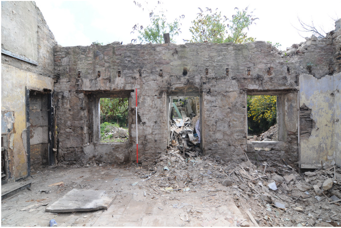
Fig. 20 Unit B, Northwest-facing elevation, with ground floor openings
