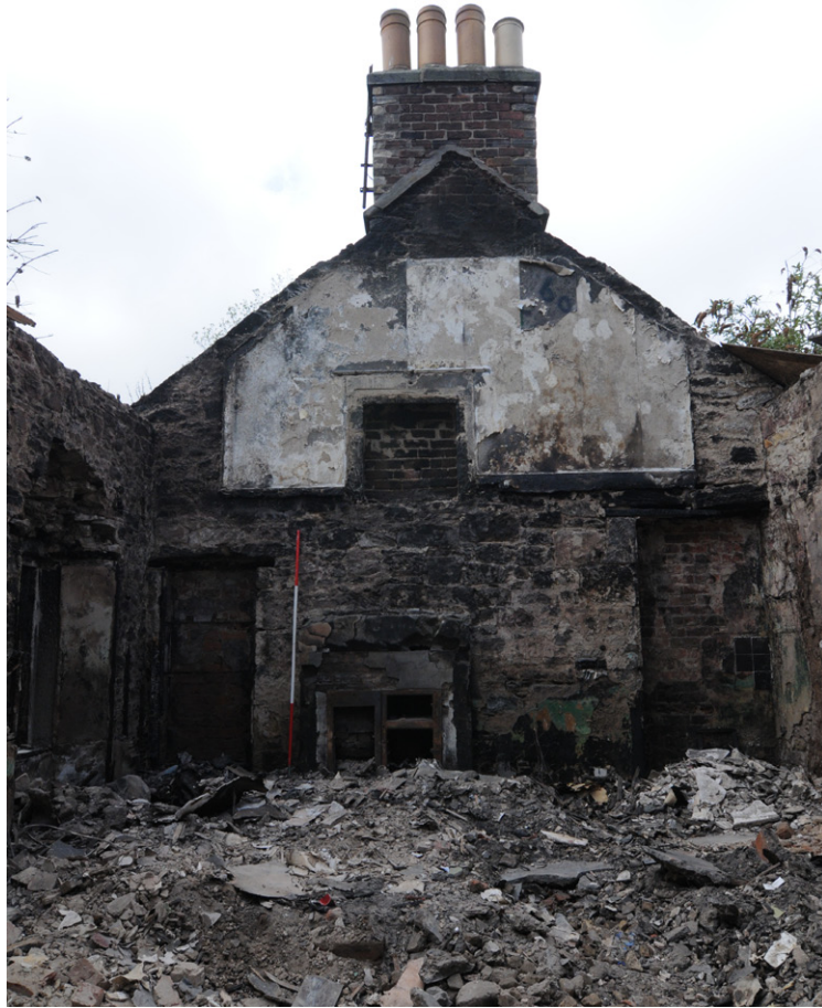
Fig. 16 Unit A, Northeast-facing partition wall showing fireplaces
