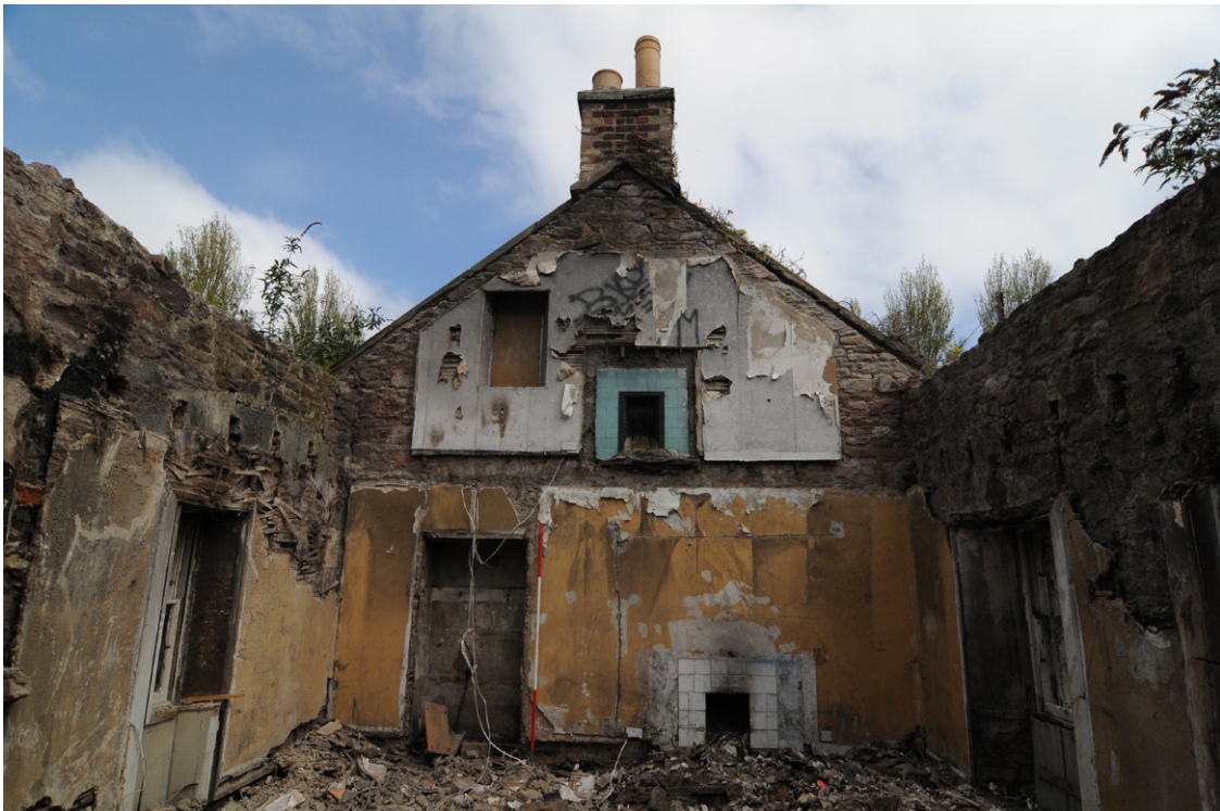
Fig. 19 Unit A, Southwest-facing elevation, gable wall with fireplaces
