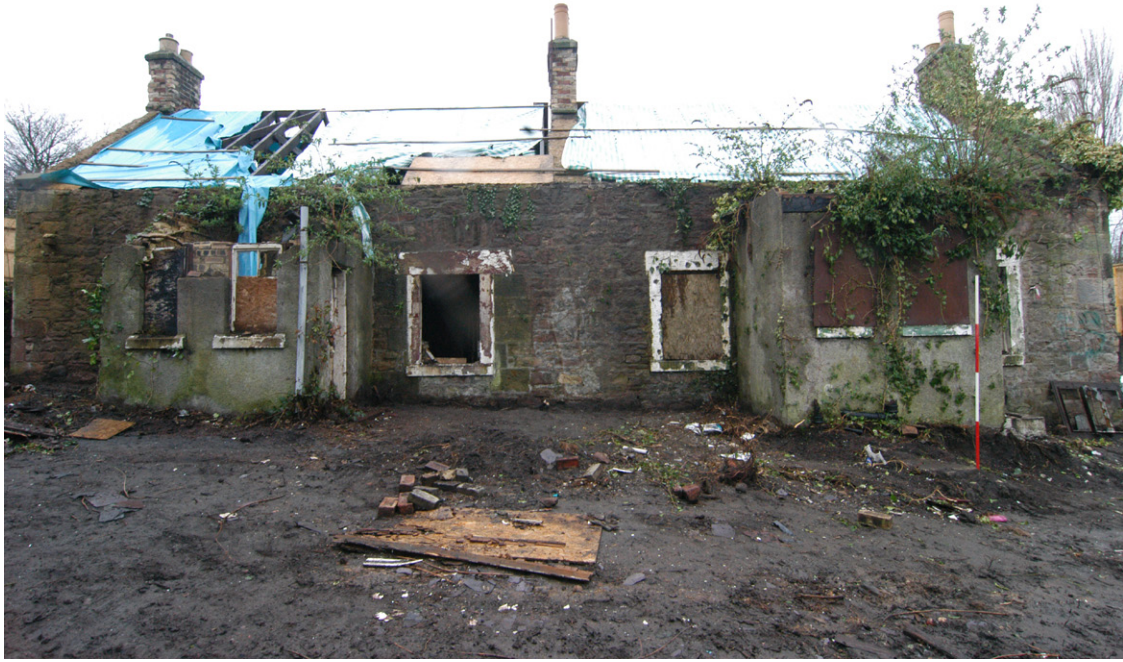
Fig. 8 Southeast-facing elevation, general view
