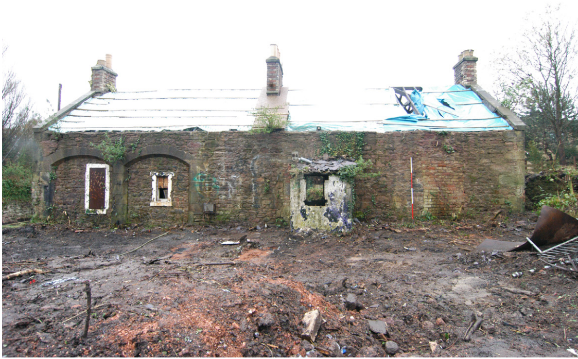
Fig. 6 Northwest-facing elevation, general view
