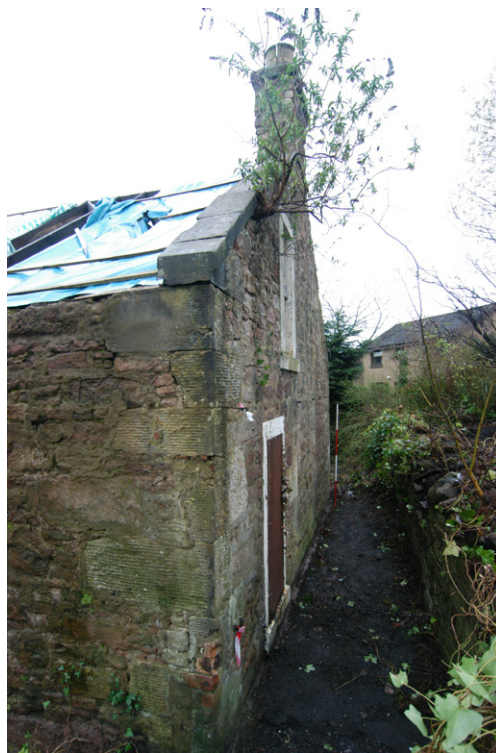
Fig. 7 Southwest-facing gable, general view
