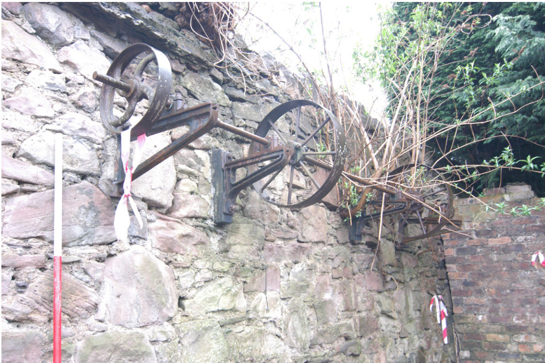
Fig. 11 Lineshaft and flywheels fixed to boundary wall
