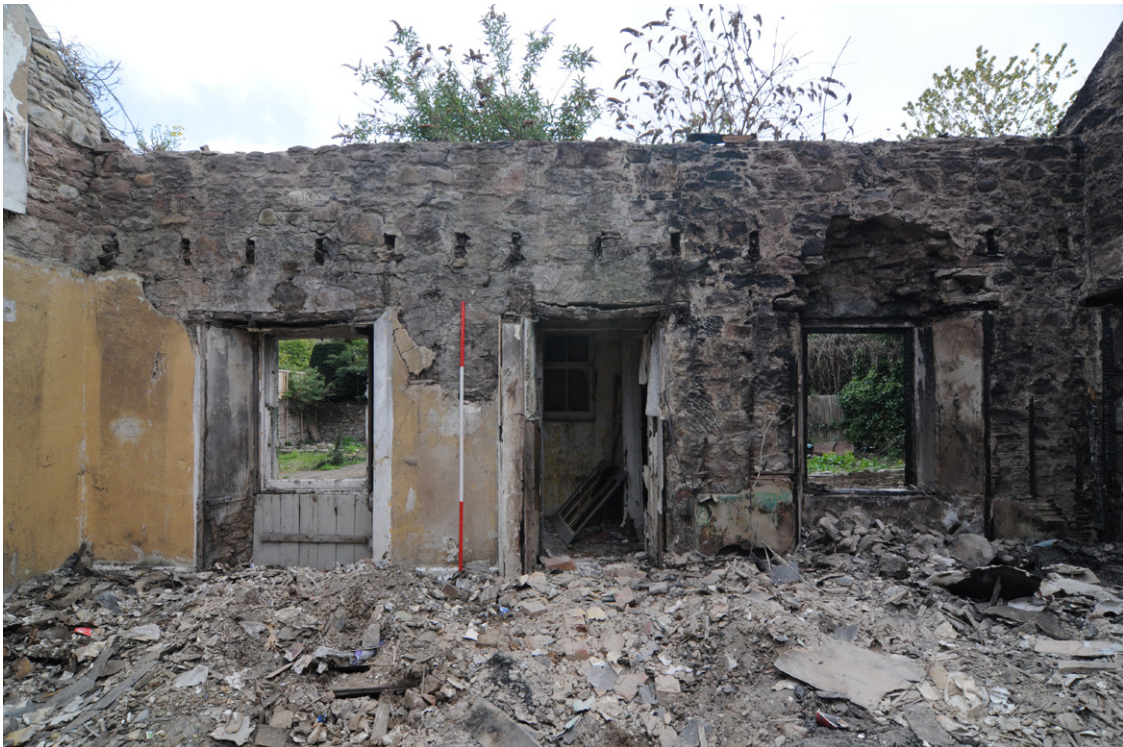
Fig. 15 Unit A, Northwest-facing elevation, post roof removal
