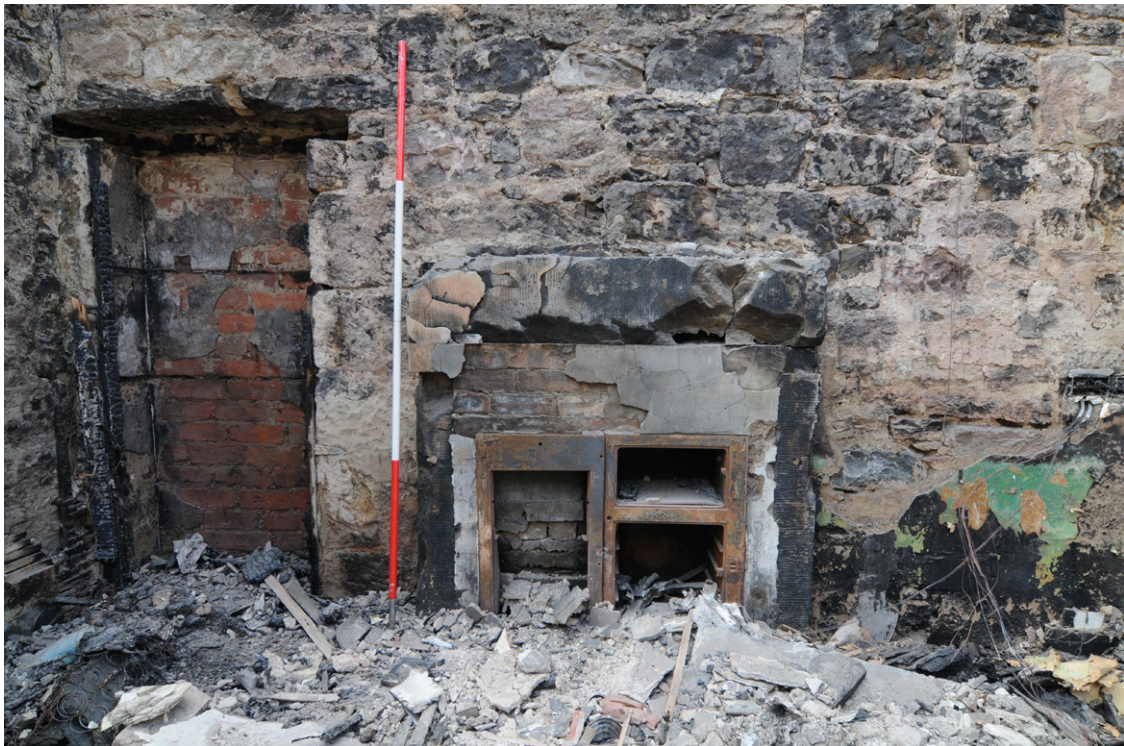
Fig. 17 Unit A, Northeast-facing partition wall showing the cast-iron range
