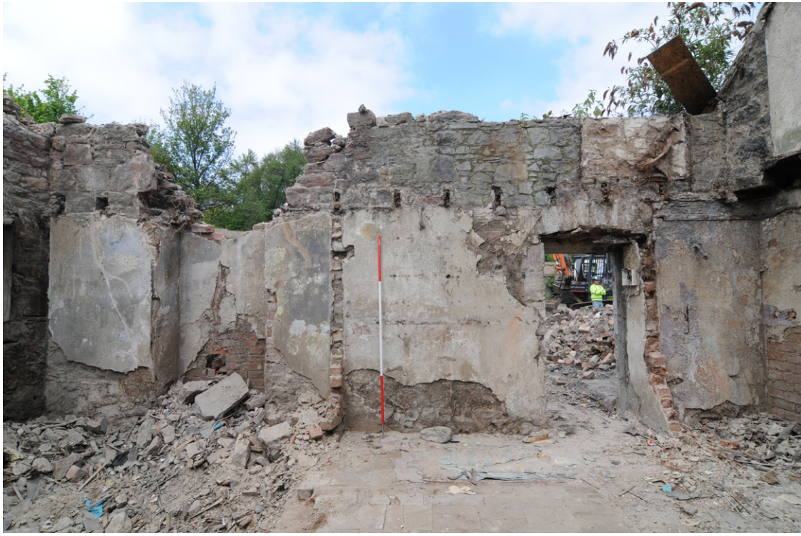
Fig. 22 Unit B, Southeast-facing elevation showing an earlier doorway and the existing doorway
