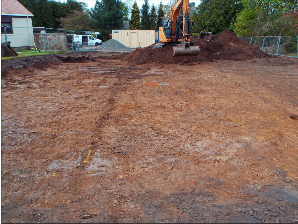
Fig. 4 - General post-excavation shot toward northern boundary of site with [003b] drain.
