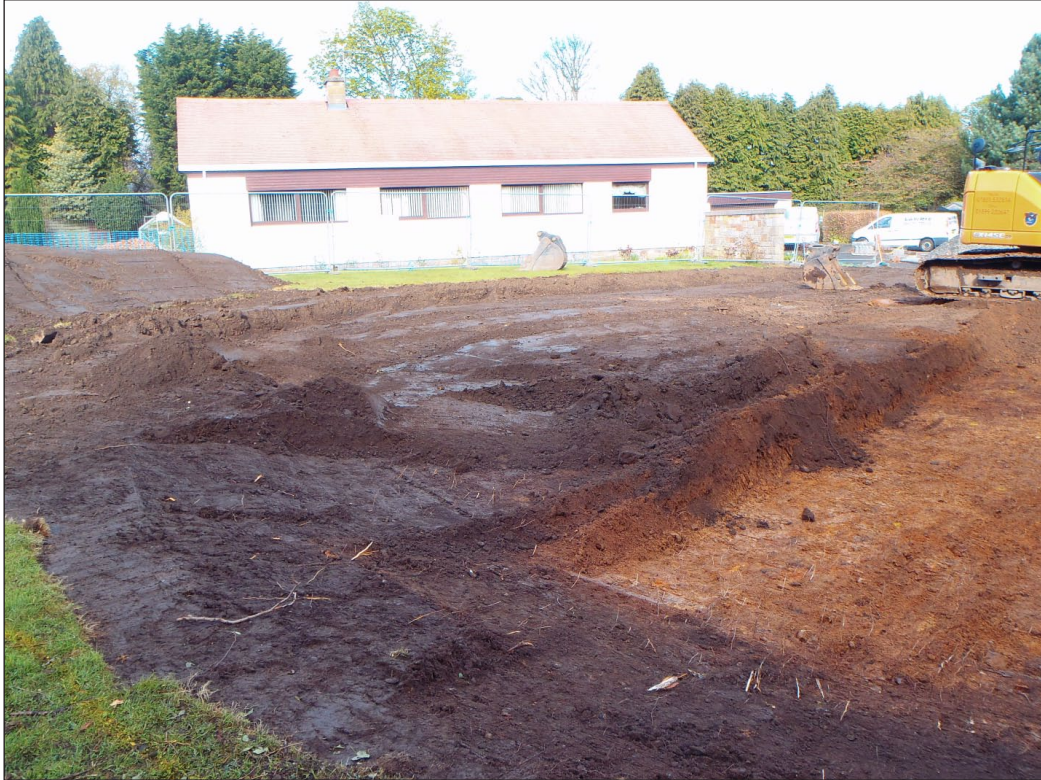
Fig. 2 - Mid-excavation shot of site toward Conifer House.
