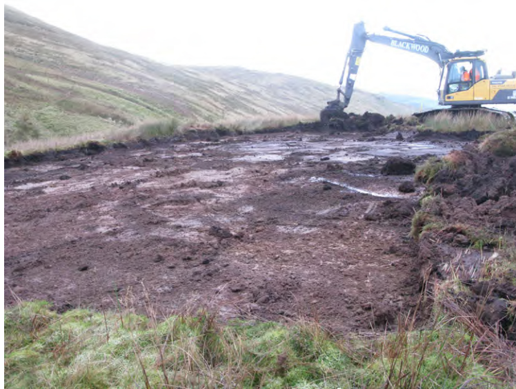
Fig. 13 - View of soil stripping for penstock along Greeto Water
