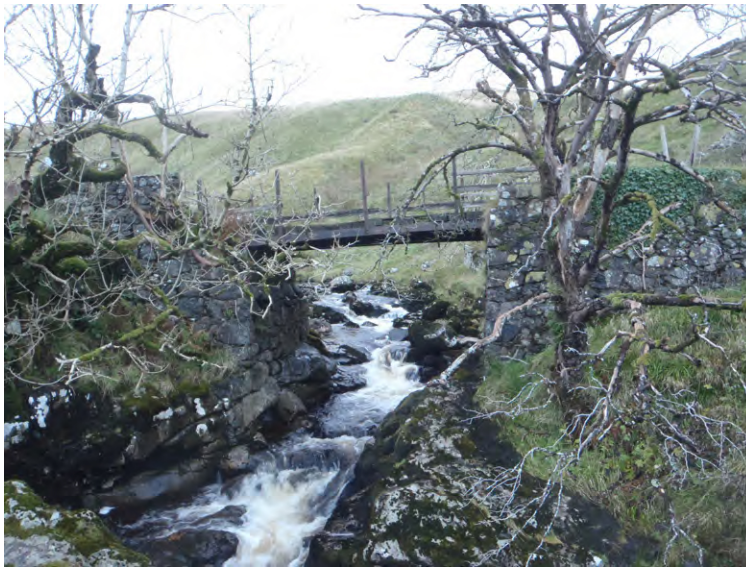
Fig. 4 - Greeto Bridge looking south-east
