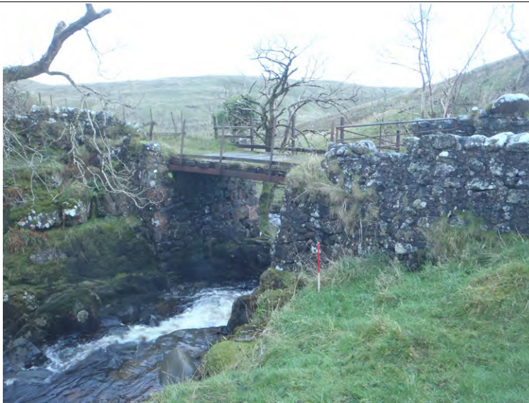
Fig. 3 - Greeto Bridge (Site 3) looking south-west
