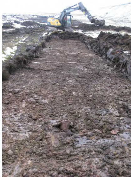
Fig. 14 - View of soil stripping for penstock east of Greeto Water
