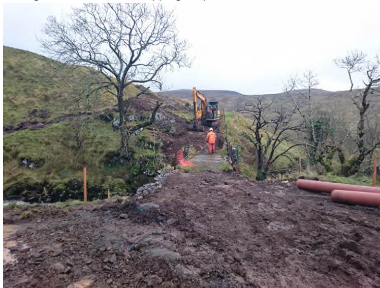
Fig. 15 - Excavation work adjacent to Greeto Bridge
