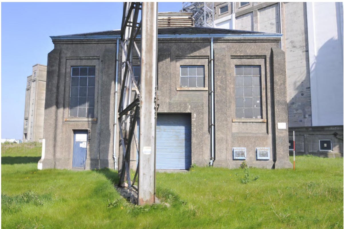
Fig. 11 Imperial Dock East Sub Station - South-east-facing elevation
