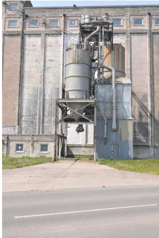
Fig. 14 East-facing elevation of the Dust Extractor Silos
