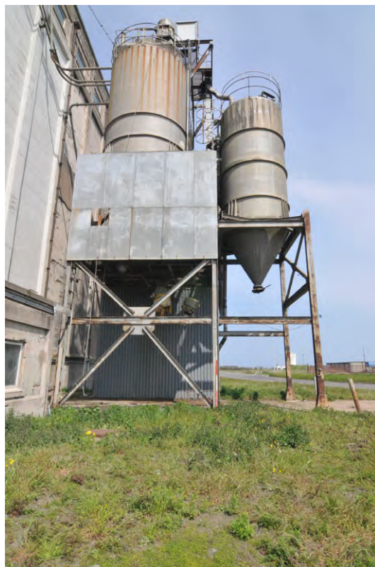
Fig. 15 South-facing elevation of the Dust Extractor Silos
