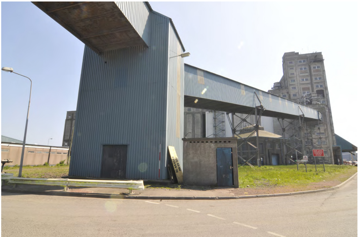
Fig. 7 Grain Conveyor crossover from incline to horizontal
