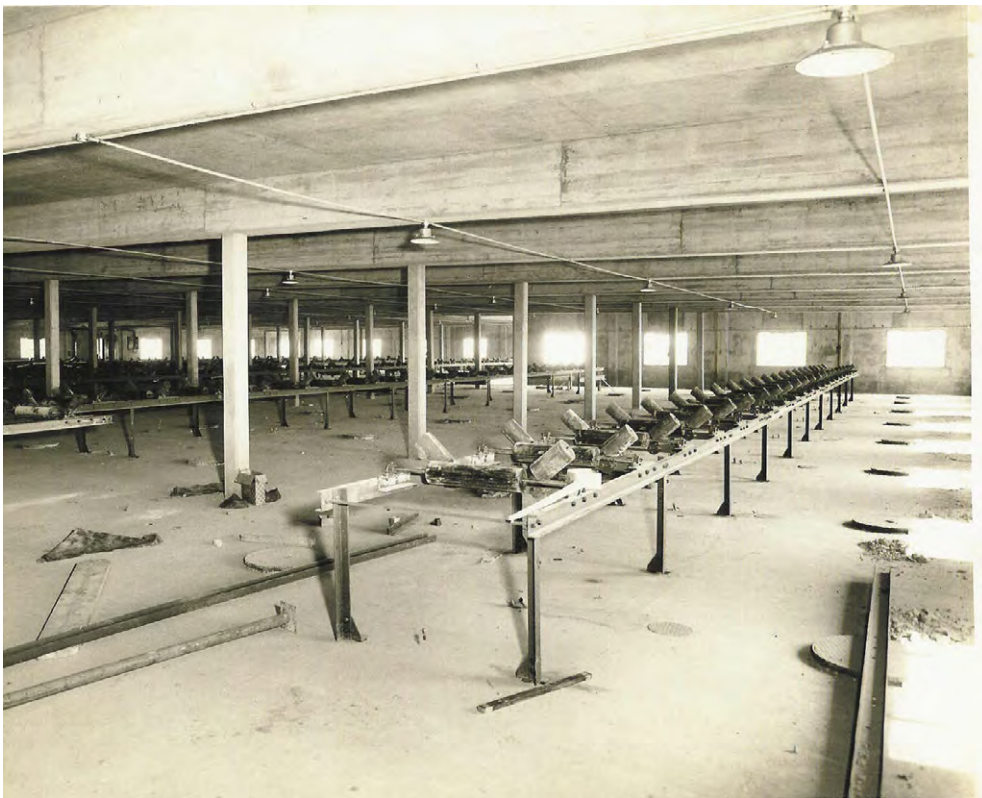
Fig. 23 Fitting out the Distribution floor
