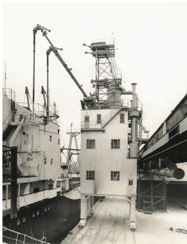
Fig. 27 Mobile grain elevator alongside Imperial Dock
