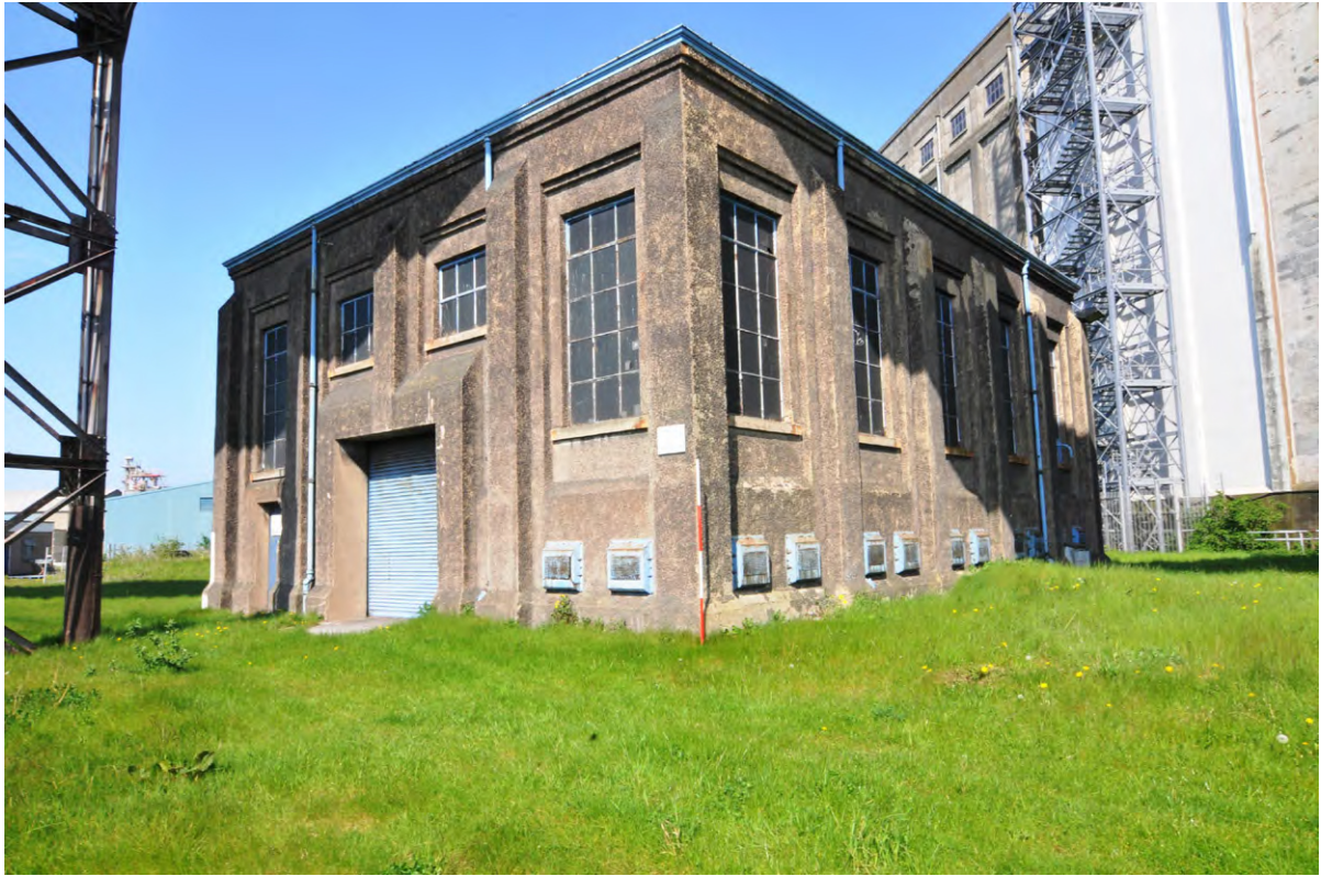
Fig. 10 Imperial Dock East Sub Station - South-west-facing elevation
