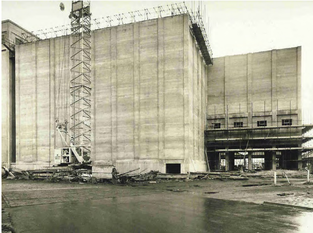
Fig. 26 Phase 3 block nearing completion
