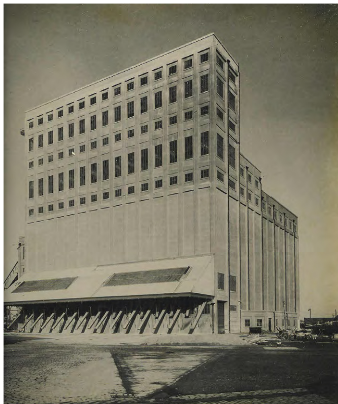
Fig. 19 The 1934 warehouse after completion
