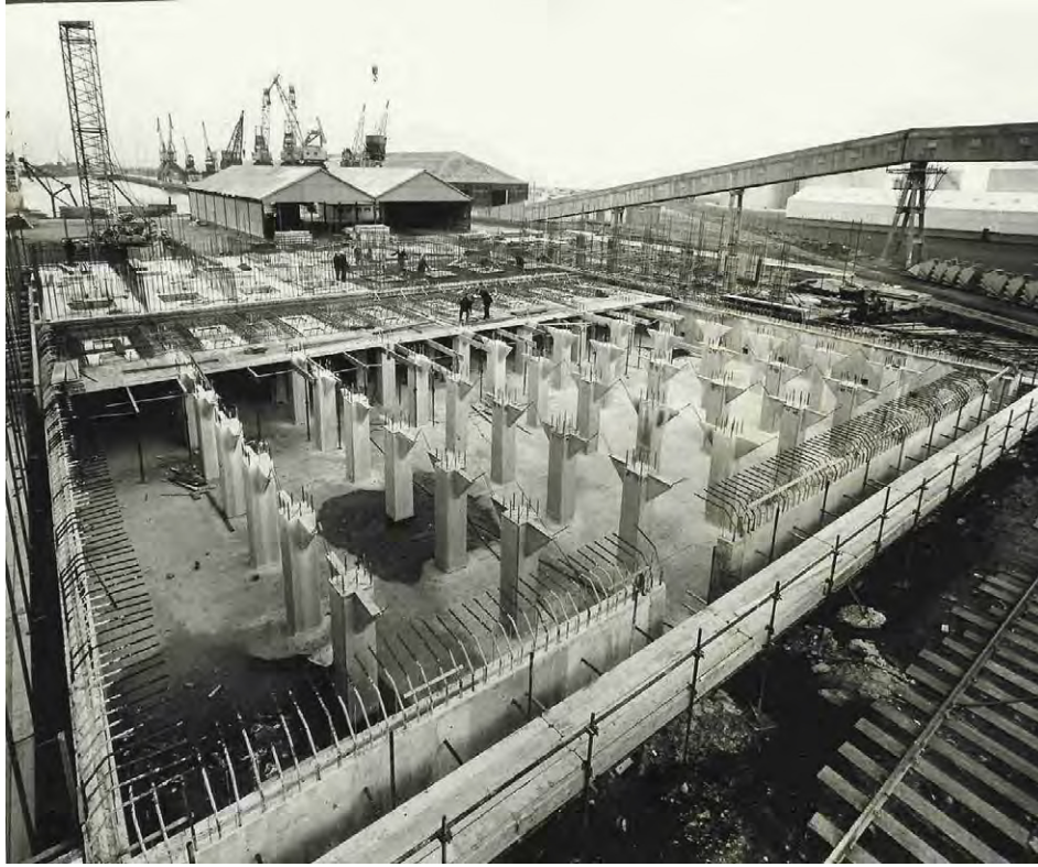
Fig. 24 General view of Phase 3 collecting floor under construction
