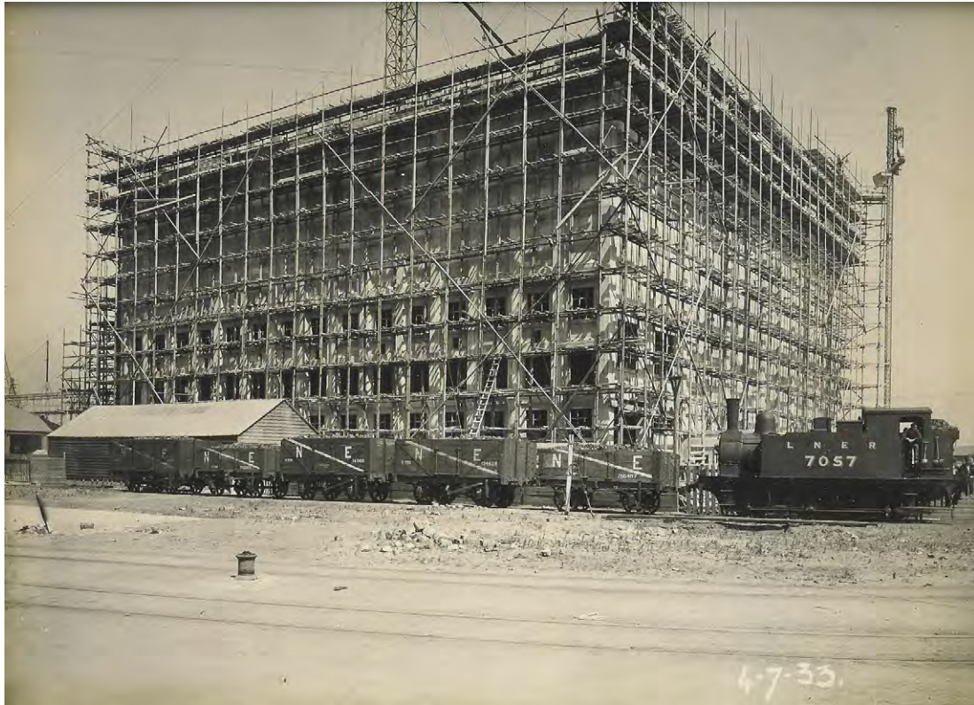
Fig. 18 South and east-facing elevations under construction
