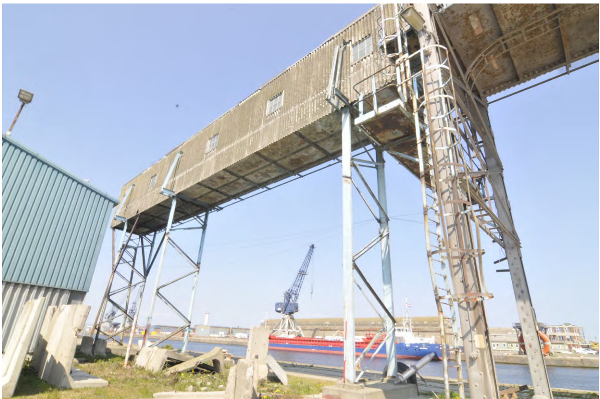
Fig. 9 West terminus of the grain conveyor and an earlier surviving section dating to 1937
