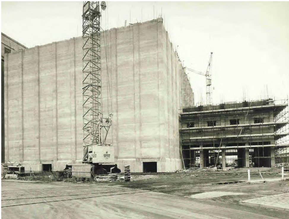
Fig. 25 Construction of the loading bays completed on the east-facing elevation
