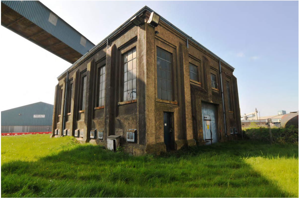
Fig. 12 Imperial Dock East Sub Station - North-west-facing elevation
