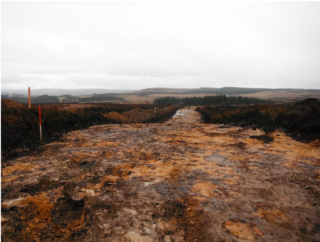
Fig. 12 Post excavation shot of haul road along Spur 6
