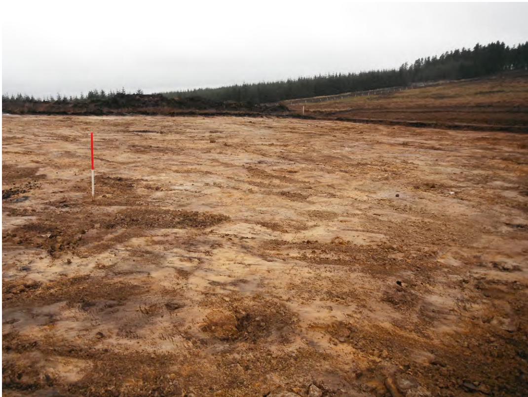
Fig. 14 Post excavation shot of crane pad at end of Spur 11
