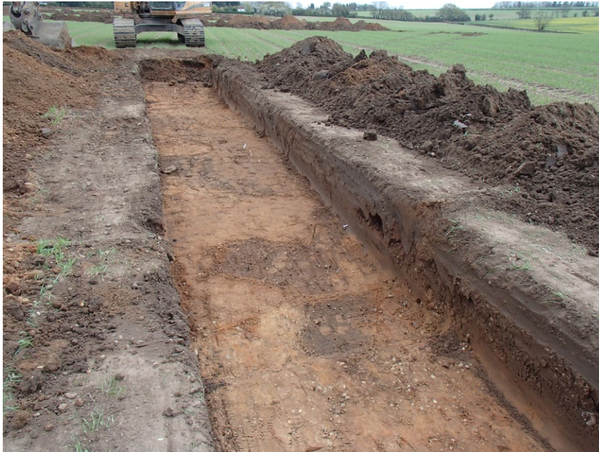
Fig. 35 - Trench 10, from the NW
