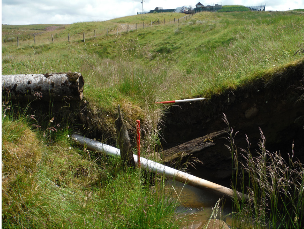
Fig. 10 - Aqueduct carrying inlet channel
