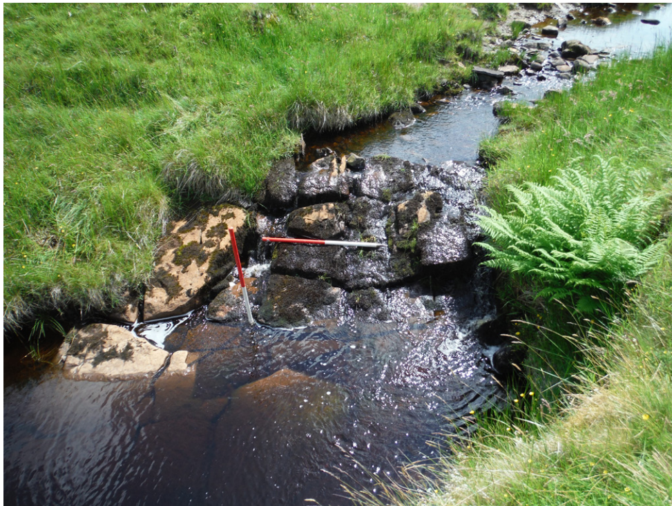
Fig. 9 - Weir in Auldhouse Burn
