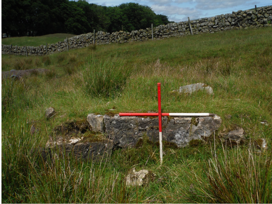
Fig. 6 - Stone facing on dam
