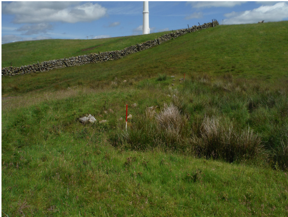
Fig. 5 - General shot of dam
