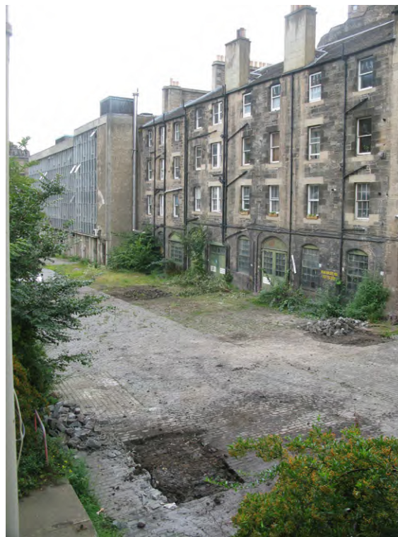
Fig. 10: General shot of site following backfilling
