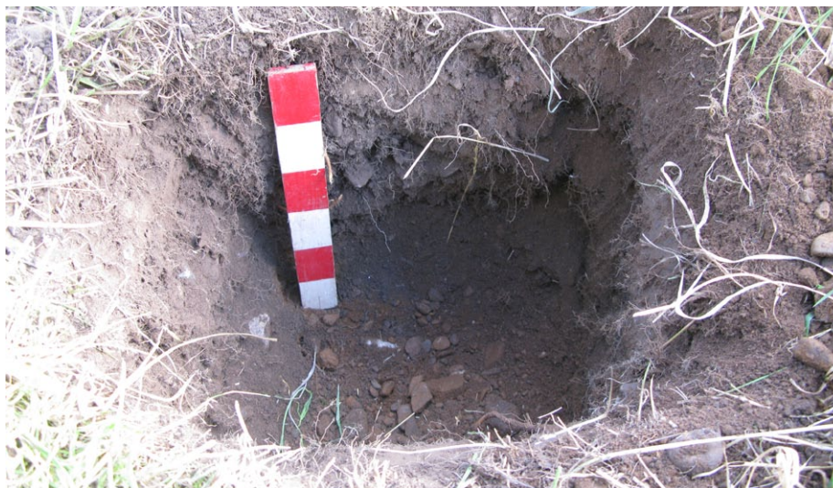
Fig. 4 - Starter pit for borehole 3.1b
