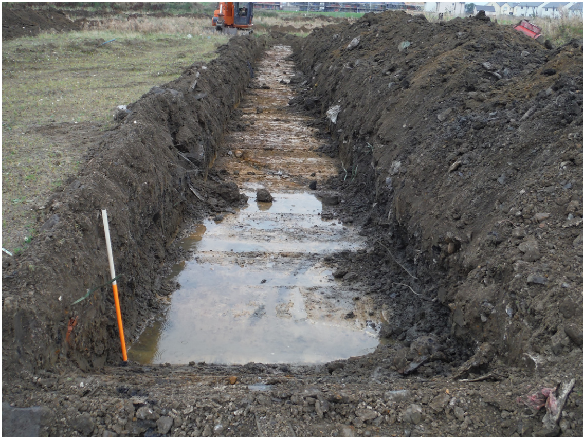
Fig. 9: Trench 54 from West
