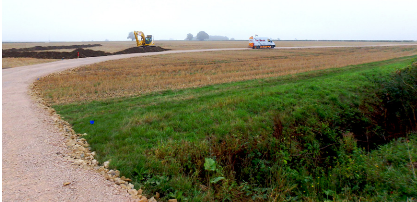
Fig. 5 - Floated access road built past central turbine, taken from W
