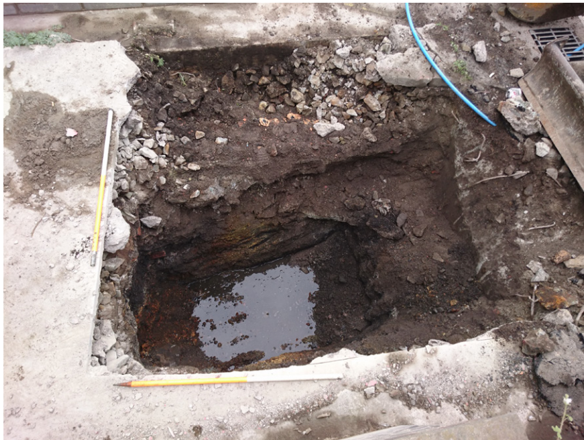
Fig. 3 - Plan view of trench (from NE)
