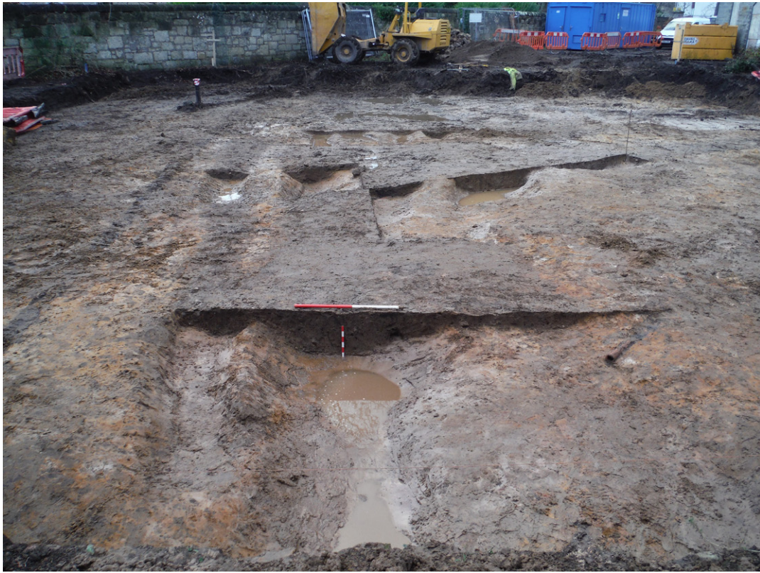
Fig. 5 General view of the ditches to the south-west of St Leonards Lodge from SE
