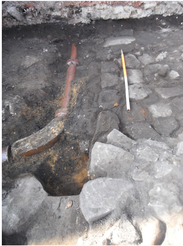
Fig. 20 Culvert 342 cut by modern pipe trench 330
